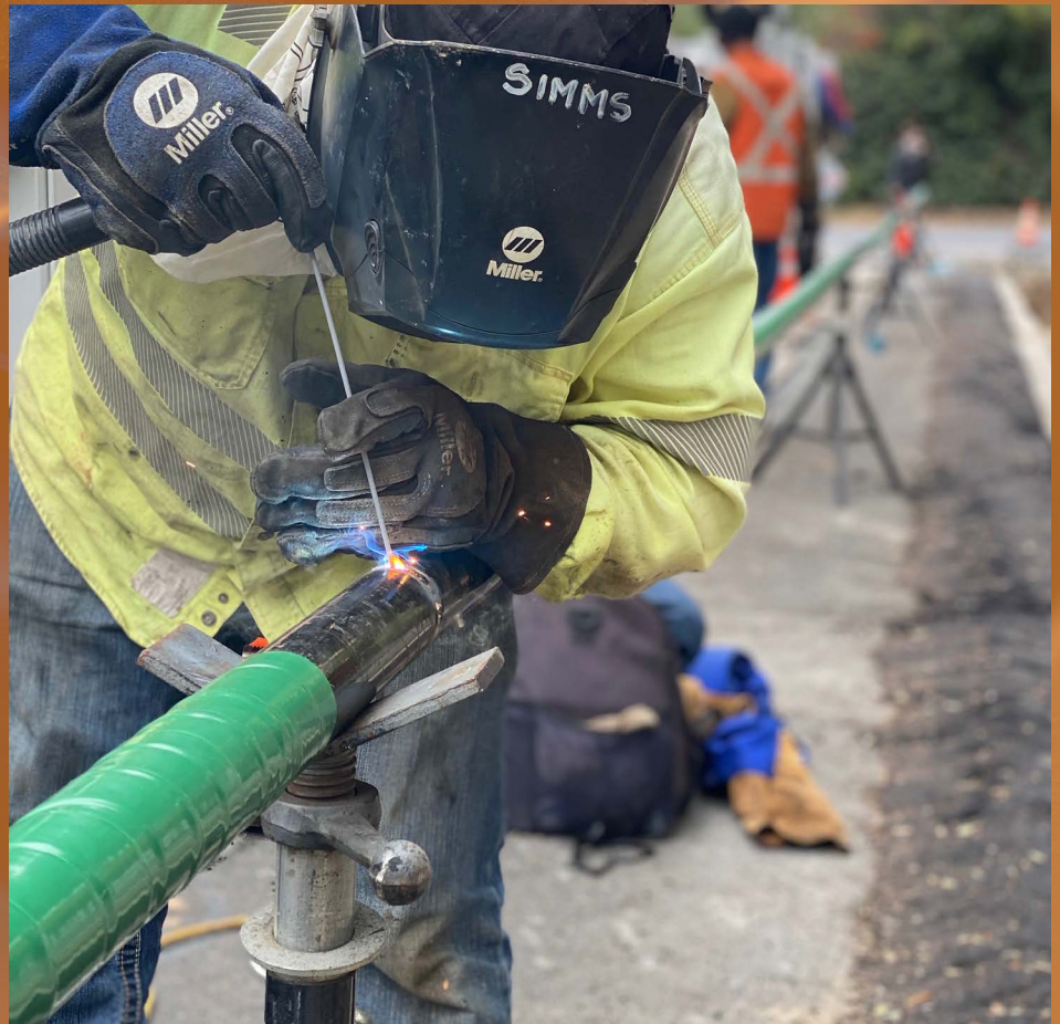
A CPAU employee replacing a natural gas main.
