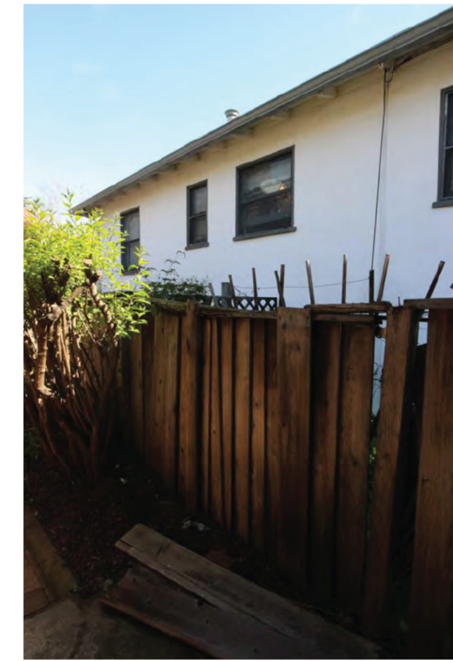
4 VIEW OF 991 CHANNING FROM EAST SIDE YARD
