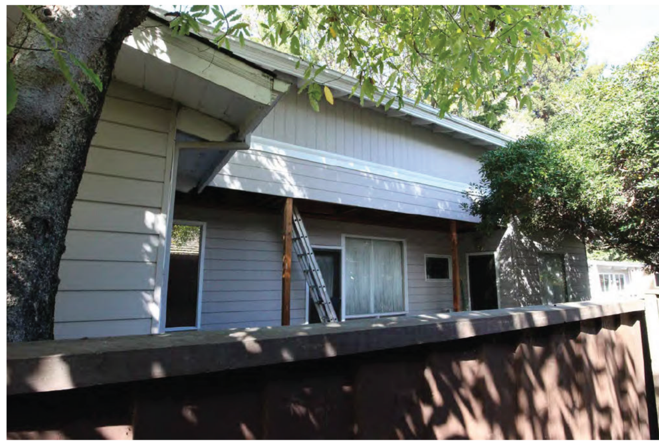
2 VIEW OF 975 CHANNING FROM WEST SIDE YARD
