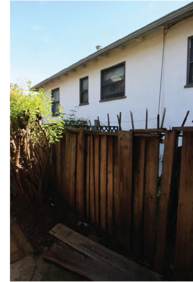
4 VIEW OF 991 CHANNING FROM EAST SIDE YARD
