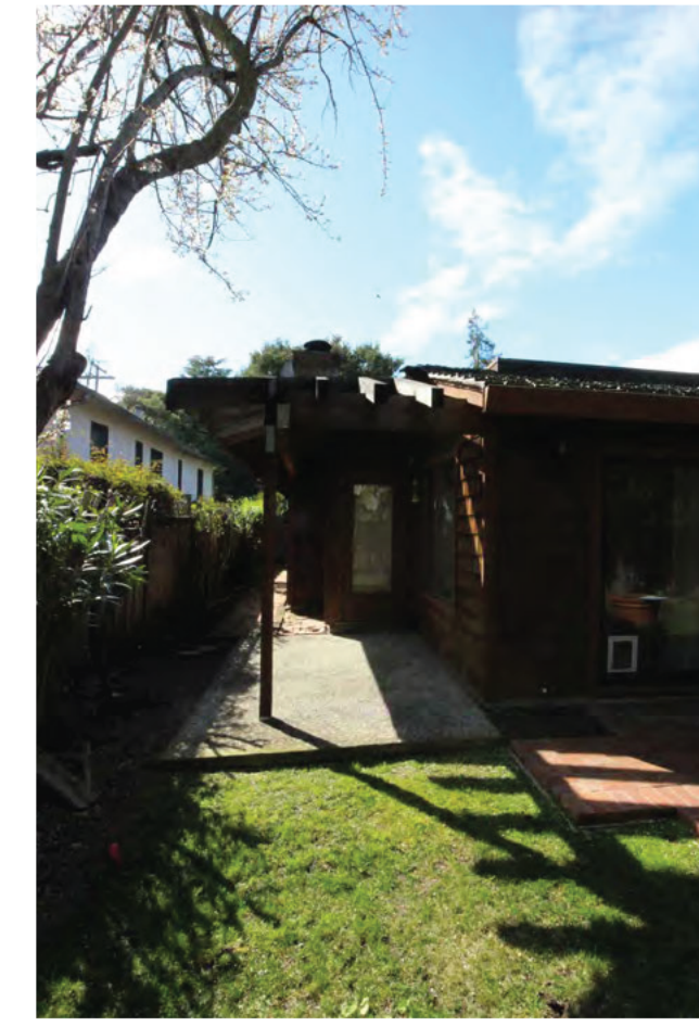
7 (E) PATIO AT AT NORTHEAST CORNER OF BUILDING
