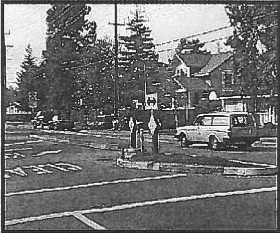
Median Barrier Park Blvd/Meadow, Palo Alto
