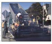
Pavement repair: White paint markings on the street show areas of Temporary striping is installed (if previously existing) prior to reopenpavement failure. These areas are excavated, re-compacted and filled ing the street to traffic. Permanent striping is installed 7 to 10 days after overlay. These operations should minimally impact traffic and parking.
