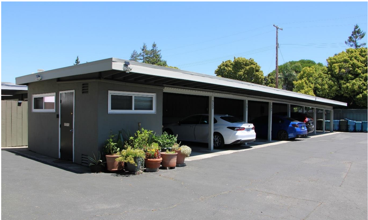
Figure 6 739 Sutter Avenue Carport, View Northeast
