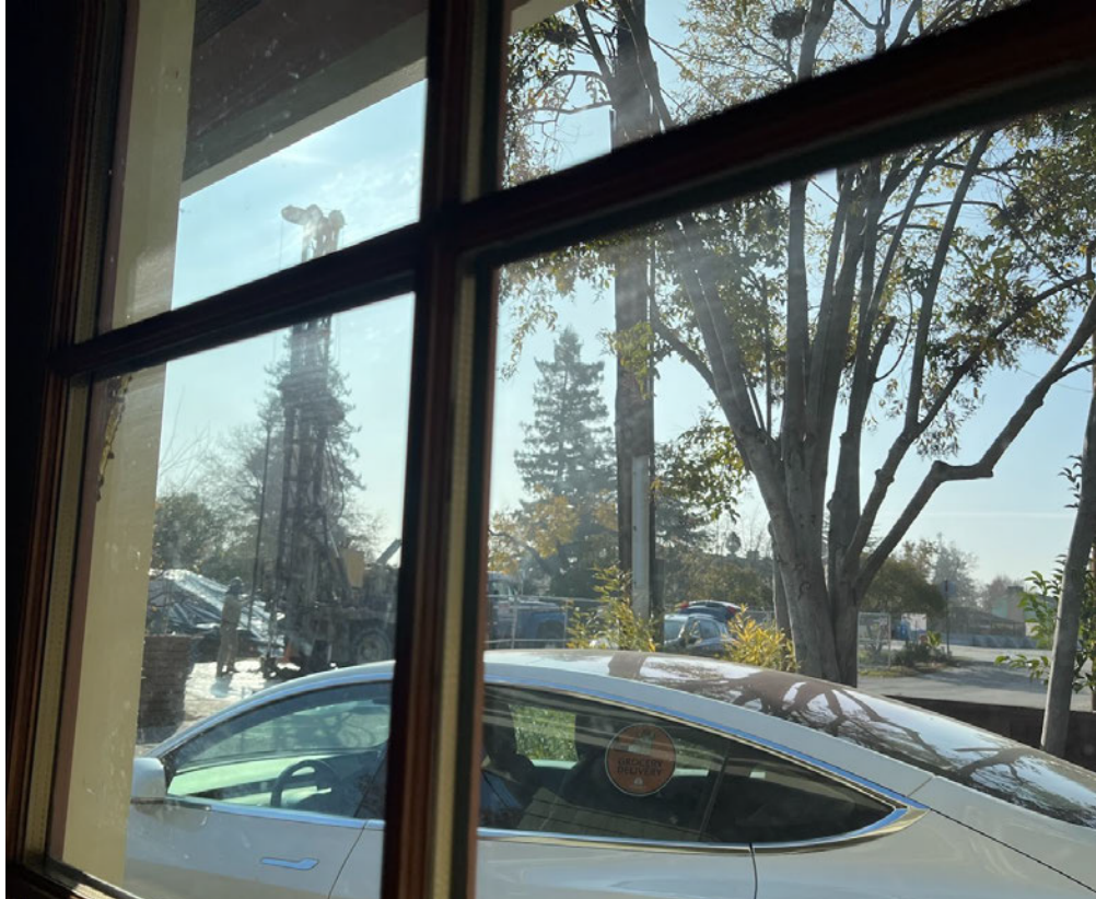
(Photo below shows the drilling rig; taken through a neighbor's window on December 20, 2022)
