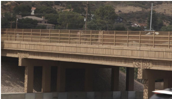
Award Winning Hand Carved Agoura Hills Bridge Cheseboro Crossing offramp - 101 Freeway
