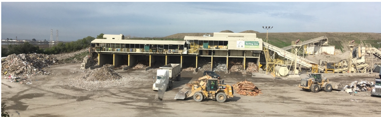
Zanker Materials Processing Facility
