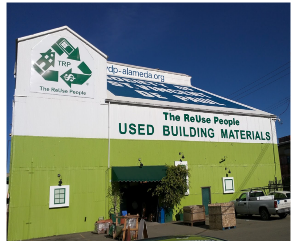
Since 2016, 25% of the City’s whole house demolition projects have been deconstructed instead of demolished.
