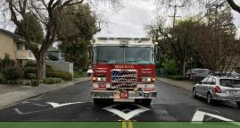
Slotted Speedhumps: speed tables that include wheel cutouts to allow large vehicles to pass unaffected, while reducing passenger car speeds.
