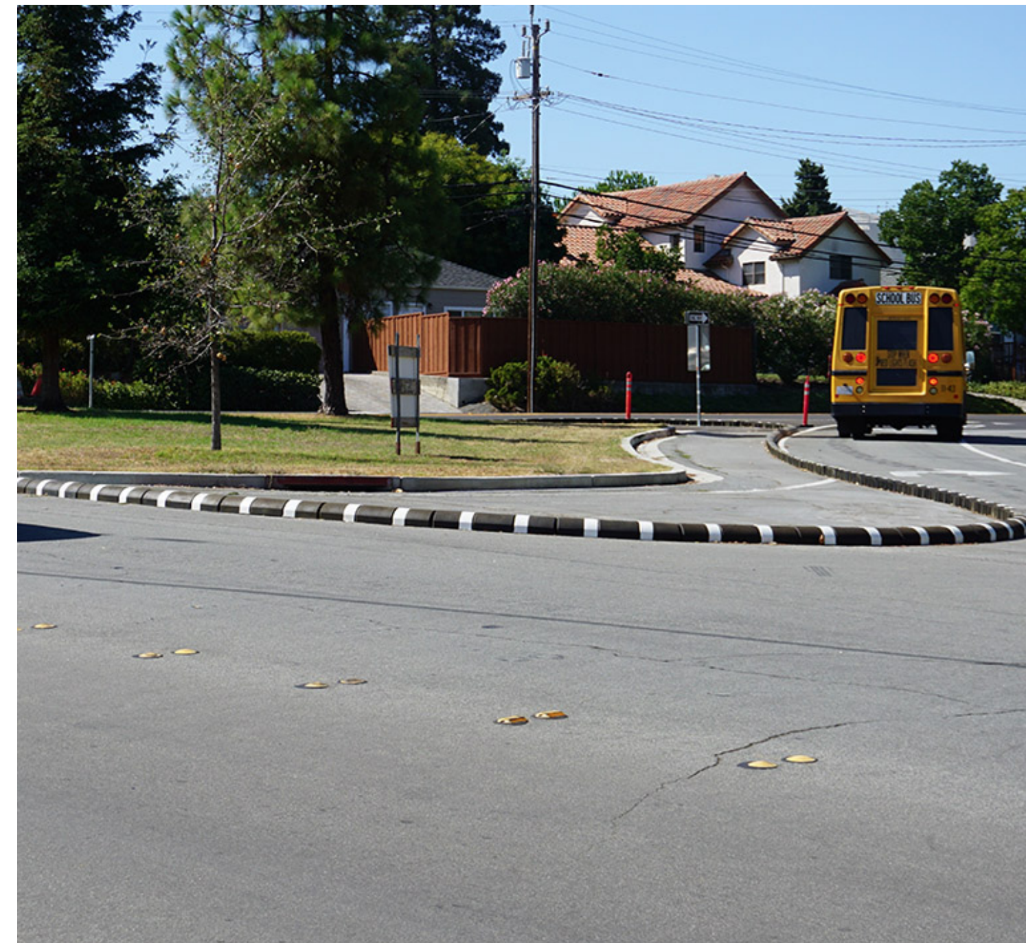
Rubber curb used for intersection realignment
