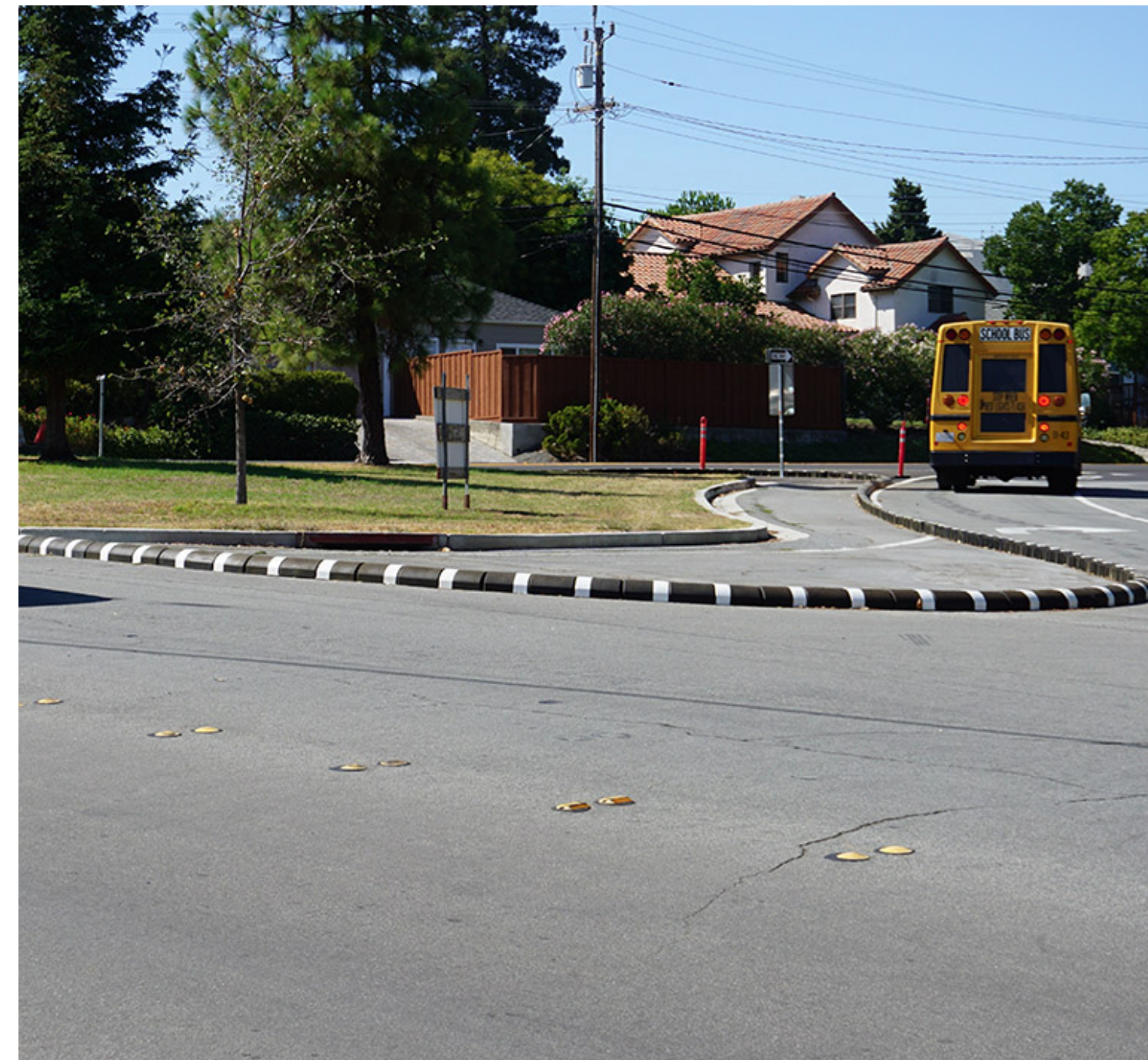
Rubber curb used for intersection realignment
