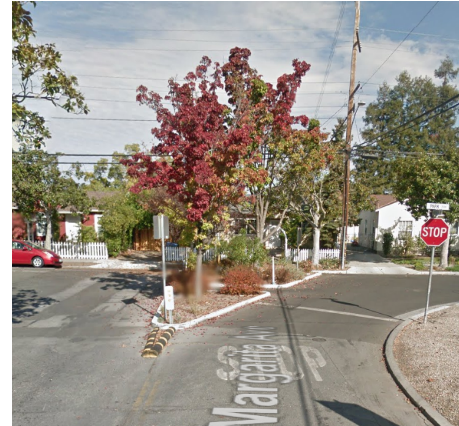
Permanent right-turn diverter island with landscaping (Margarita Avenue at Park Boulevard)
