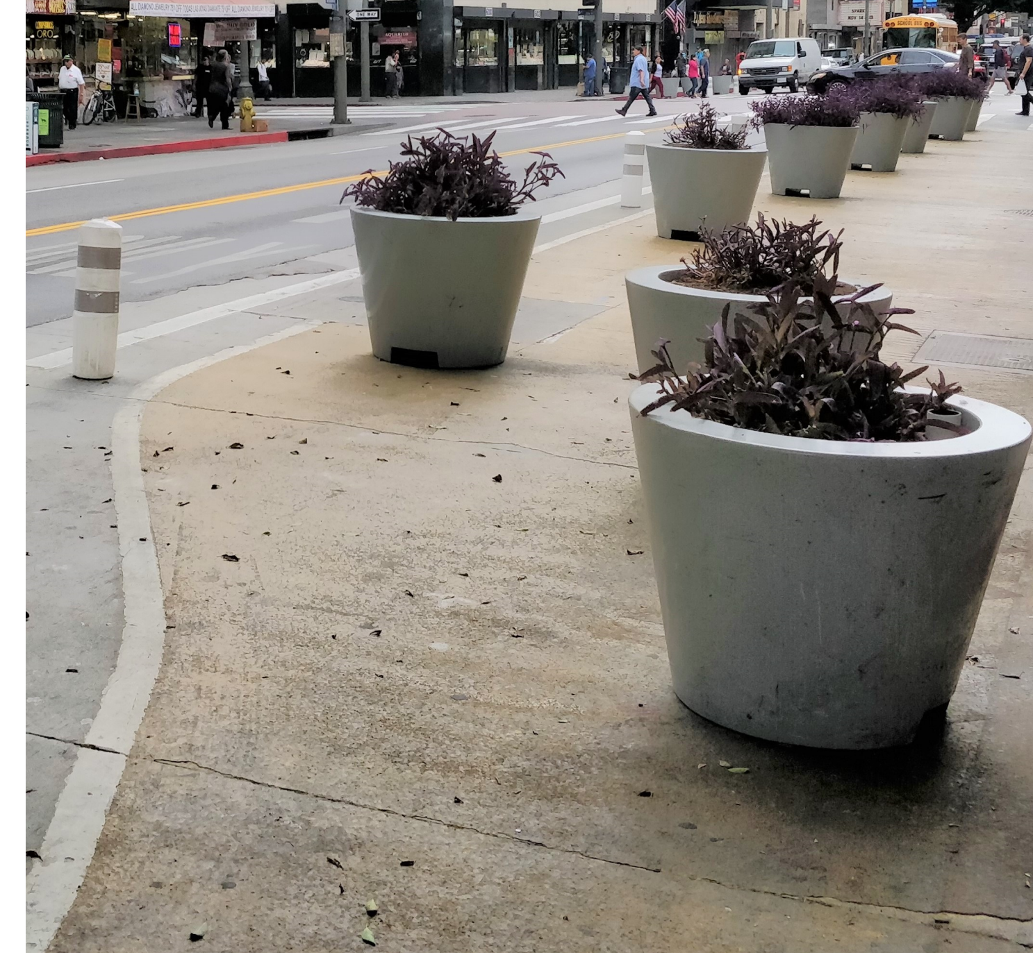
Planters, flexible bollards, and paint used for roadway realignment
