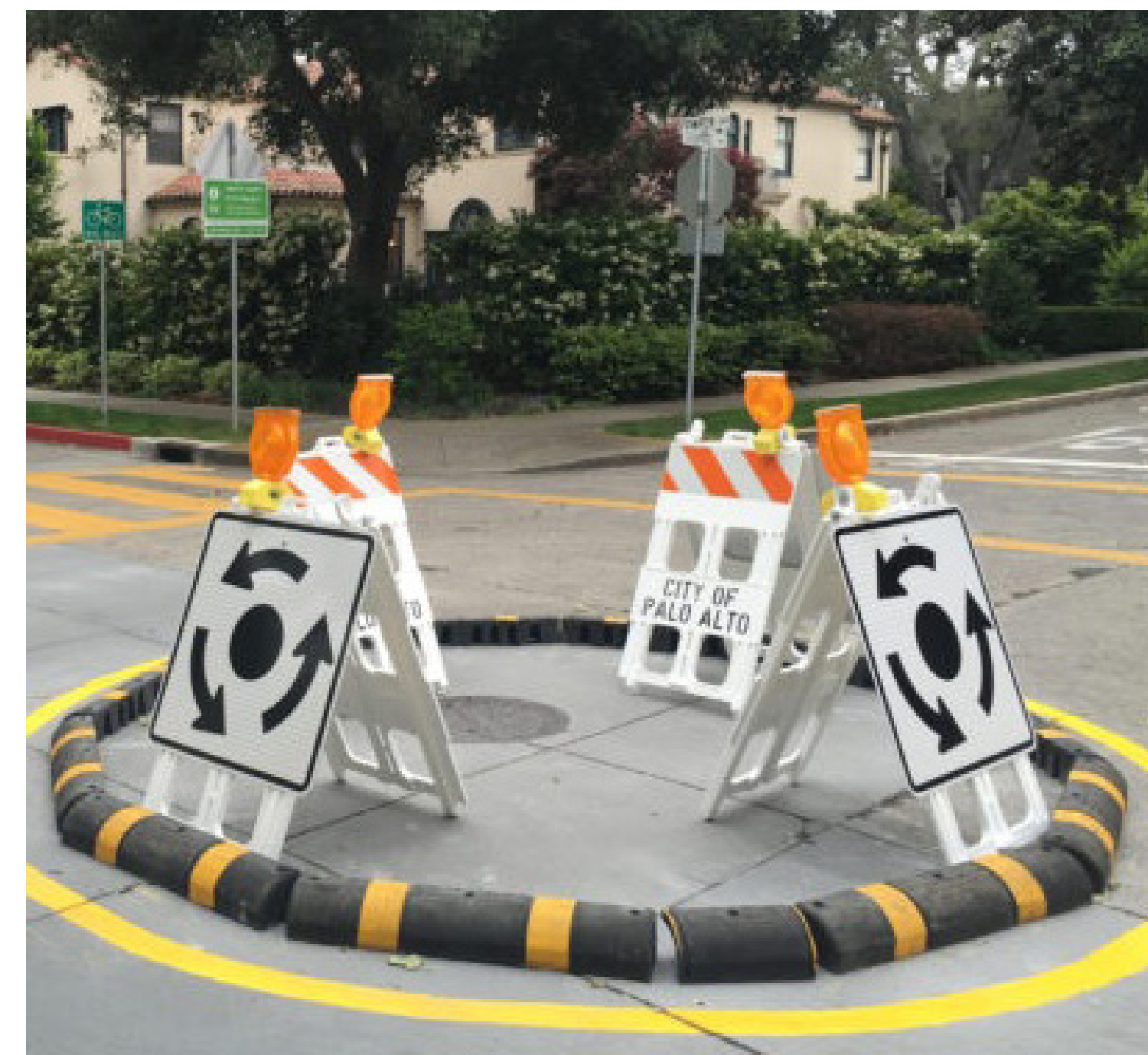
Temporary traffic circle using rubber curbs and signs (Cowper Street & Coleridge Avenue)
