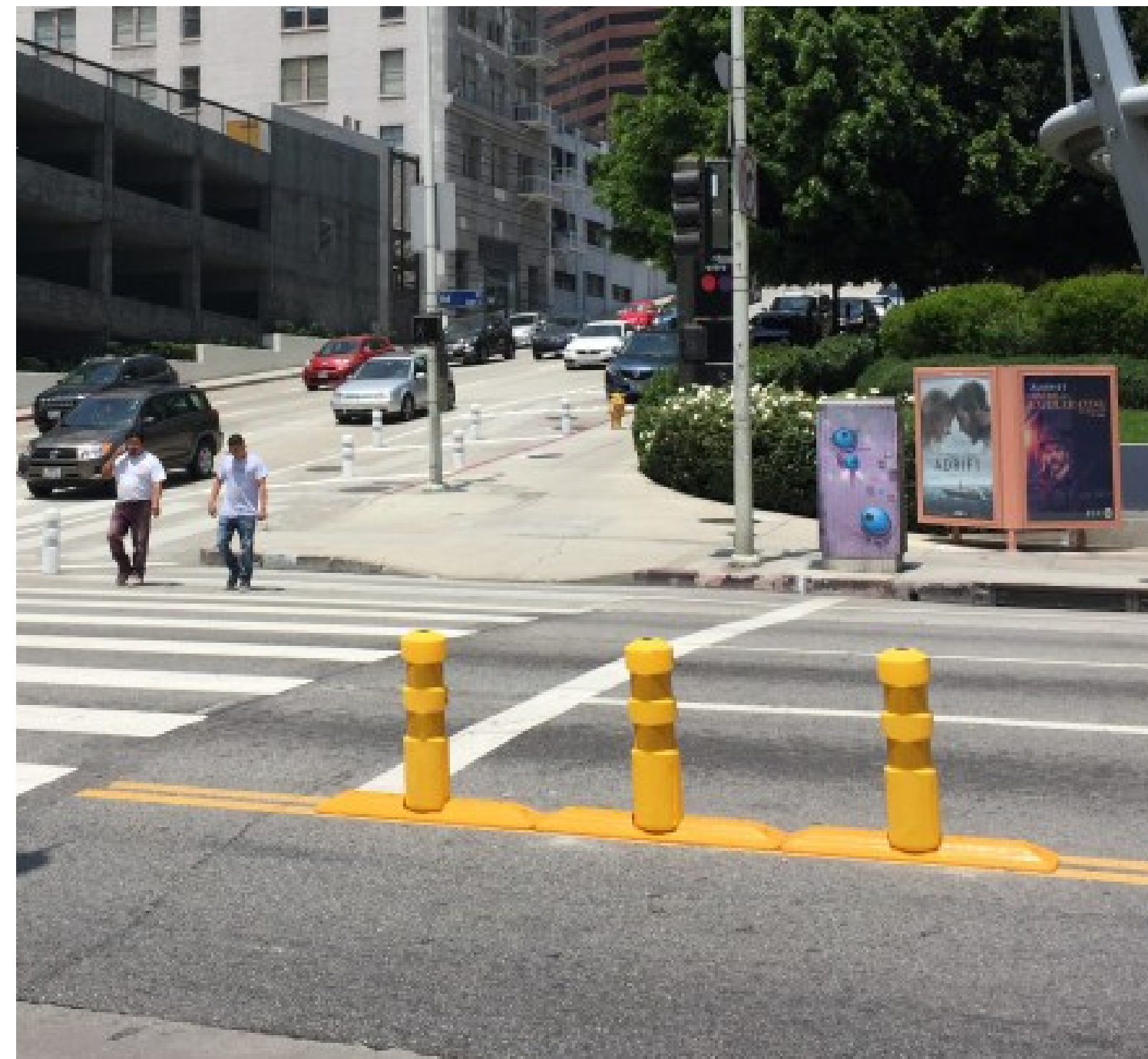
Flexible posts to channelize traffic
