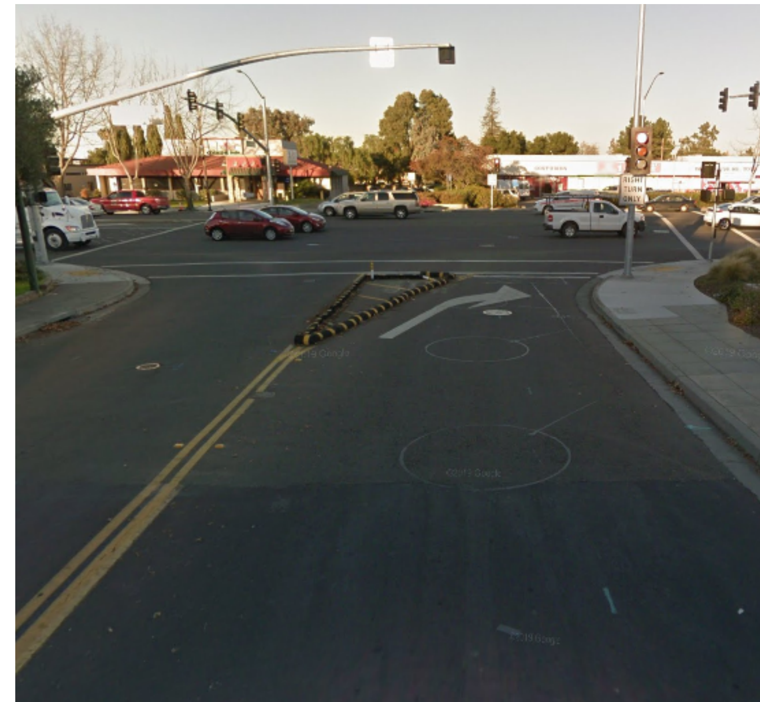
Rubber curb diverter to prevent left turns (Clark Avenue at El Camino Real, Mountain View)
