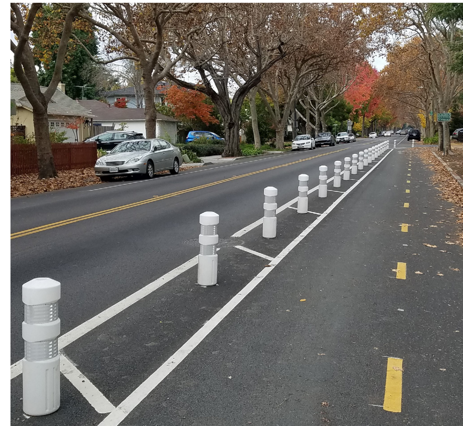
Flexible posts to separate parallel bicycles and vehicles (Middlefield Road adjacent to Greene Middle School)
