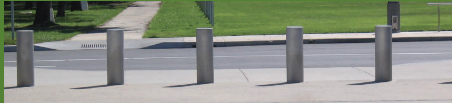
Contemporary removable bollards for Cal Ave
