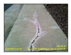
Cracking (Shattered Slab) – Cracks that cut through the concrete slab, dividing the slab into multiple pieces. These cracks are commonly caused by a combination of repeated heavy loading (in the case of sidewalks adjacent to a driveway), or thermal gradient curling, shrinkage/swelling of the underlying subgrade or tree root uplift.
