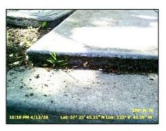
Faulting – The difference in elevation across adjacent concrete slabs or across cracks that have divided the slab.
