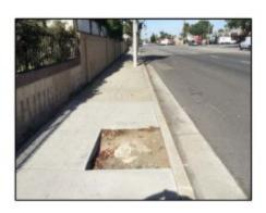
Holes – Gaps in the sidewalk that extends vertically through the concrete slab. Holes may obstruct traffic as they limit the useable area of the sidewalk.
