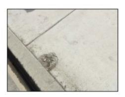
Spalling – The breakdown of the concrete in the sidewalk or curb and gutter within two feet of its edge. A spall usually does not cut through a concrete slab vertically like a crack, but is angled toward the edge.
