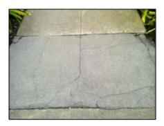
Patching – Areas where the original sidewalk has been removed and replaced with a new material, or where the sidewalk has been overlaid with a new material such as concrete or asphalt concrete.
