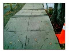
Vaulting – The difference in elevation between two adjacent concrete slabs, where they are both raised to a high point.
