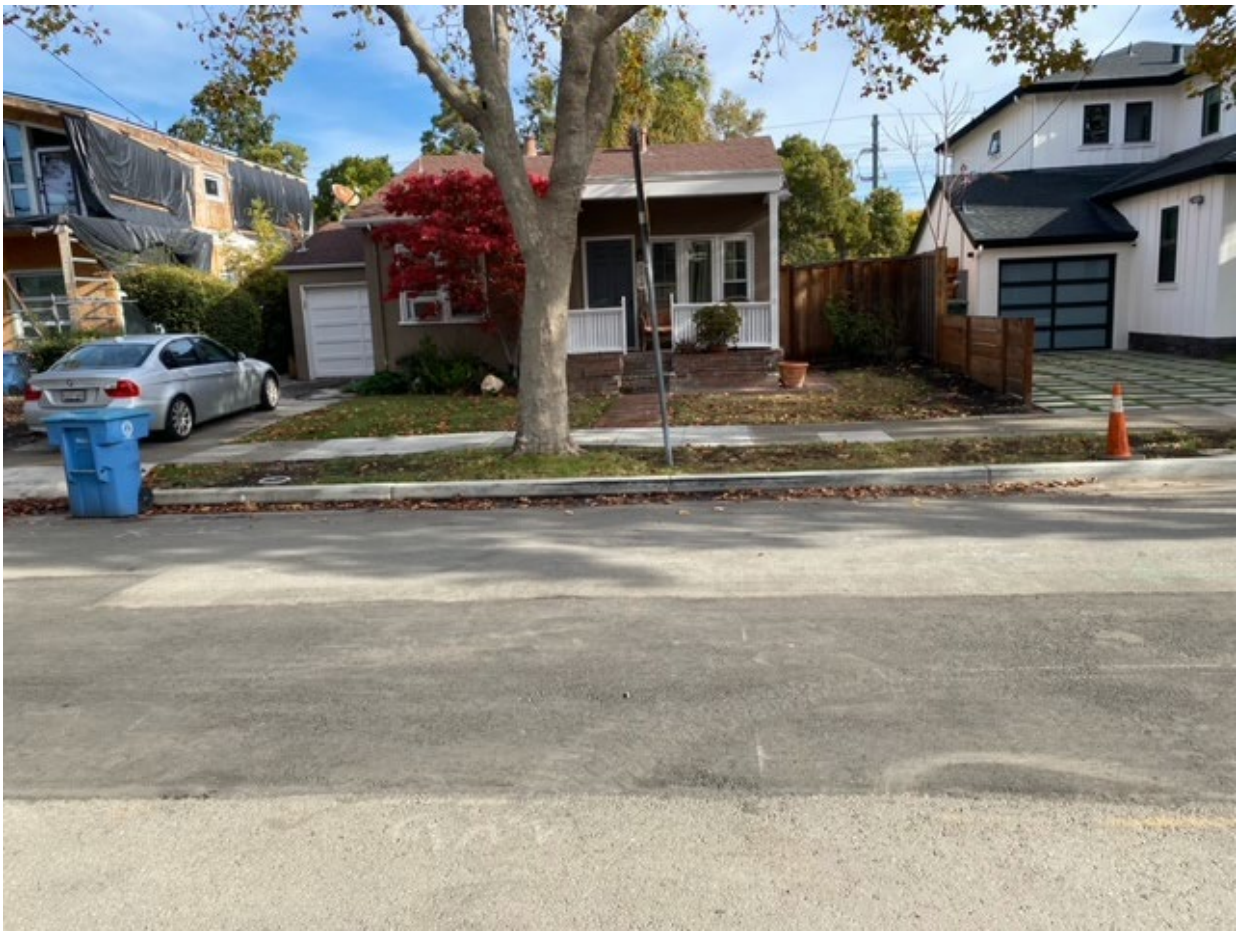
The quality of that patch is *significantly* better than the asphalt immediately adjacent at 3605 Park Blvd:
