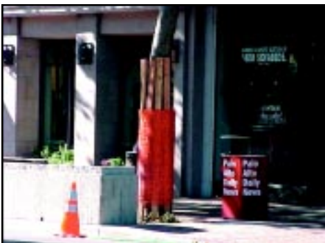
IMAGE 2.15-4 Trunk Wrap Protection
