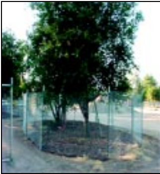
IMAGE 2.15-1 Tree Protection Fence at the Dripline
