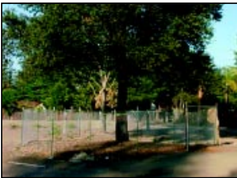
IMAGE 2.15-2 Tree Protection Fence at the Dripline
