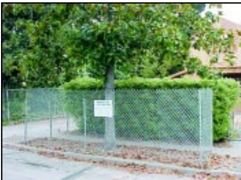
IMAGE 2.15-3 Tree Protection within a Planter Strip
