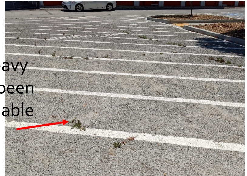
San Fransiquito Pump Station
