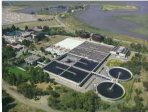
The City of Palo Alto Regional Water Quality Control Plant treats 17 million gallons of wastewater each day from Palo Alto and its five partner communities.
