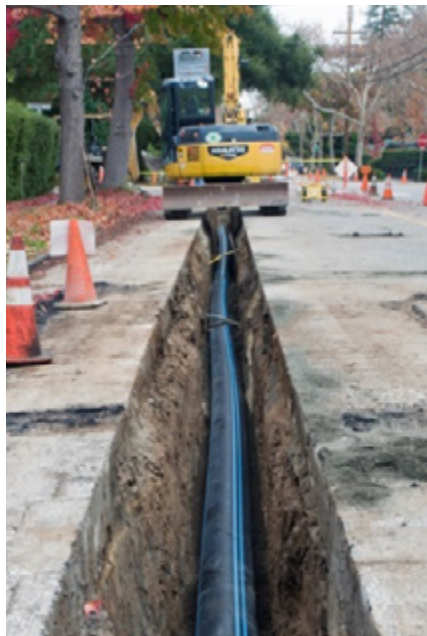
Palo Alto's 235 miles of water main lines are resilient to flooding, but high shallow groundwater could cause uplift forces that are problematic for pipes.
