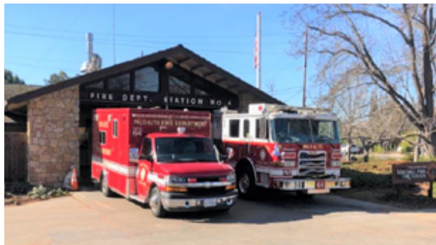
Regular foundation and structural inspections should begin at Fire Station #4 with 12 inches of sea level rise to avoid structural risks from rising shallow groundwater.
