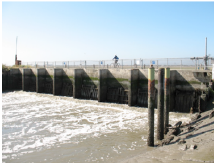
The Palo Alto Flood Basin tide gate regulates water between San Francisco Bay and a flood detention basin to protect urban areas from flooding.
