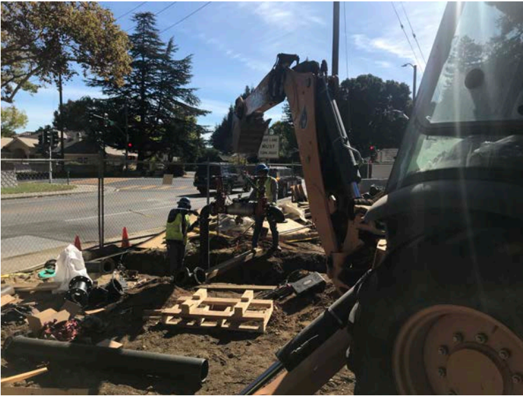
New backflow assemblies being installed.
