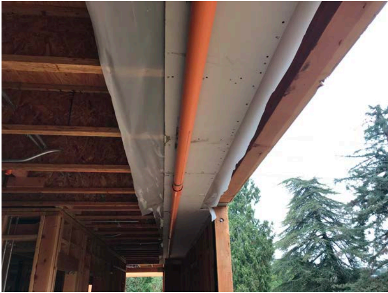
Sprinkler line install on second floor.
