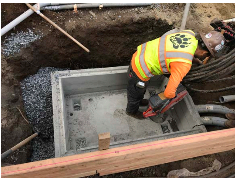
New Utilities Vault being Installed.
