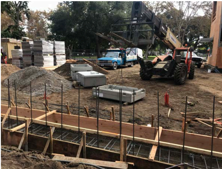
Forms and rebar for CMU fence foundation.
