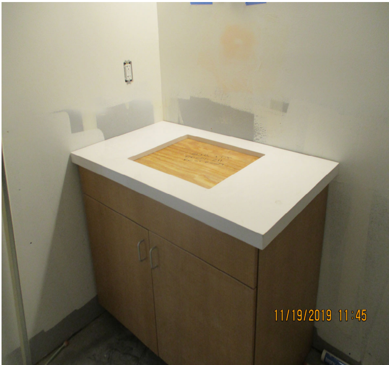
Casework and countertop installation.
