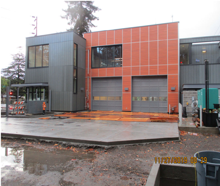
North elevation with completed concrete drive lane in foreground.
