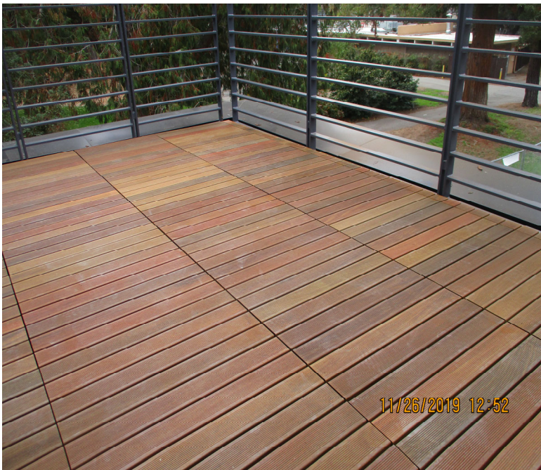
Completion of balcony decking.
