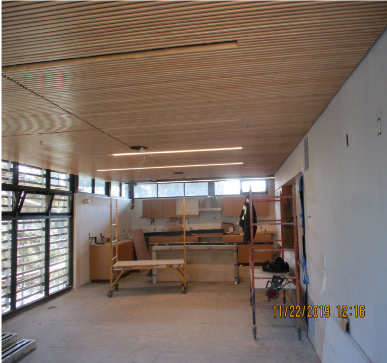
Installation of wood ceiling.
