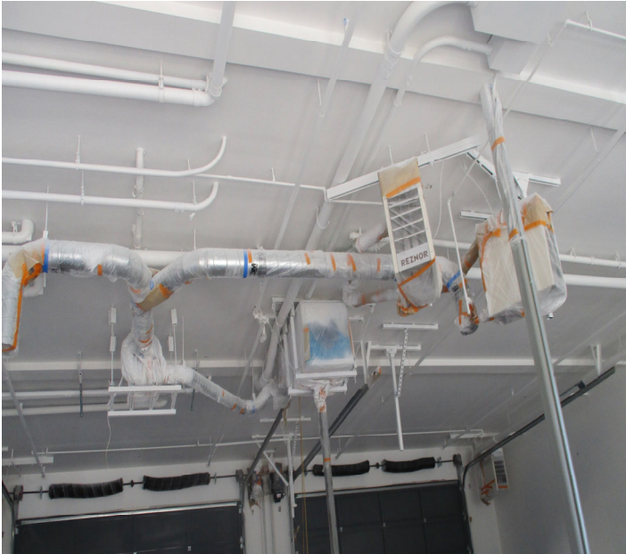
Painting Apparatus Bay Ceiling
