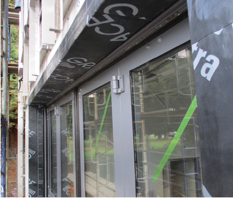
SAF Grace Ultra Flashing at Folding Apparatus Doors.
