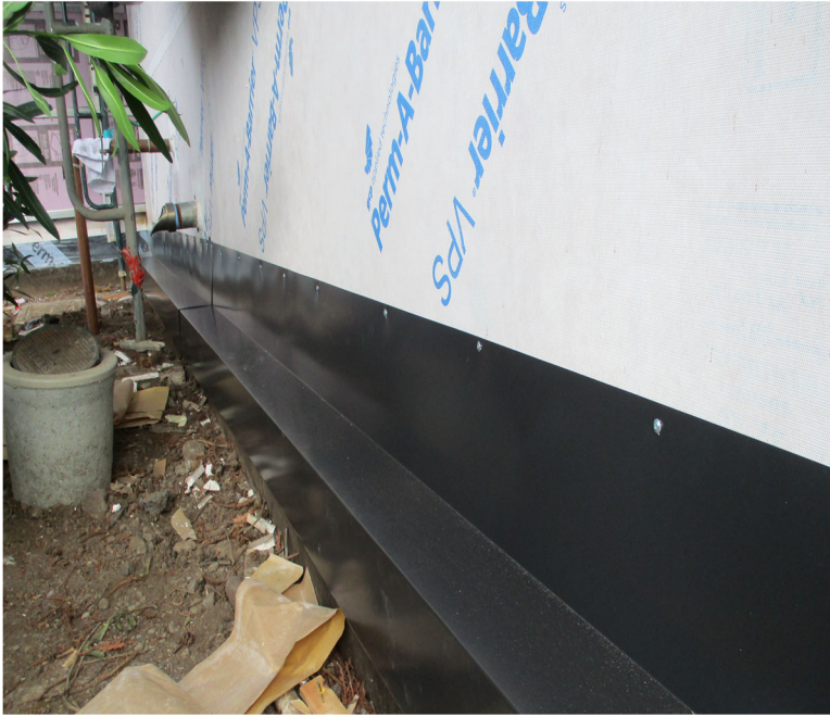
Aluminum Base Flashing Installation
