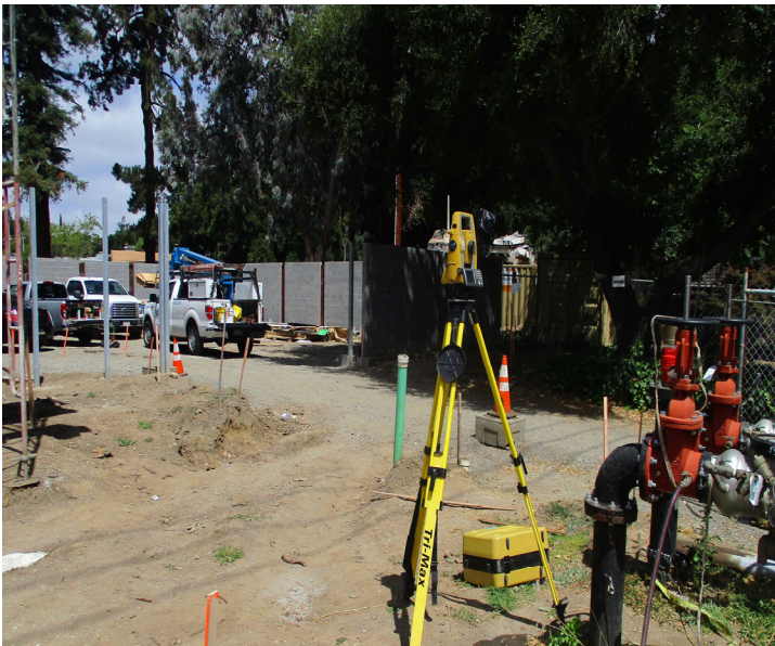
Parking Lot Site Survey
