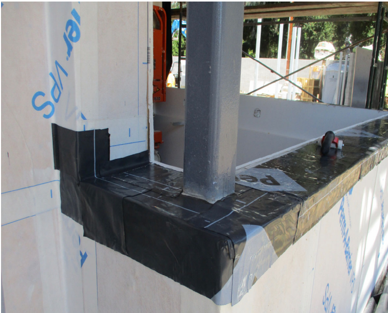
SAF Flashing at Watch Room
