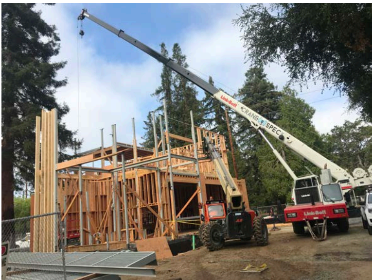
Crane placing second story steel.
