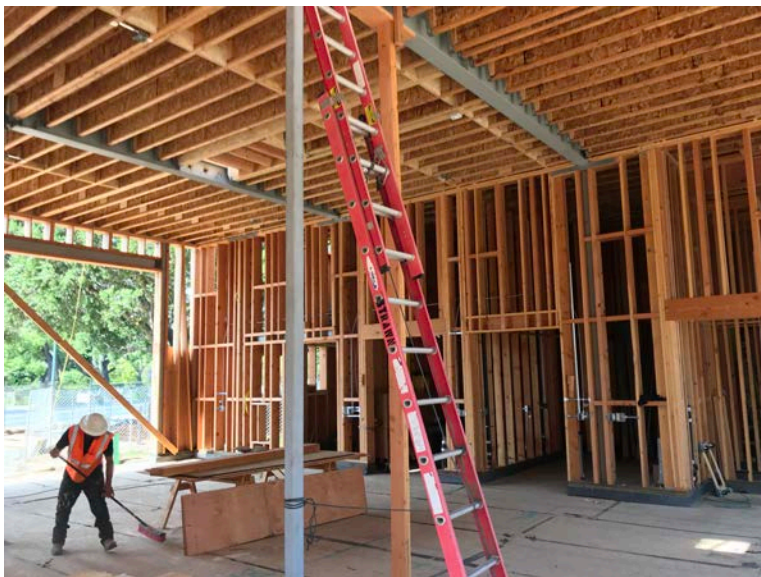
Interior structural framing in apparatus bay.
