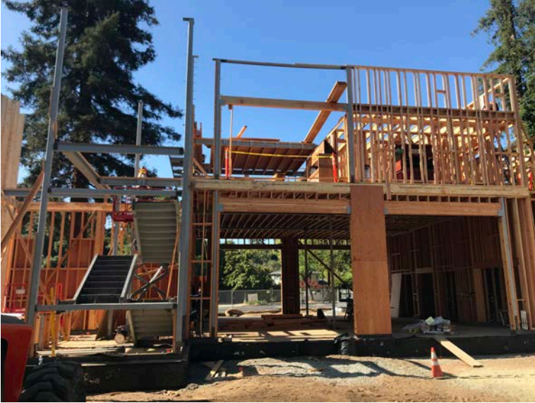
Structural framing from the north side.
