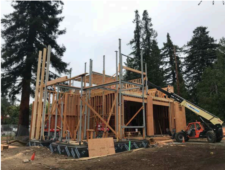
Second story structural framing started.
