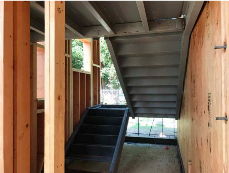
Metal stairs installed.
