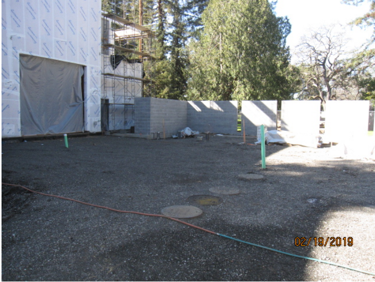
Finish grade of back parking lot.
