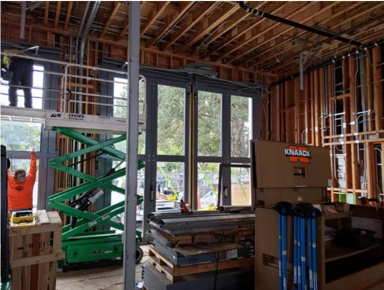
Bi-Fold front doors installed with glass
