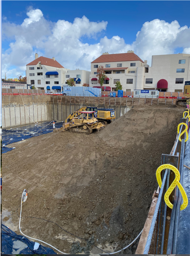
Mass Excavation ongoing.
