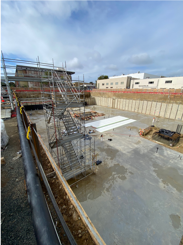
Mud slab in place in Area A.
