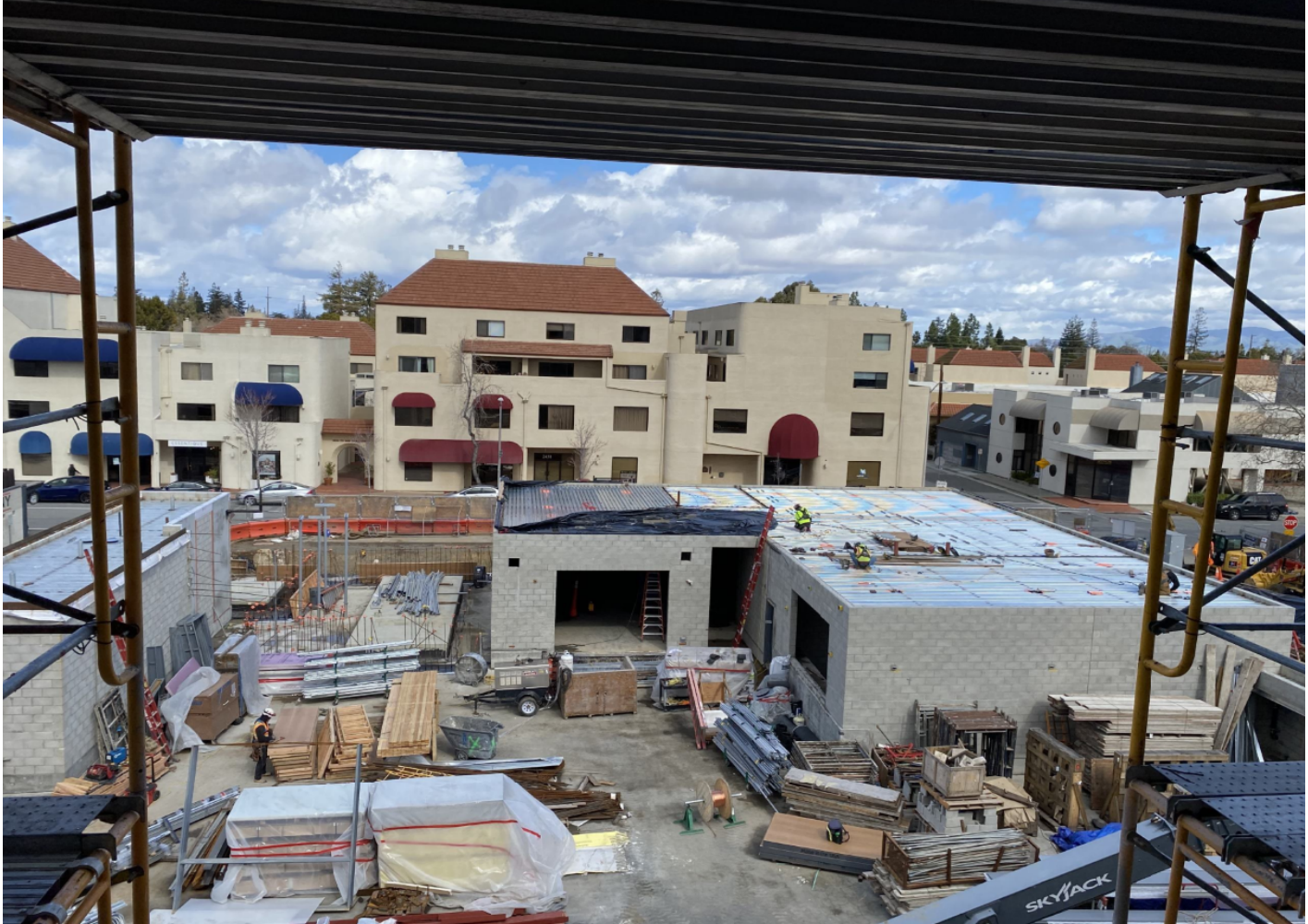
View of Utility Yard from Building
