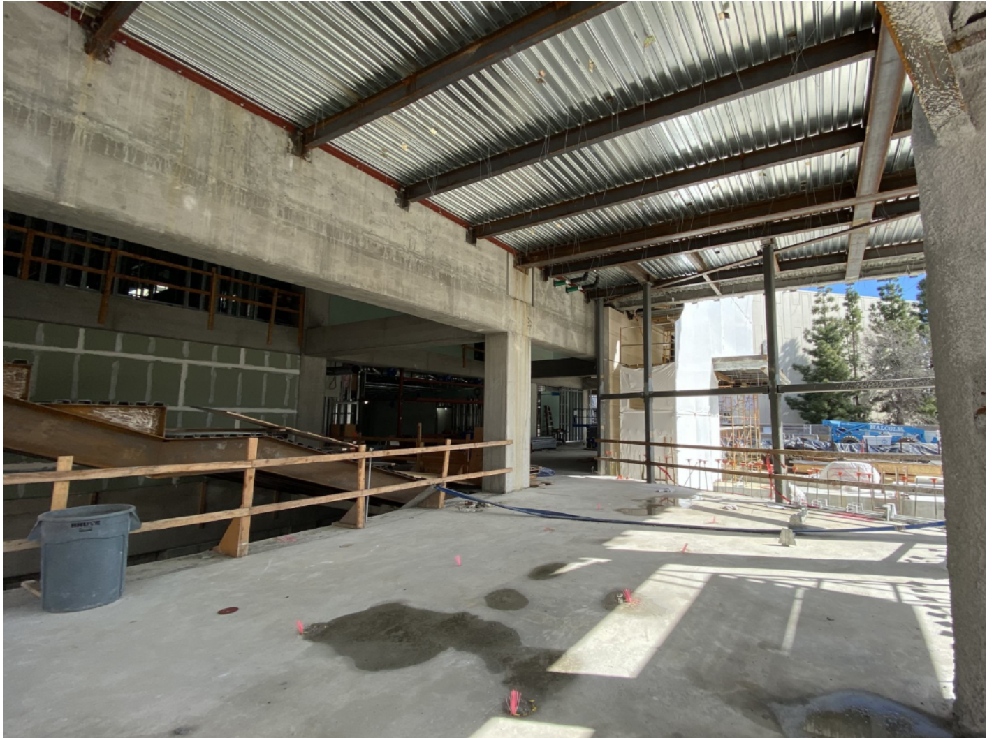
View of Multi-Purpose Room .
