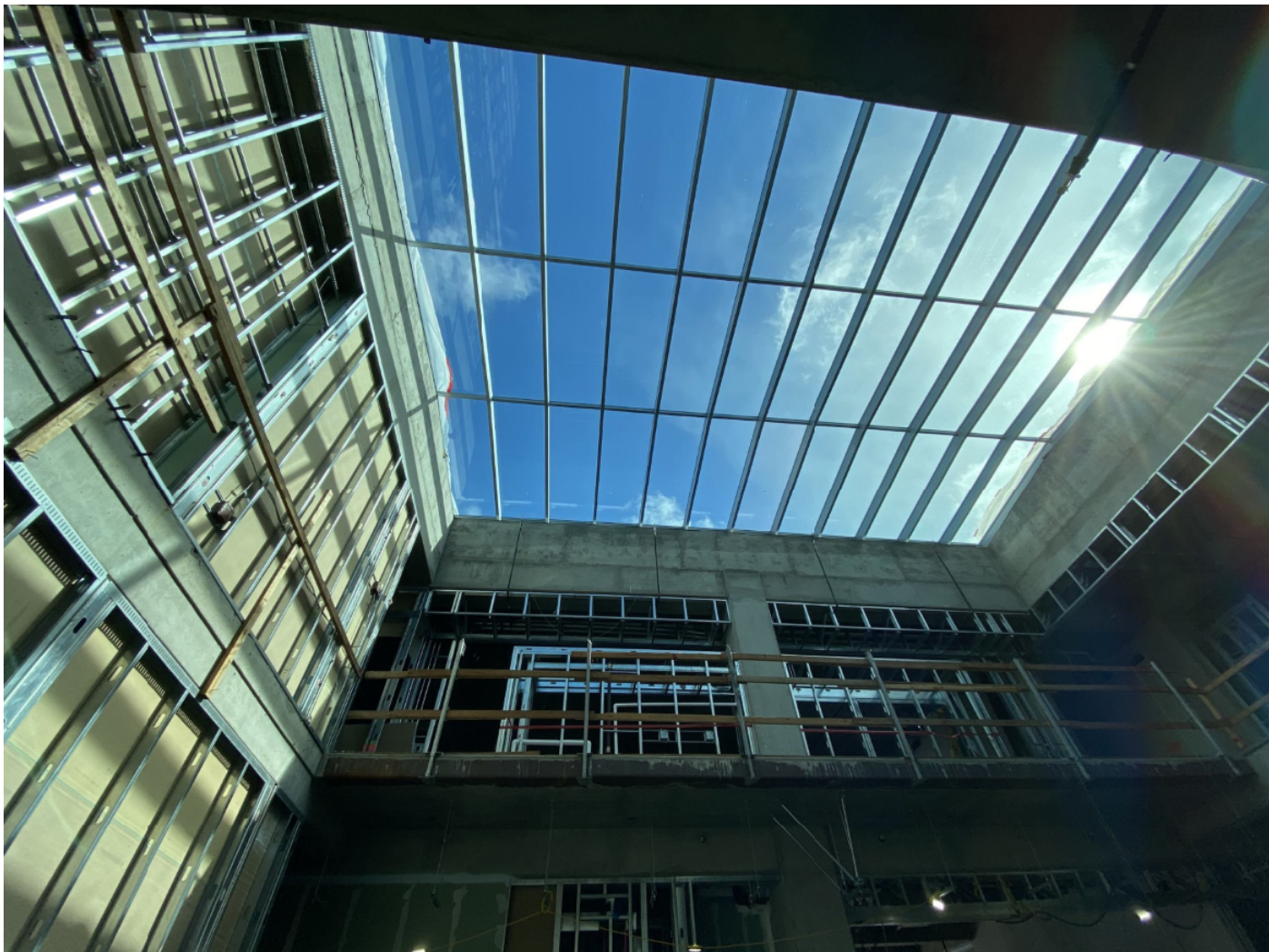
View of Skylight from Level 2.
