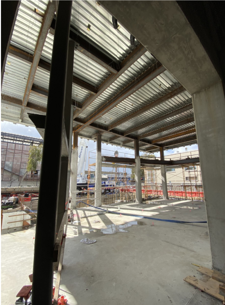
View of Multi-Purpose Room.
