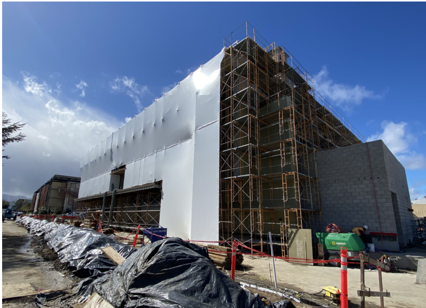
View from South elevation.
