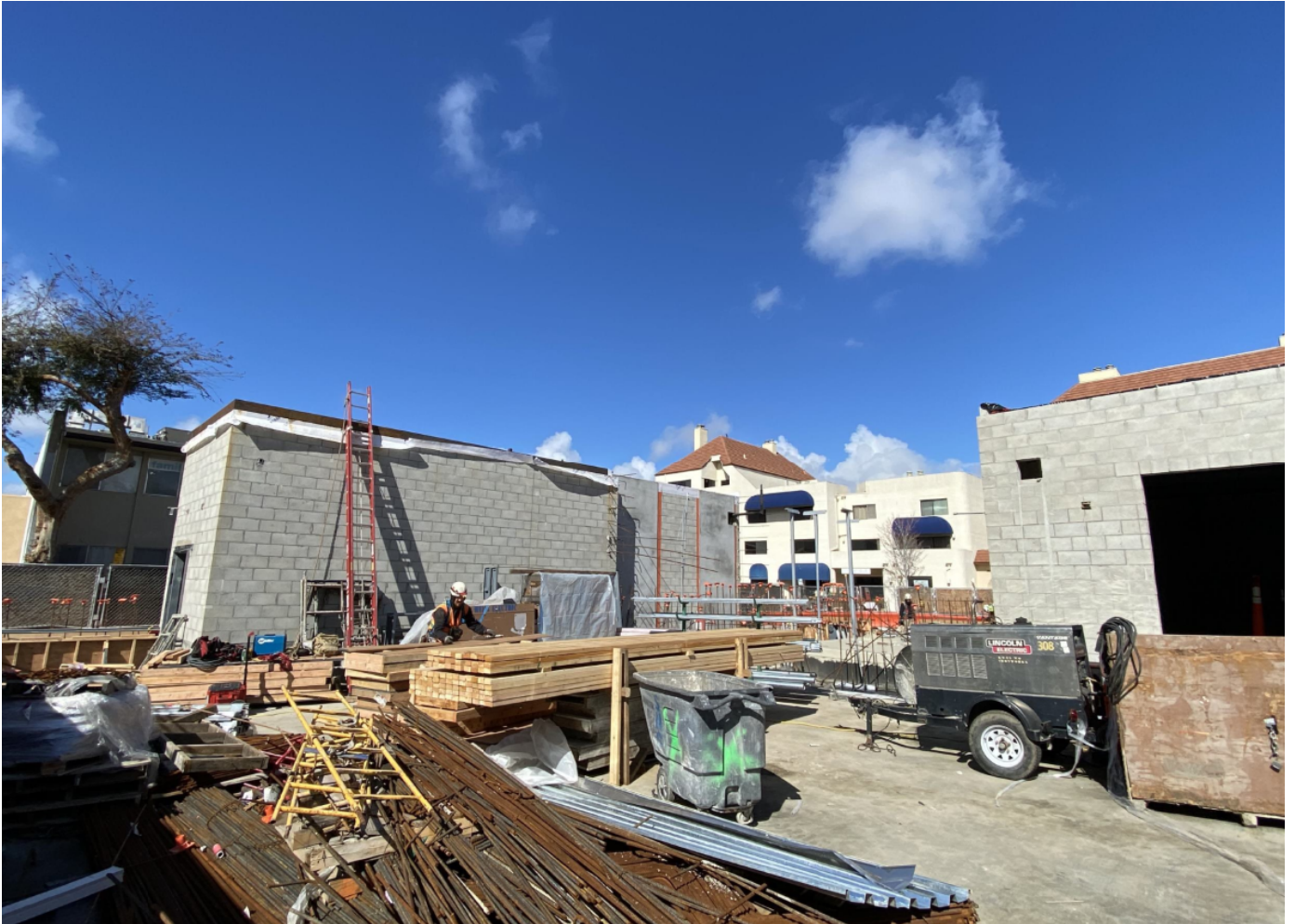
View from Utility Yard
