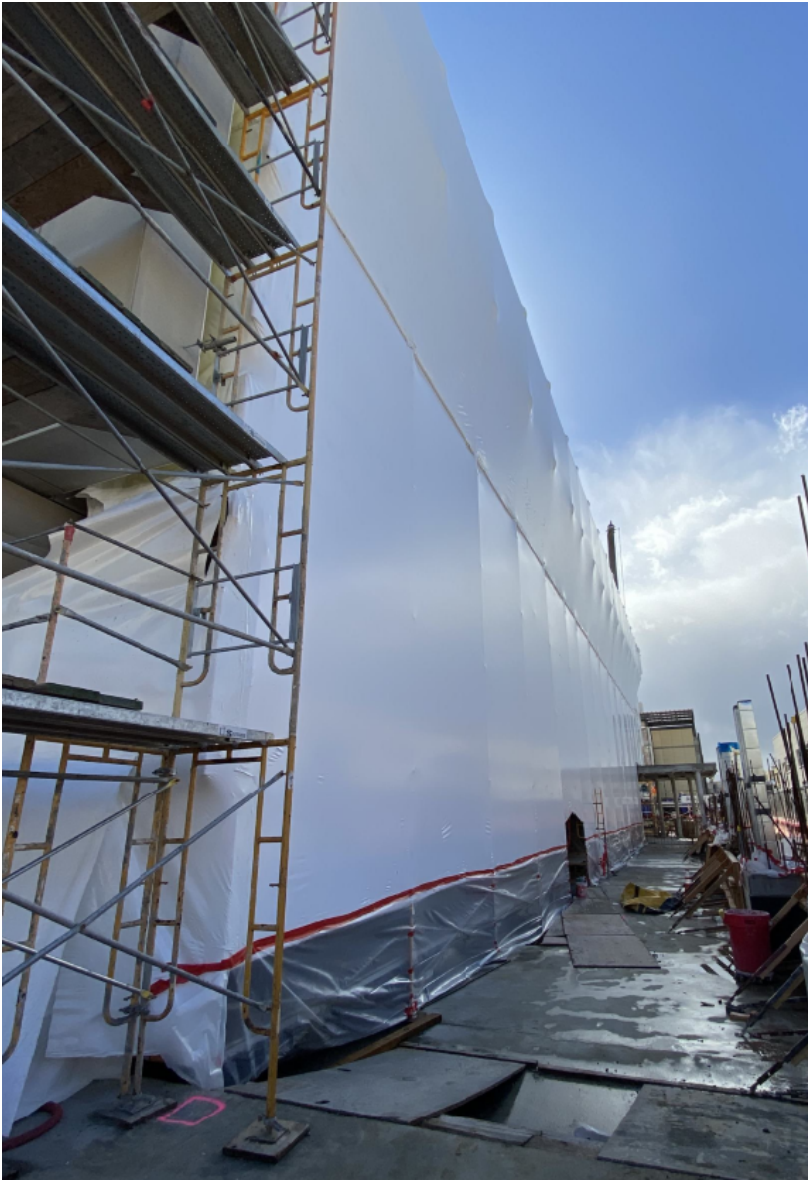
View from North elevation capturing Exterior Tile cover.
