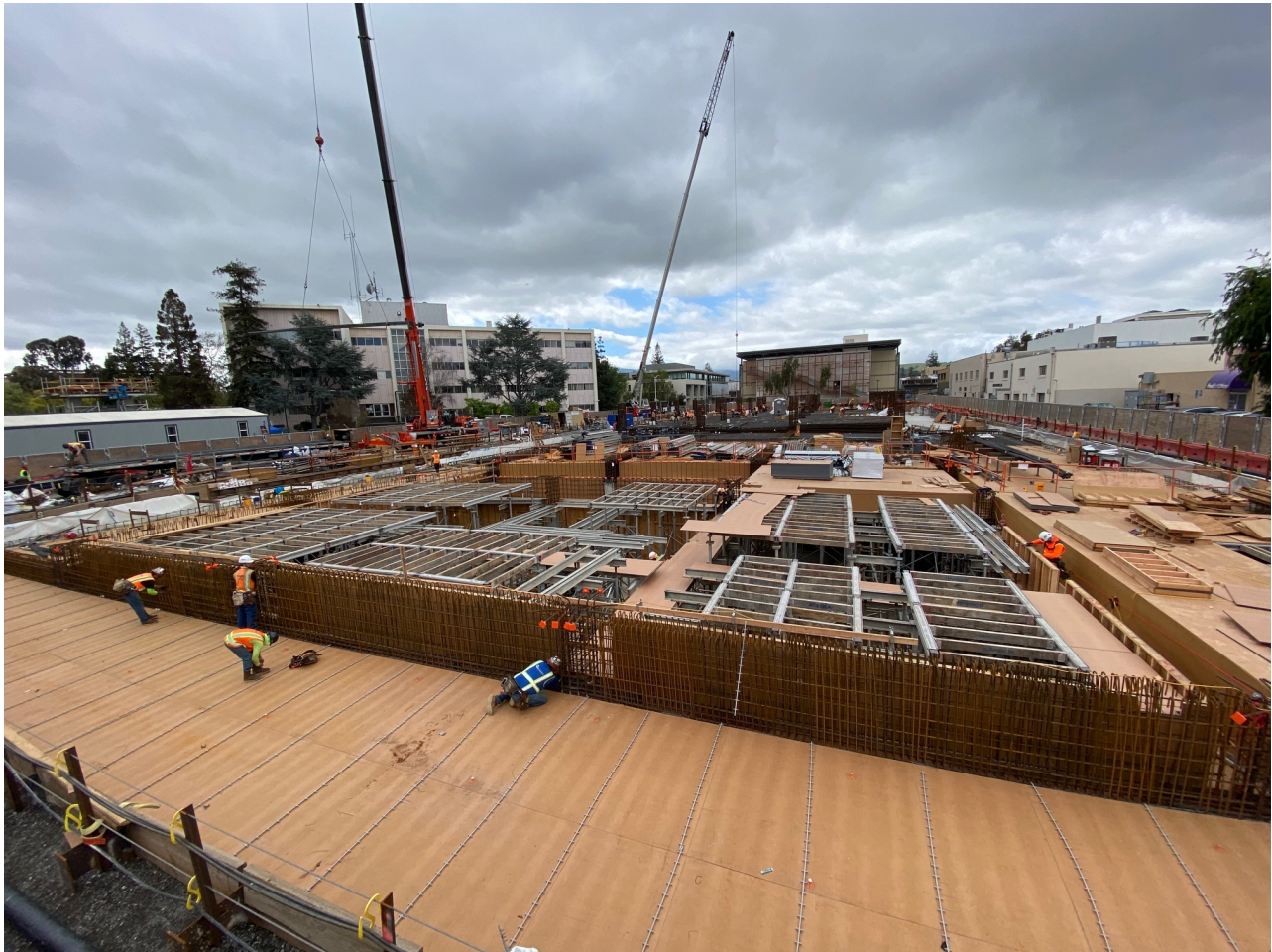
Formwork in place for Level 1 concrete slab.
