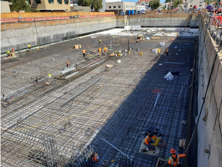
Mat foundation rebar and in-slab utilities being installed.
