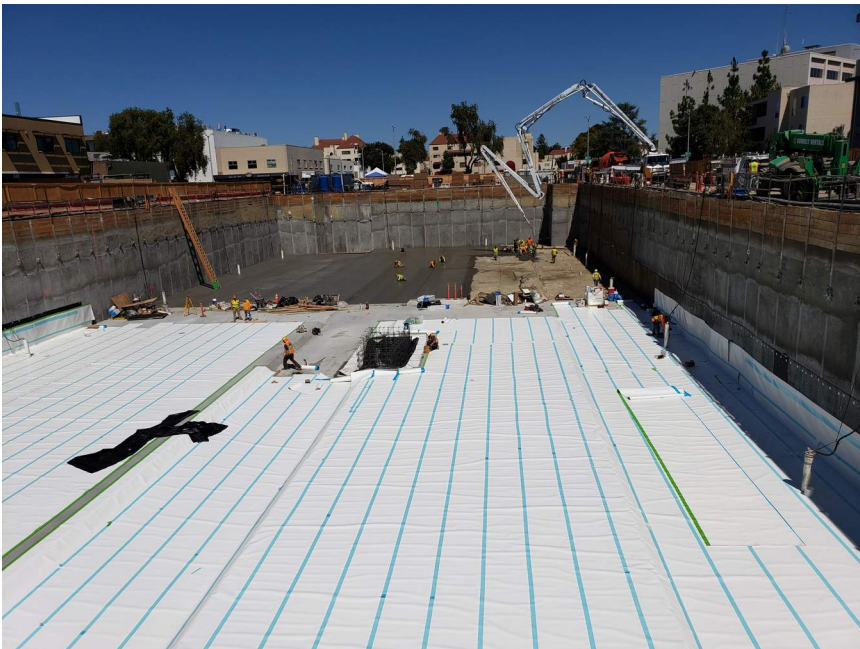
Below grade waterproofing installation ongoing, rat slab pour occurring in background.
