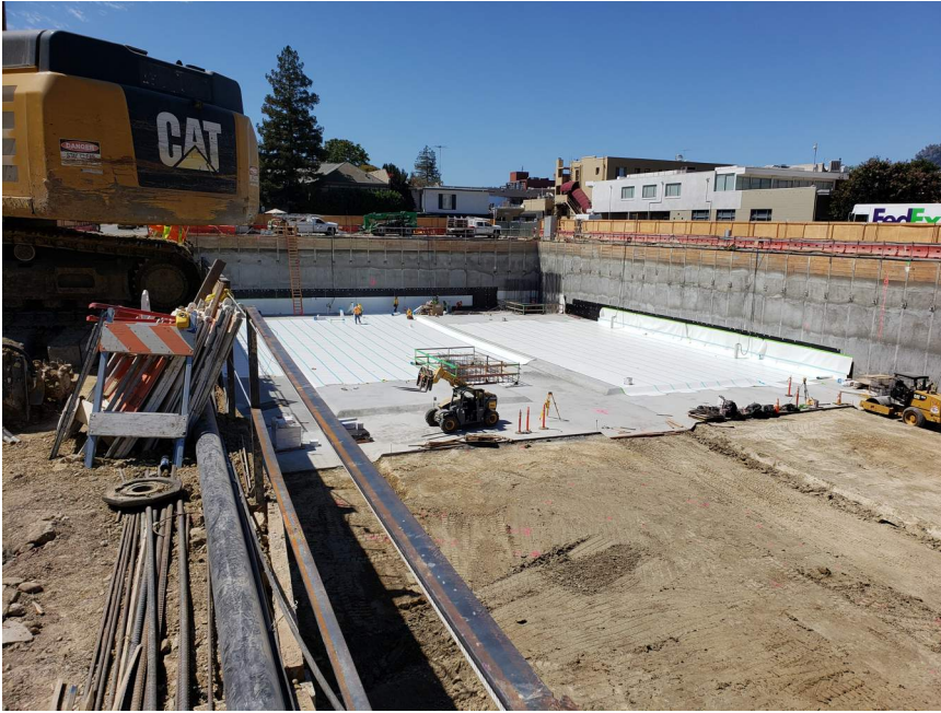
Mass soil excavation activities concluding.
