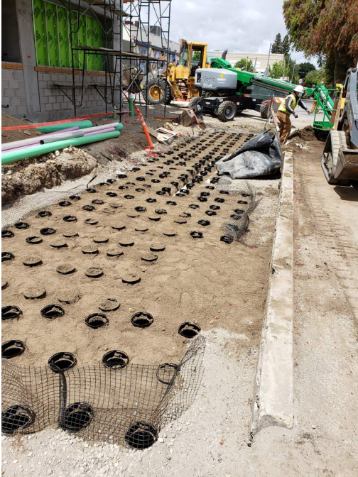
Silva cell installation along Birch St.
