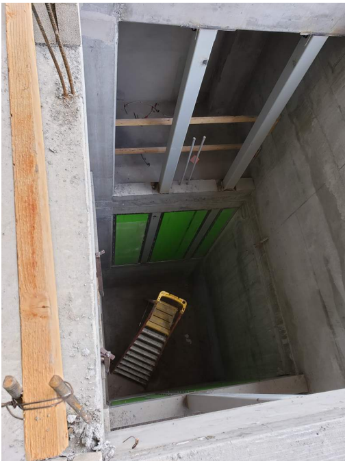
Elevator shaft framing progress.
