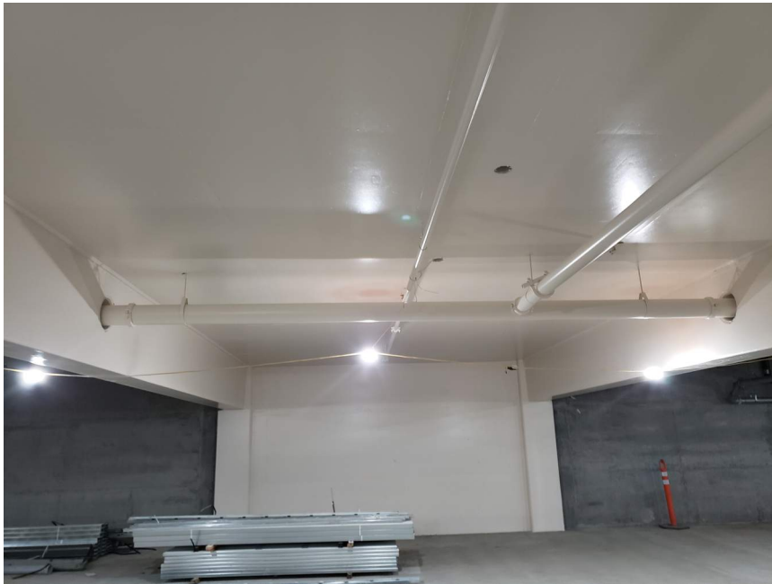
Paint mockup review in basement level.
