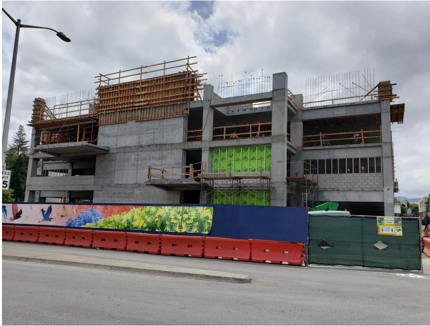
Exterior progress of Birch St. elevation.
