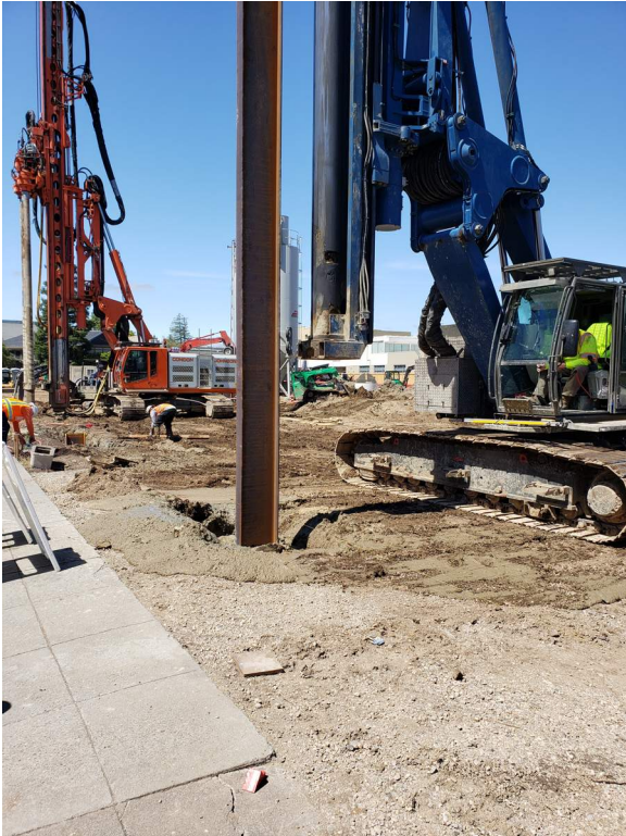
Steel for cut-off wall being installed along Sherman Ave.
