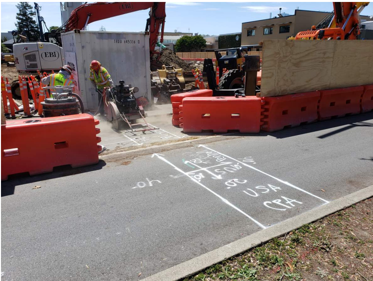
Preparation for utility tie-in at Birch St.
