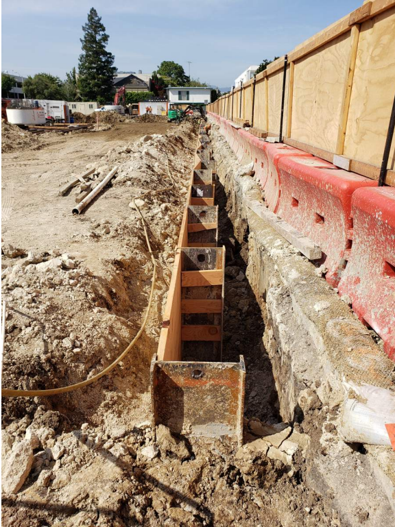
Wood lagging installed along shoring wall.
