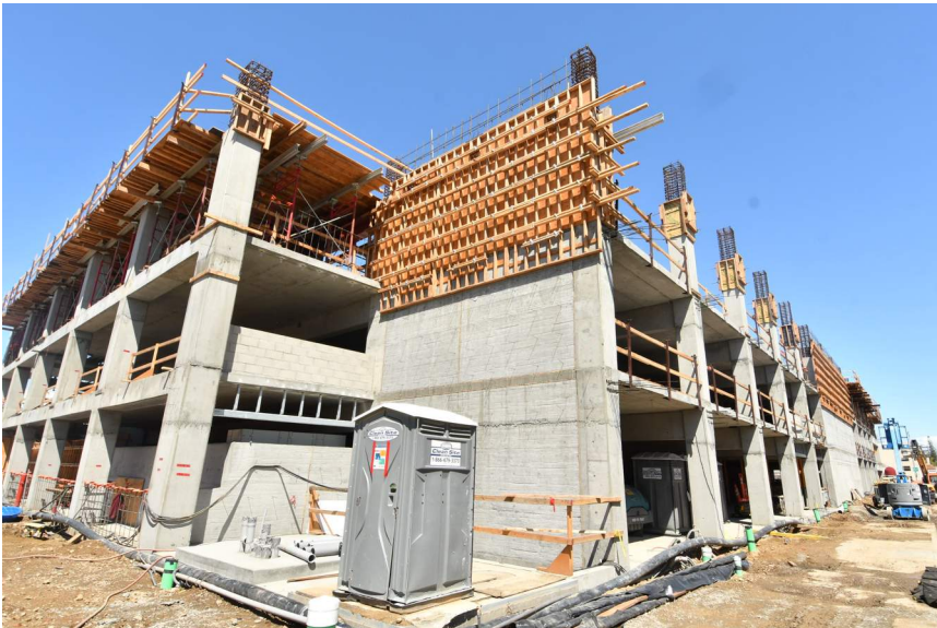
Progress view from corner of Ash St. and Sherman Ave.
