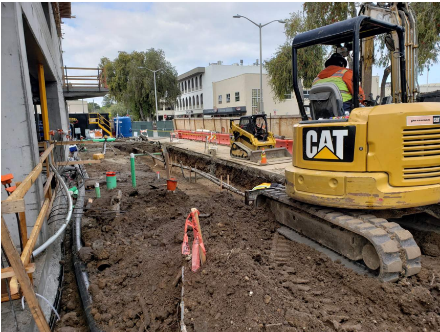
Excavation for Silva Cells along Birch St.
