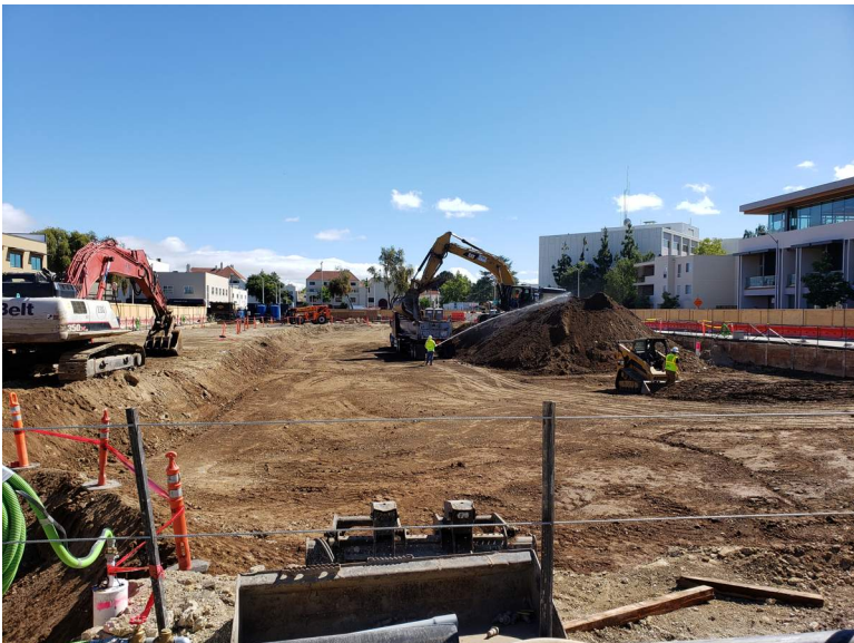
Mass soil excavation in progress.
