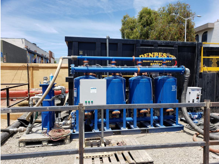
Dewatering treatment system being setup onsite.
