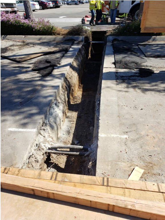
Sanitary Sewer tie-in being installed along Birch St.
