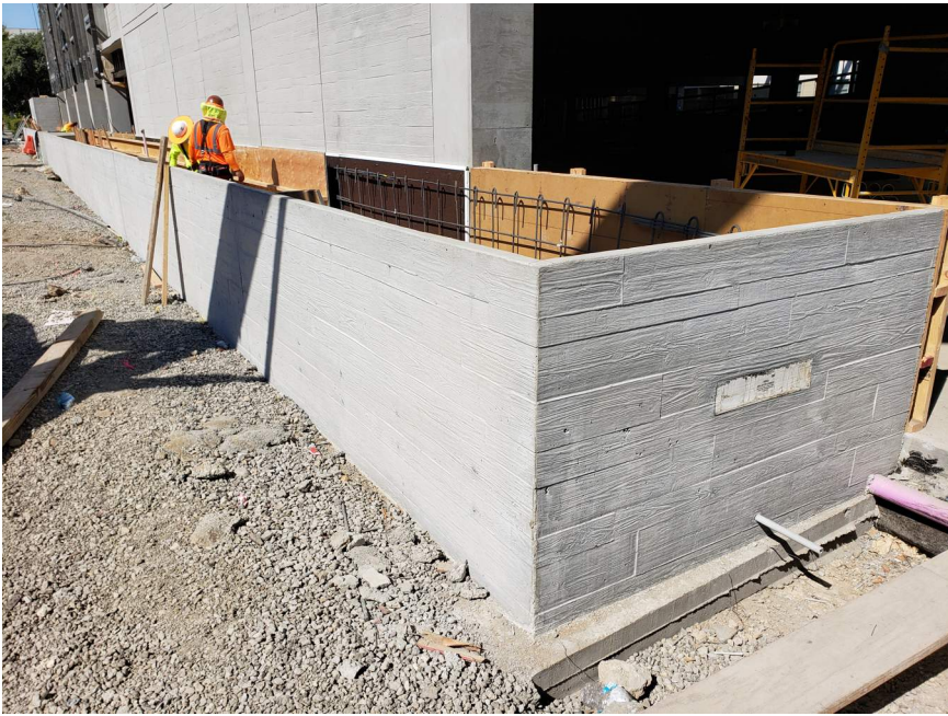
Planter wall on Sherman Ave.
