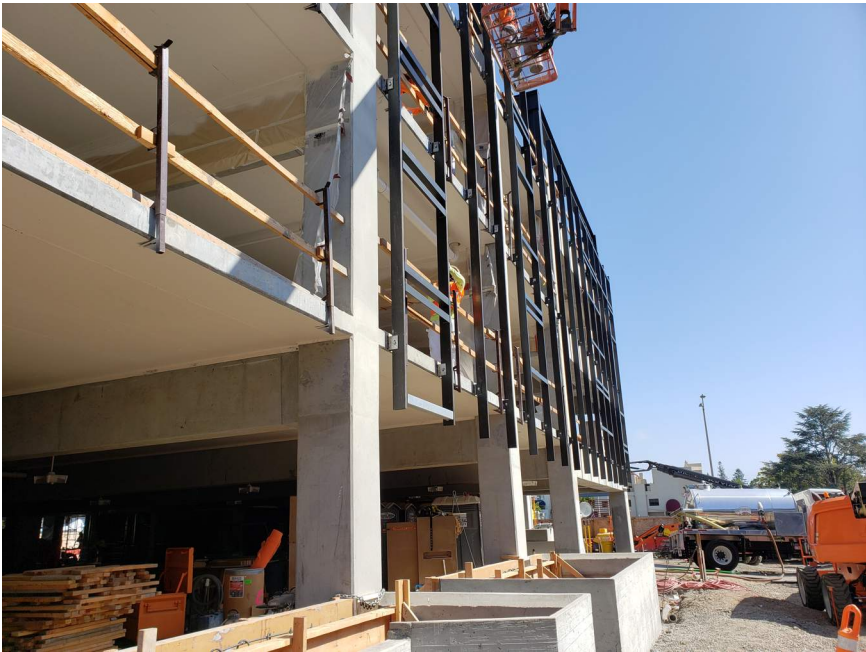
Painting of Terra Cotta supplemental steel ongoing.
