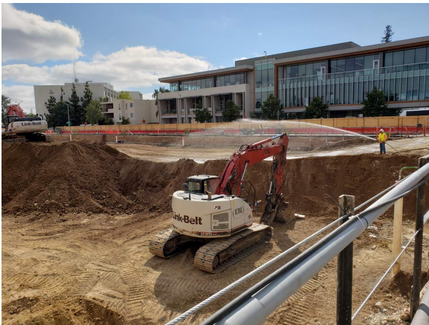
Contractor implementing dust control measures.
