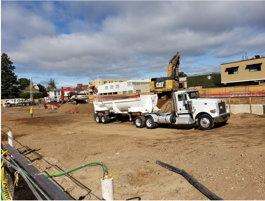
Mass soil excavation in progress.
