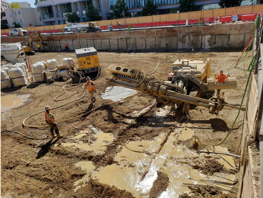
Tieback drilling along Ash St.
