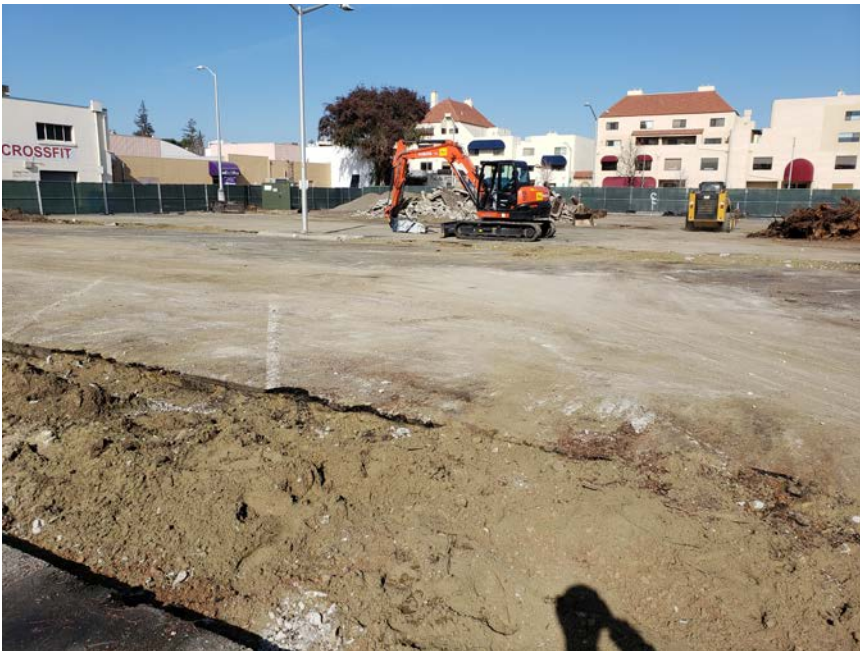
Concrete island demolition and removal.
