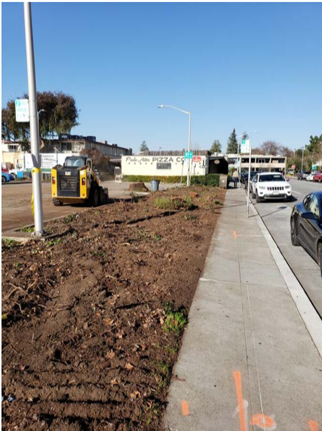
Parking lot ready to be reopened to the public.
