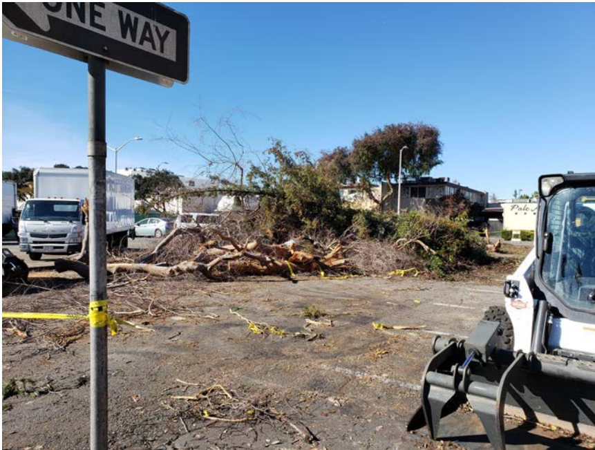
Tree removal and debris off haul at Lot C-6
