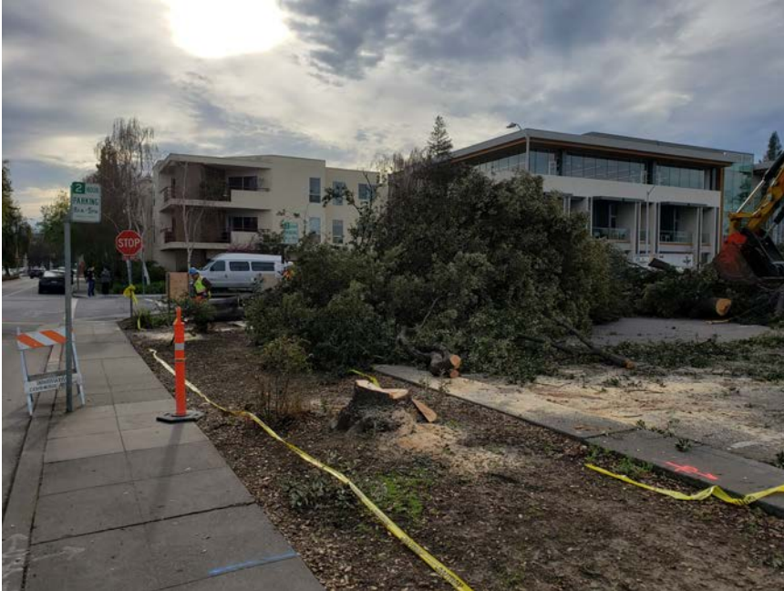
Tree removal at Lot C-7.
