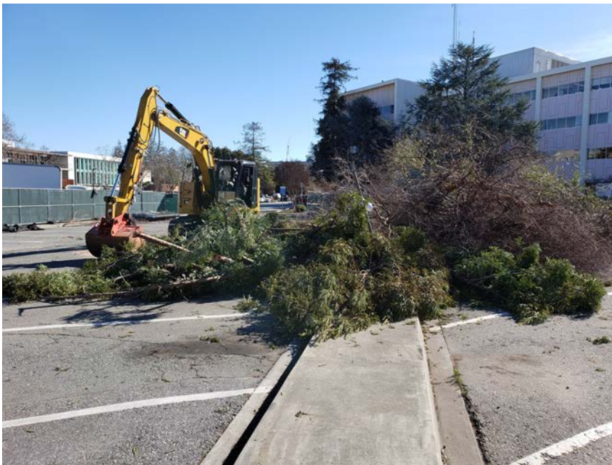
Tree removal at Lot C-6.
