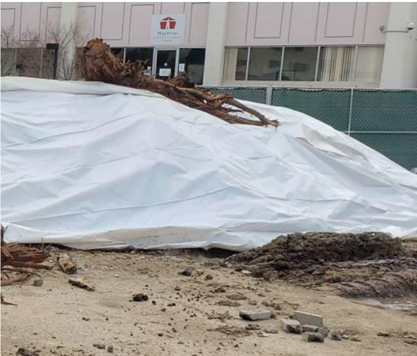
Off-haul of tree and demo debris.
