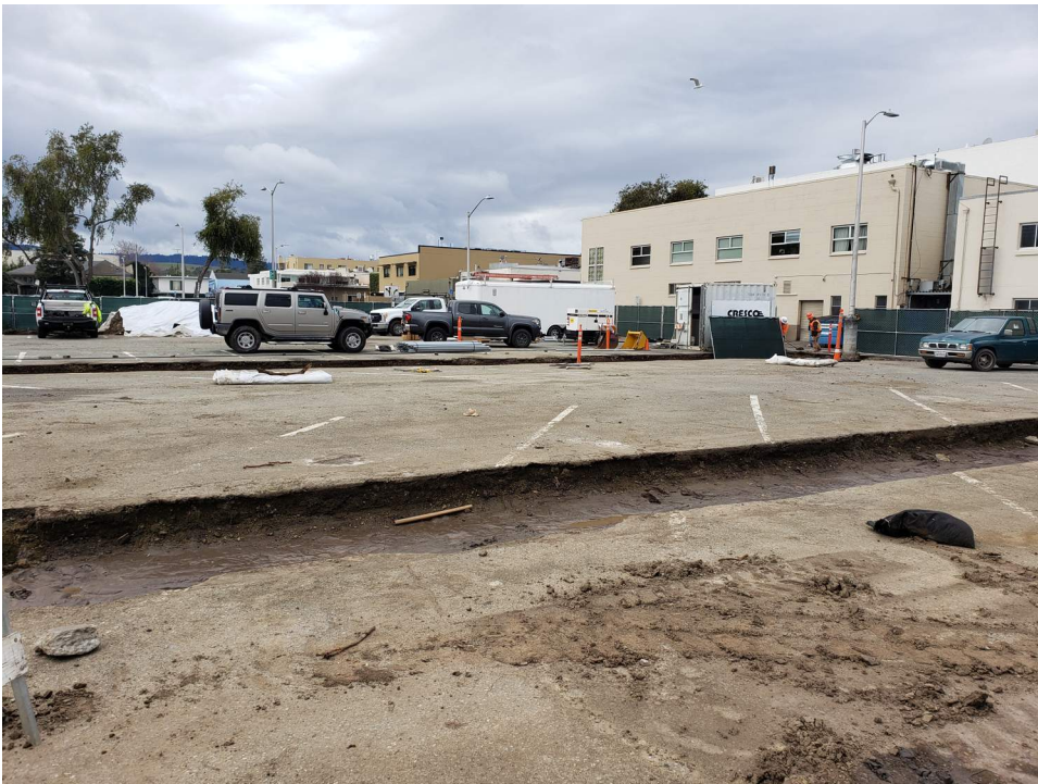
Compaction of subgrade at existing islands.
