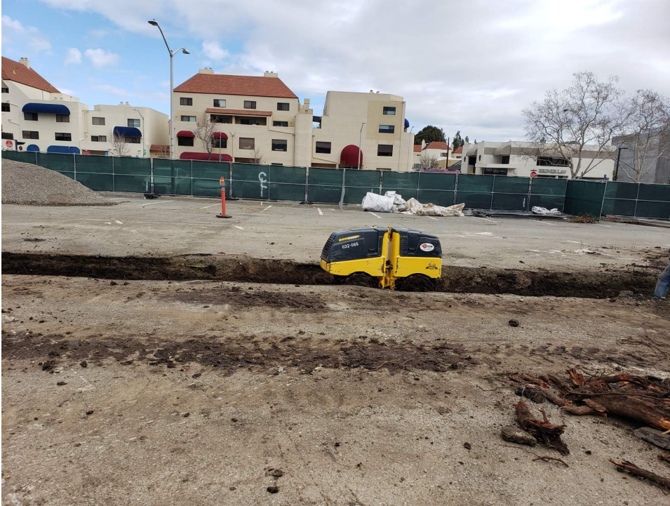
Compaction of subgrade at existing islands.
