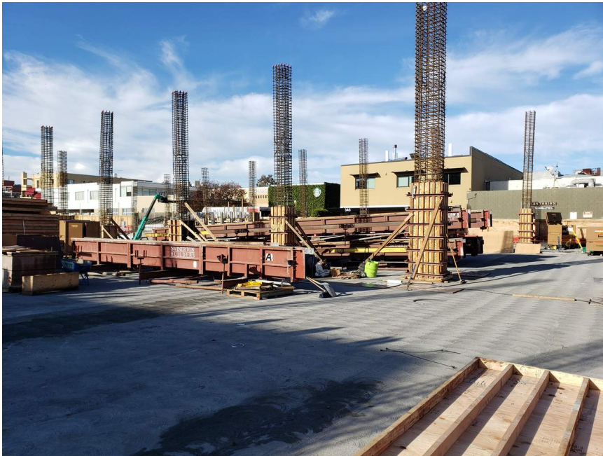
Ground level columns being formed.
