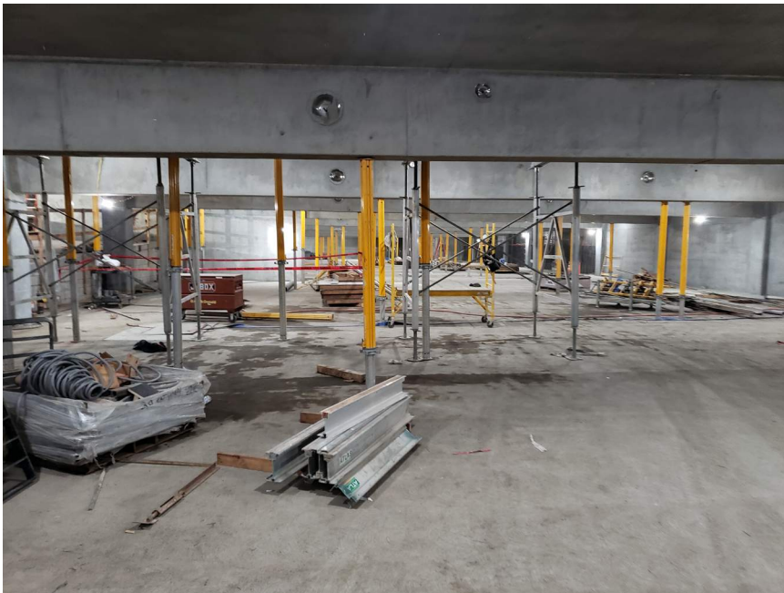
Re-shores in place at the basement levels.
