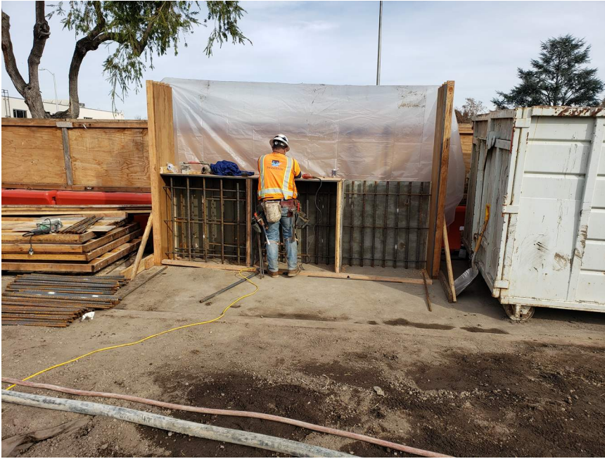
Shotcrete test panel being constructed.
