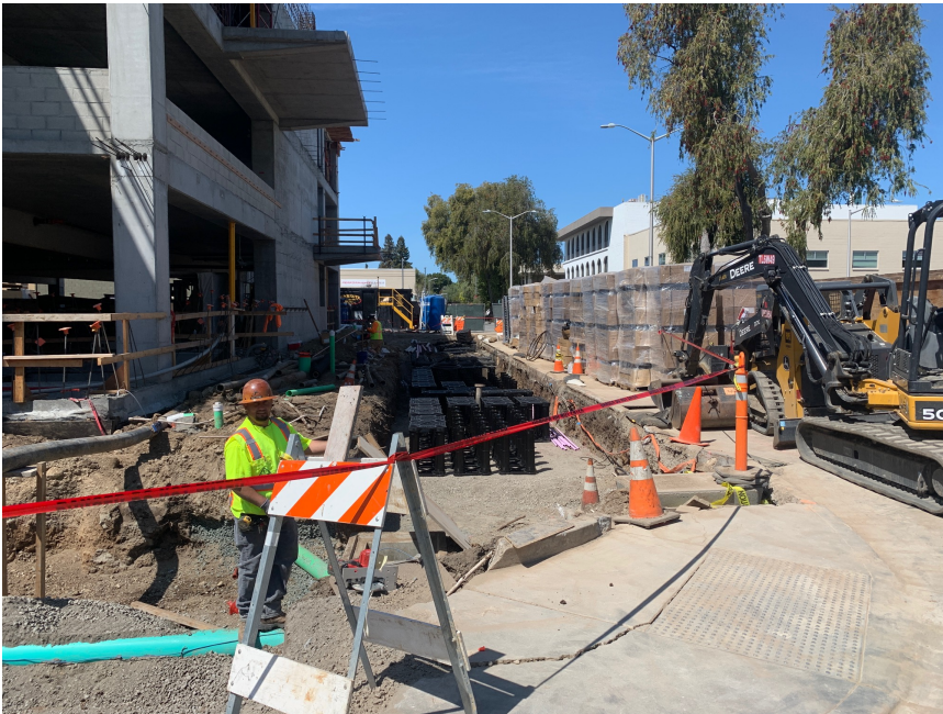
Layout of Silva Cells along Birch St.
