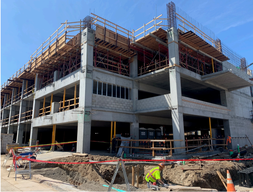
Progress view from corner of Birch St. and Sherman Ave.
