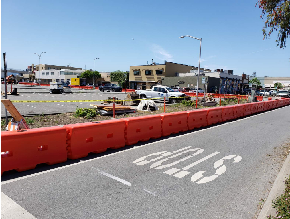
Barricades have been installed around lot C-7.
