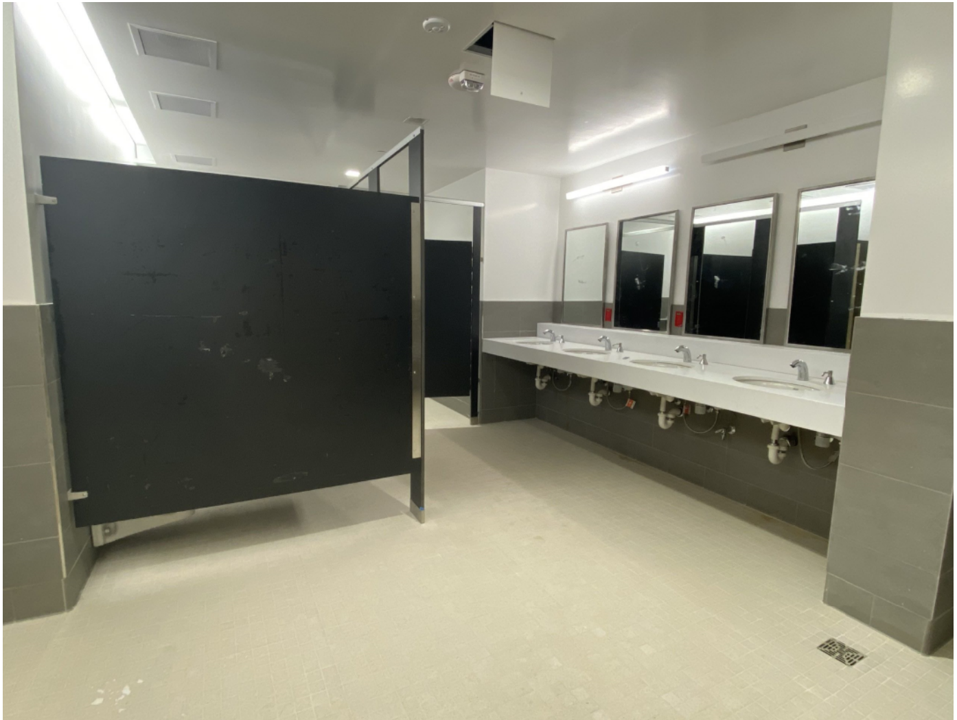
L2 Men's Restroom.
