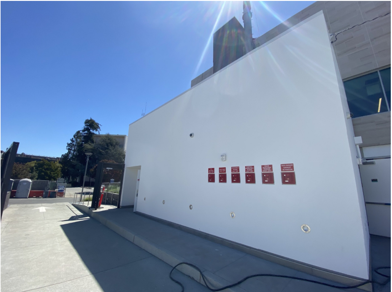
View of Signage installation in the Courtyard.
