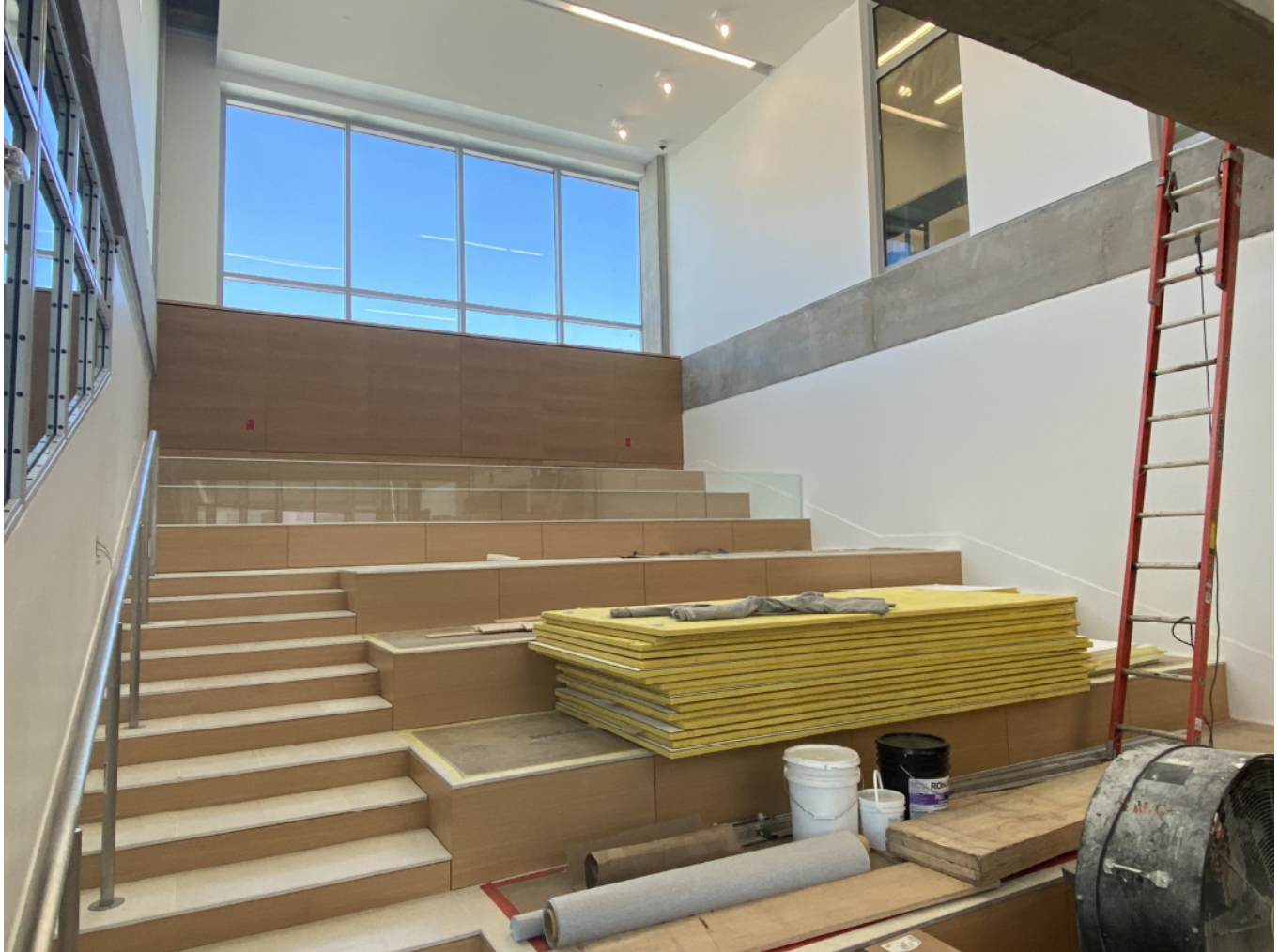
View of bleachers on L1 Lobby.
