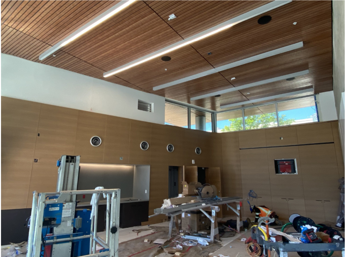
View of Multi-Purpose Room.
