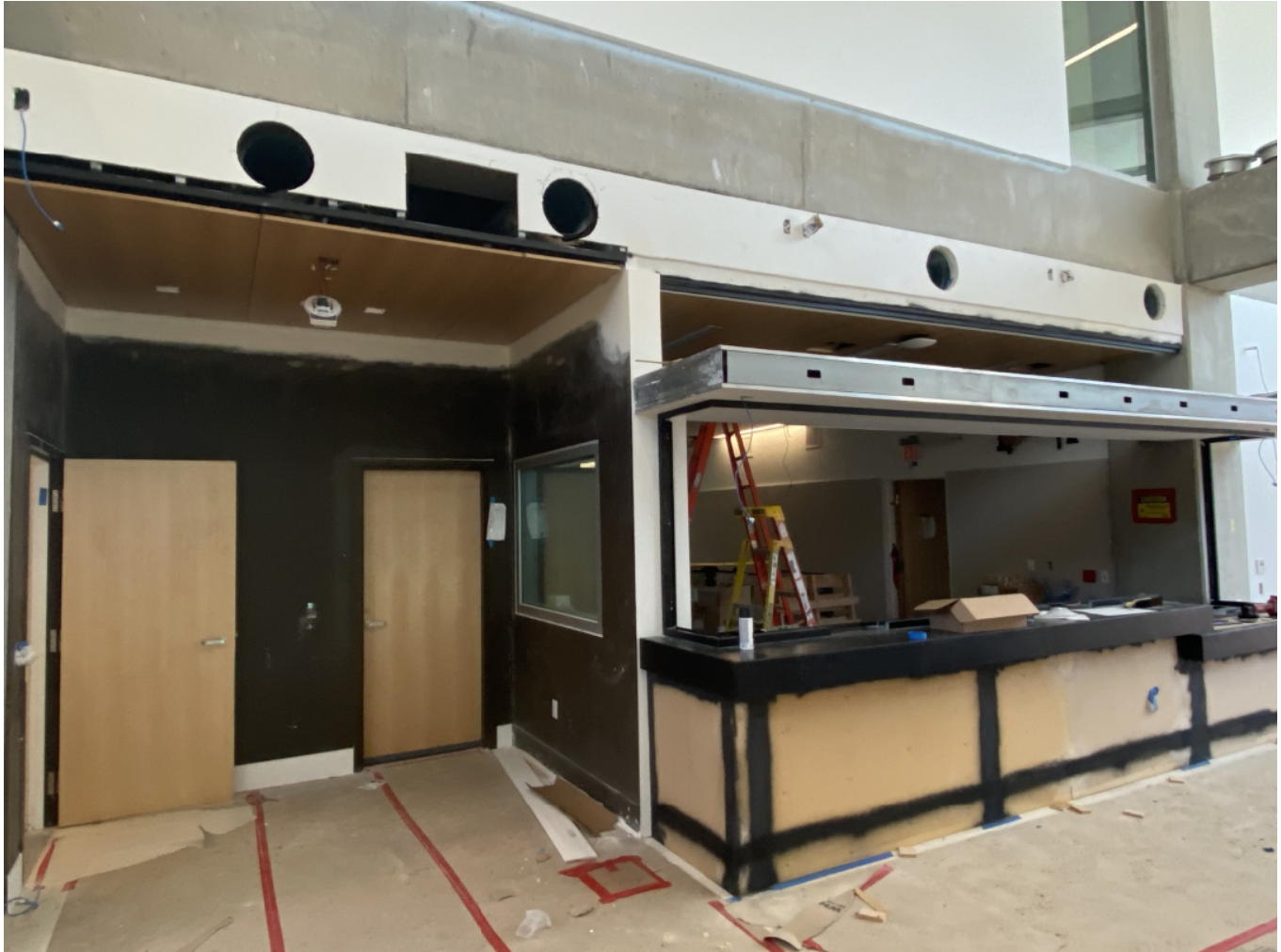
View of Public Counter on L1 Lobby.
