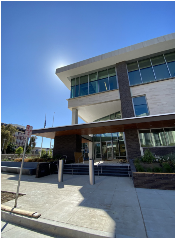
Front entrance Sherman Ave.
