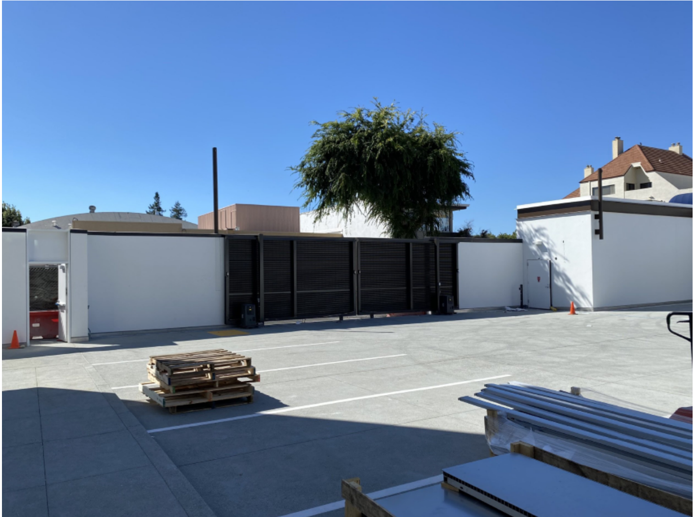
Interior utility yard gate.
