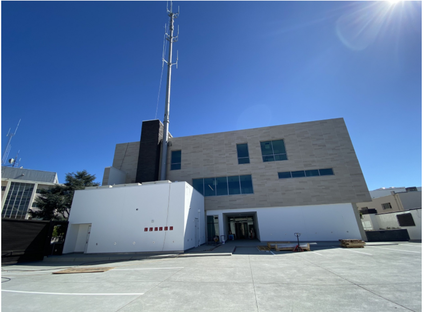
View of Utility Yard with Striping.
