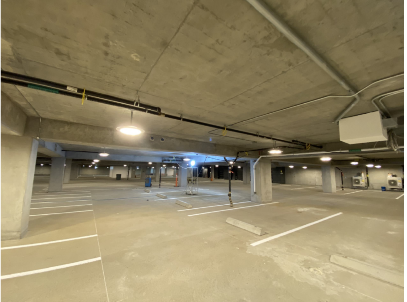
B2 Parking Lot Striping.
