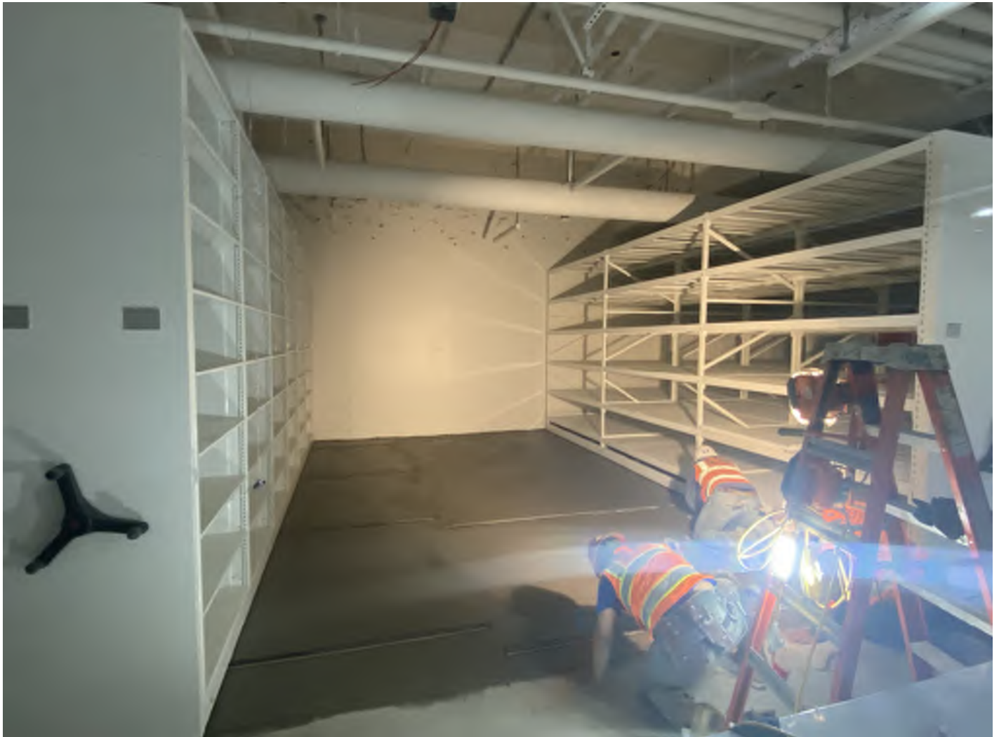
Depressed slab infill on B1.
