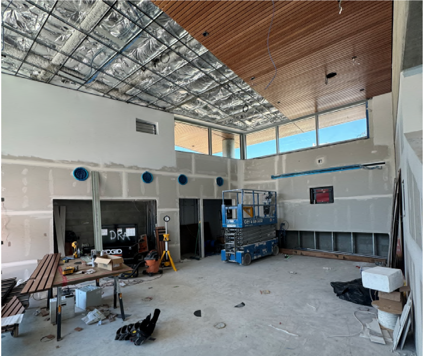
View of Multipurpose Room on L1.
