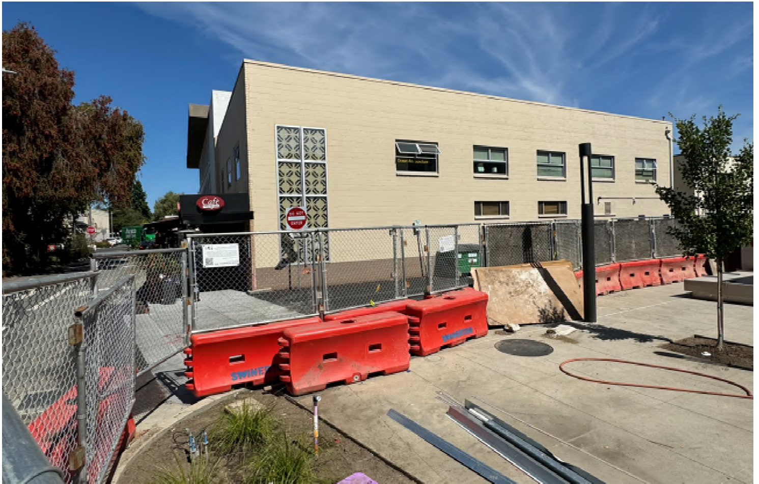
Jacaranda Driveway repair.
