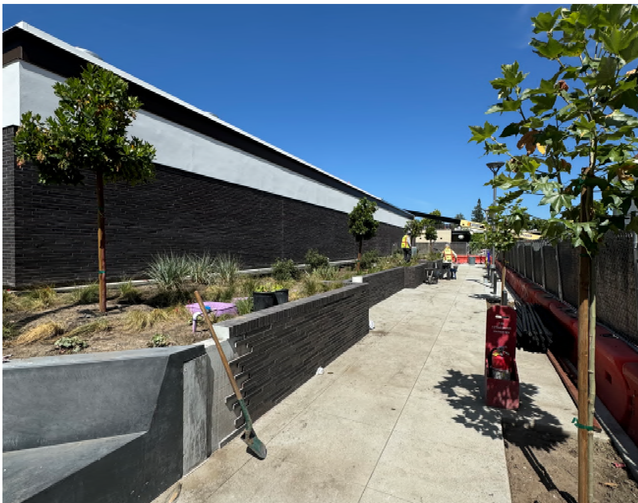
Park Ave Site Work.
