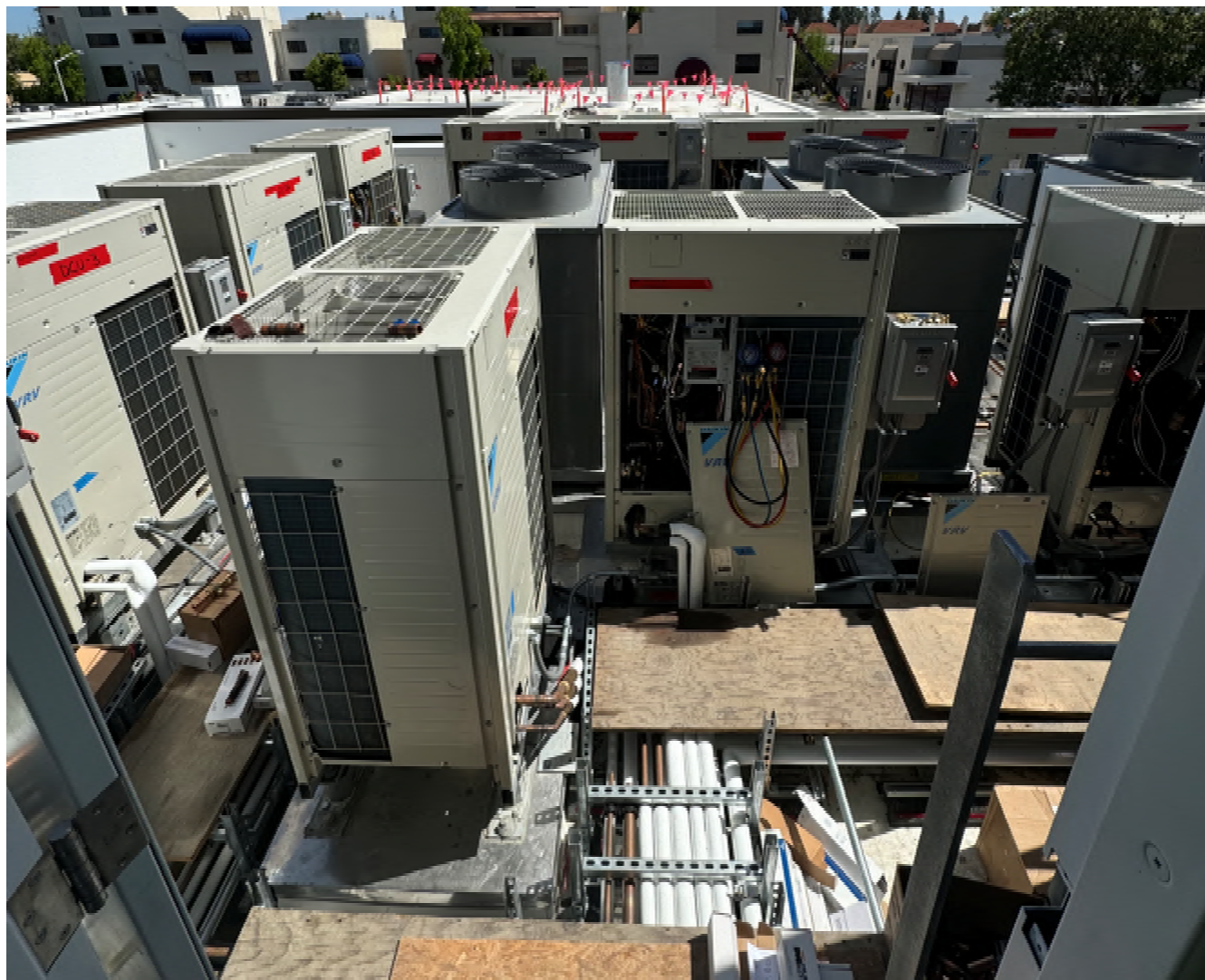
View of emergency Electrical Roof Unit Installation.
