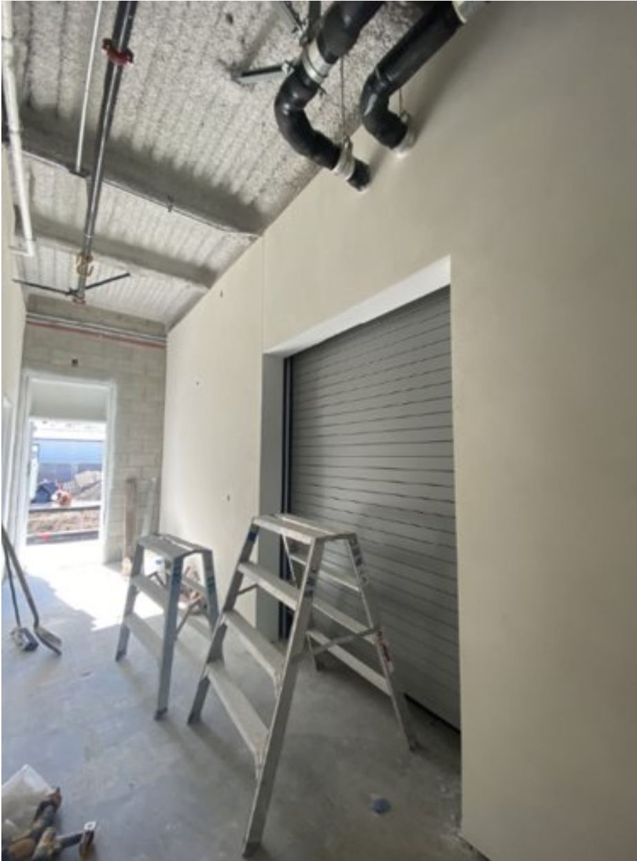
Utility Yard Coil Door Installation.
