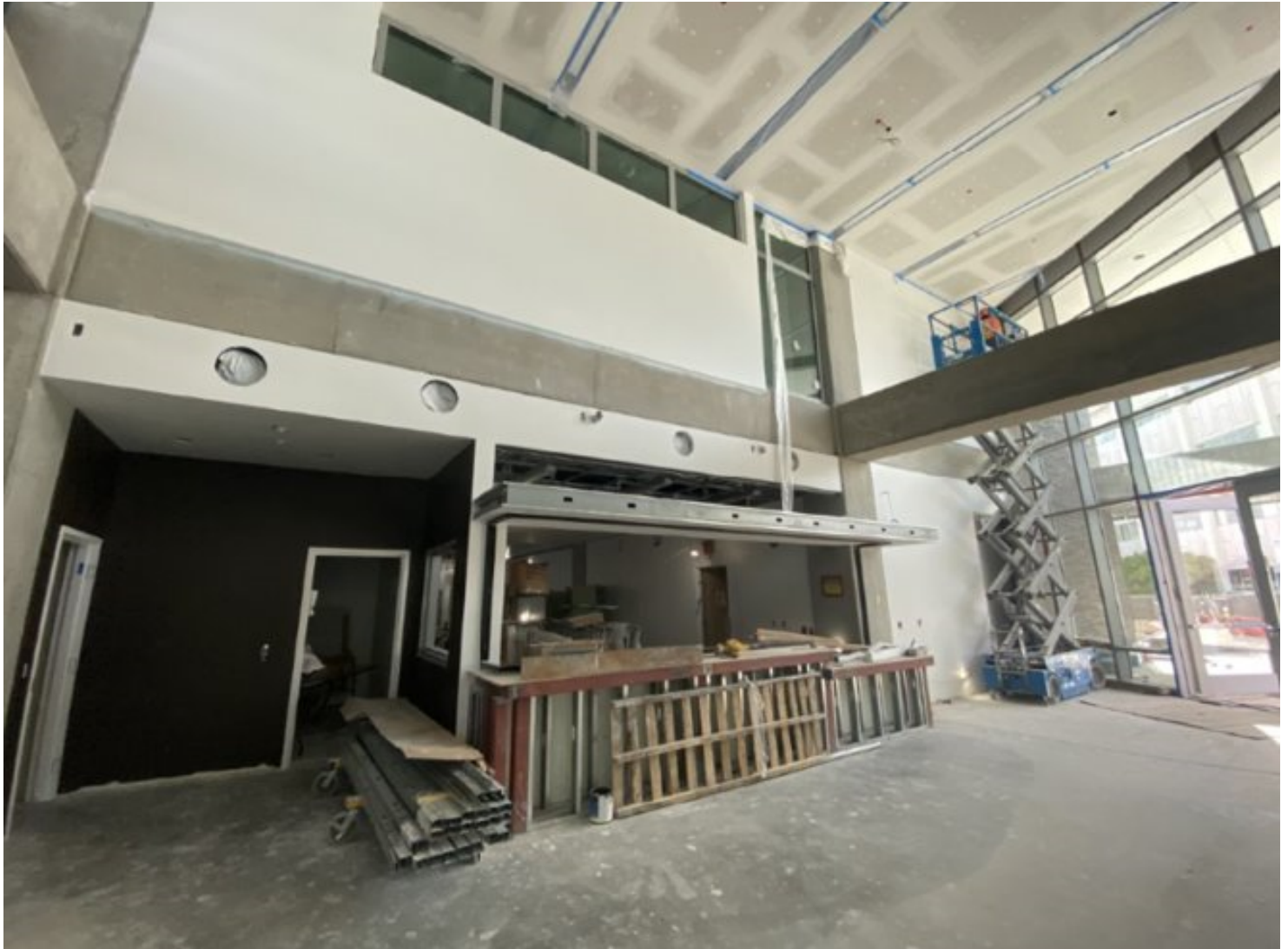
Public Lobby Counter.
