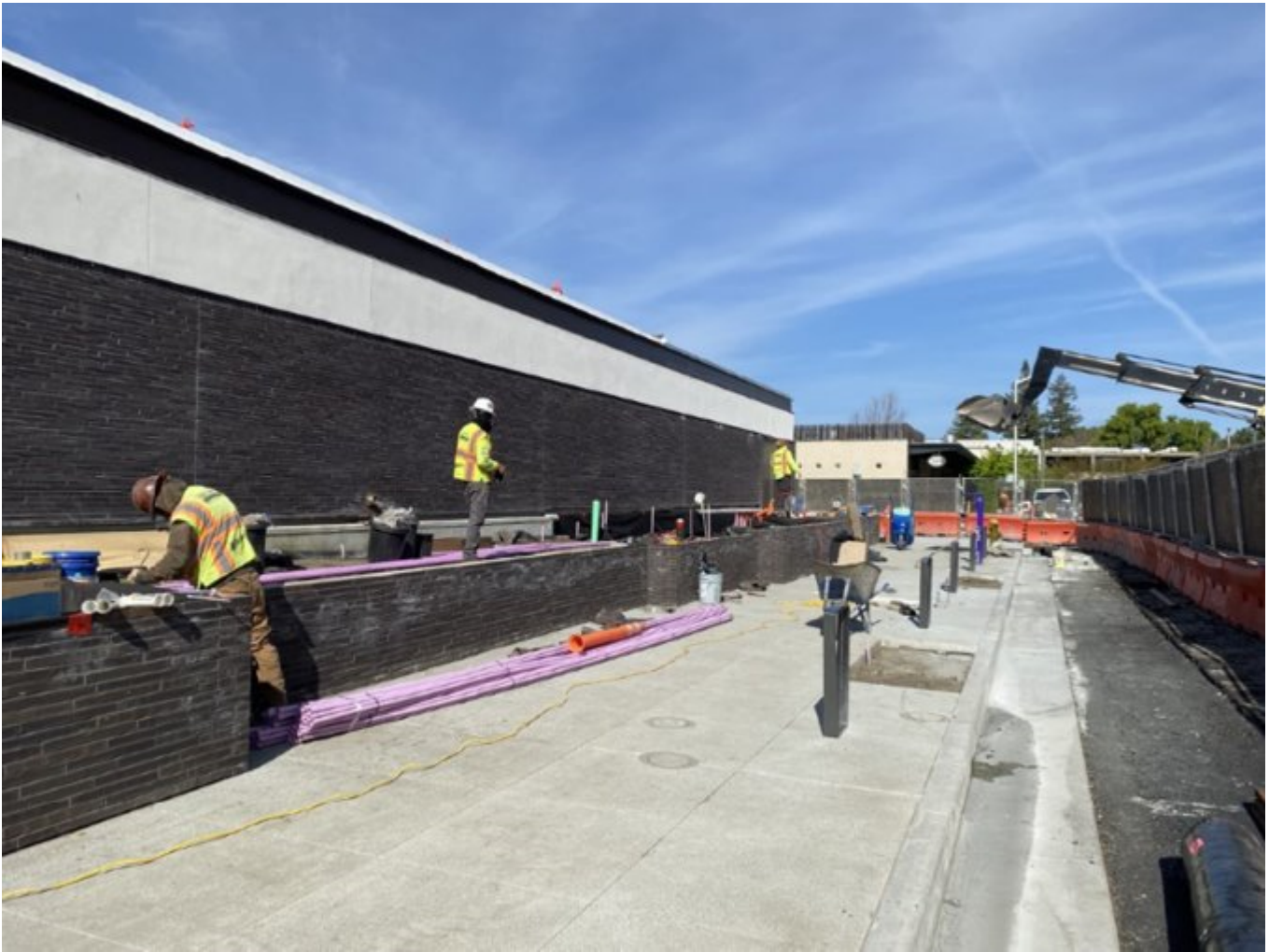
Park Ave Site Work.
