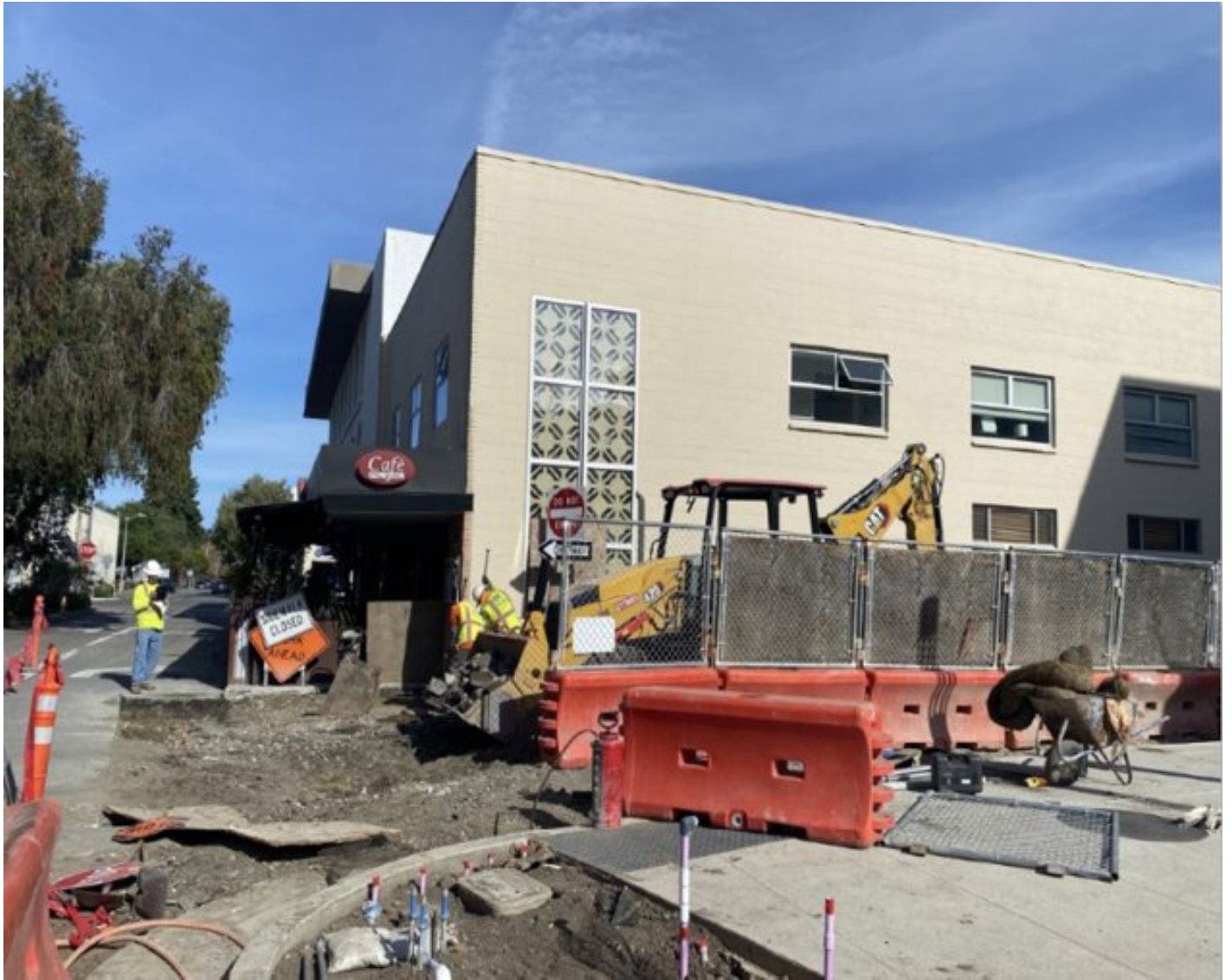
Jacaranda Driveway repair.
