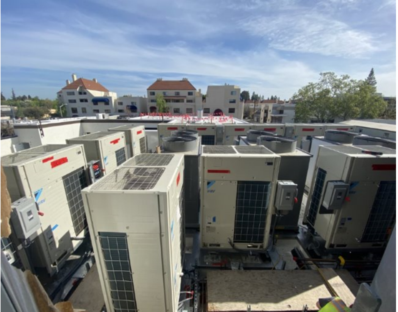
View of emergency Electrical Roof Unit Installation.
