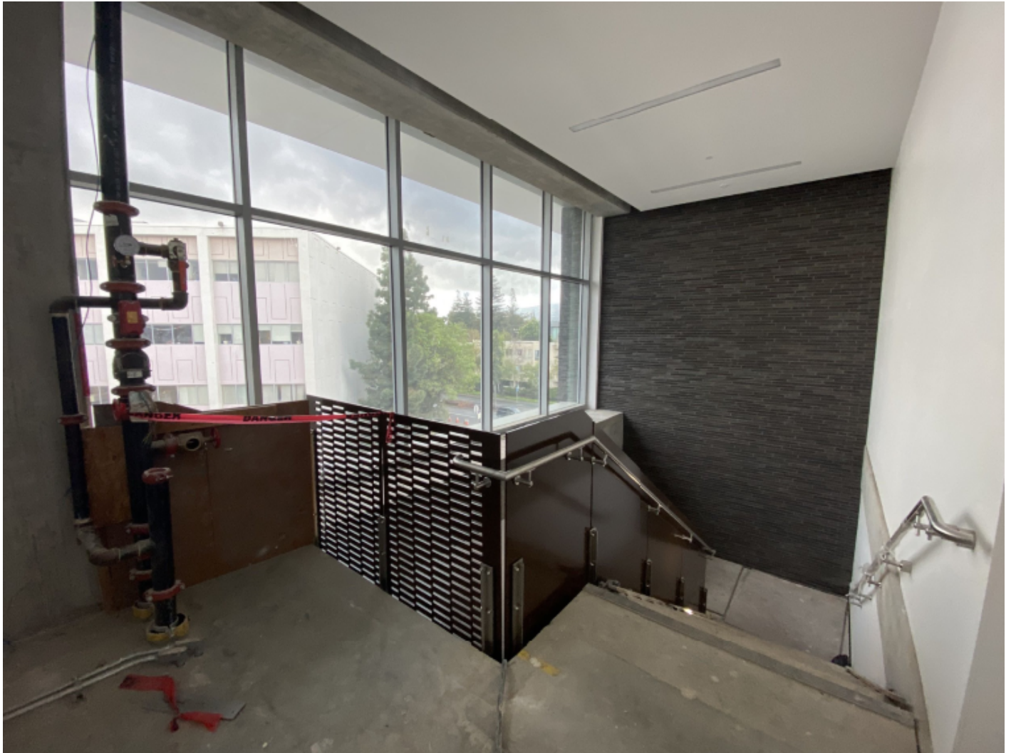
Stair rail installation.
