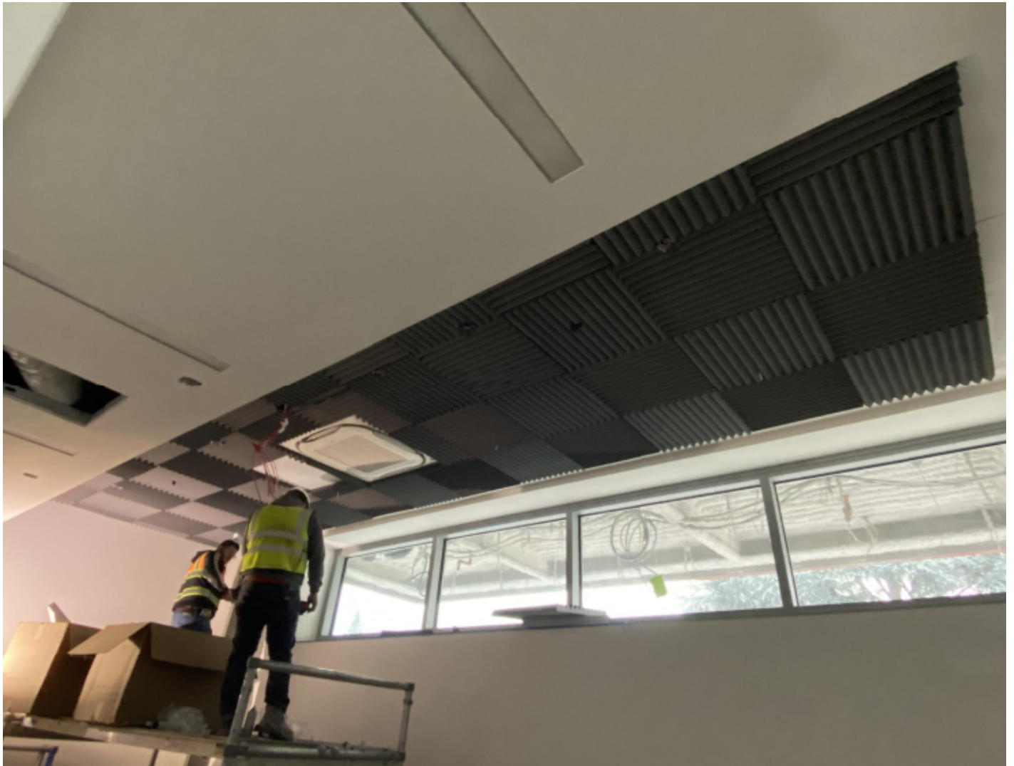
Ceiling installation L1.
