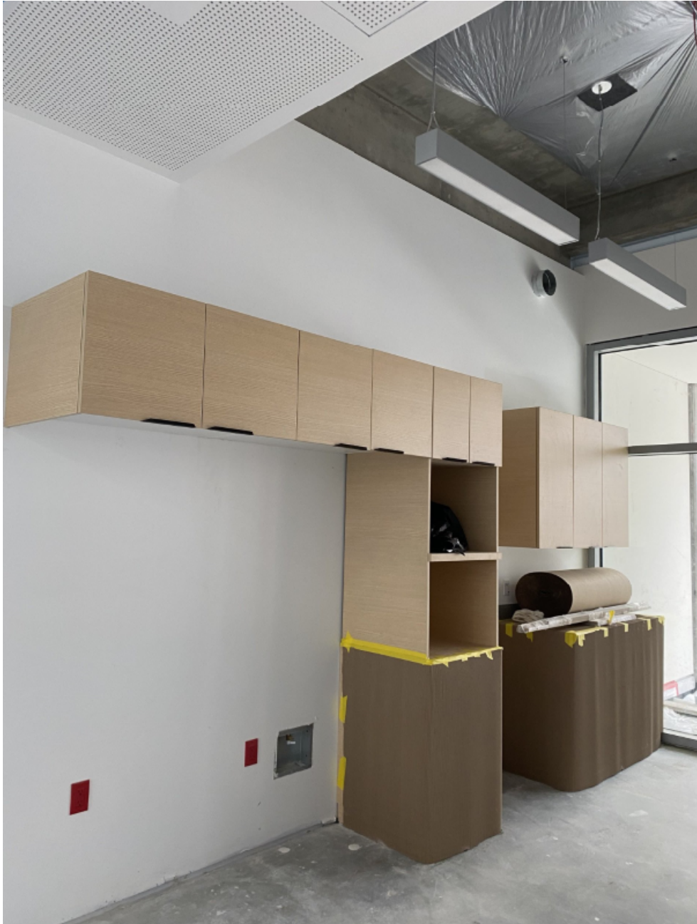
L2 Millwork installation.
