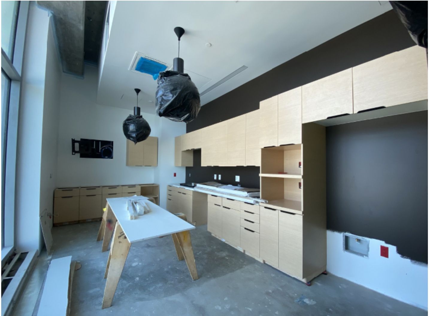
L3 kitchen millwork installation.
