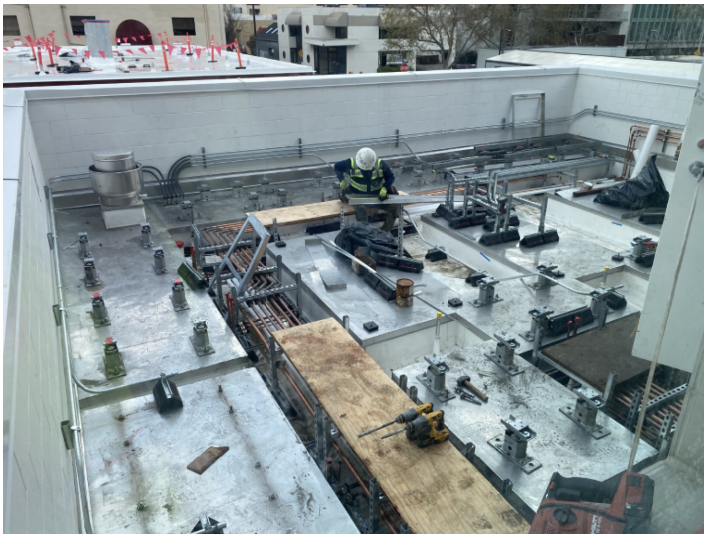
View of piping installation on Emergency electrical Room Roof.
