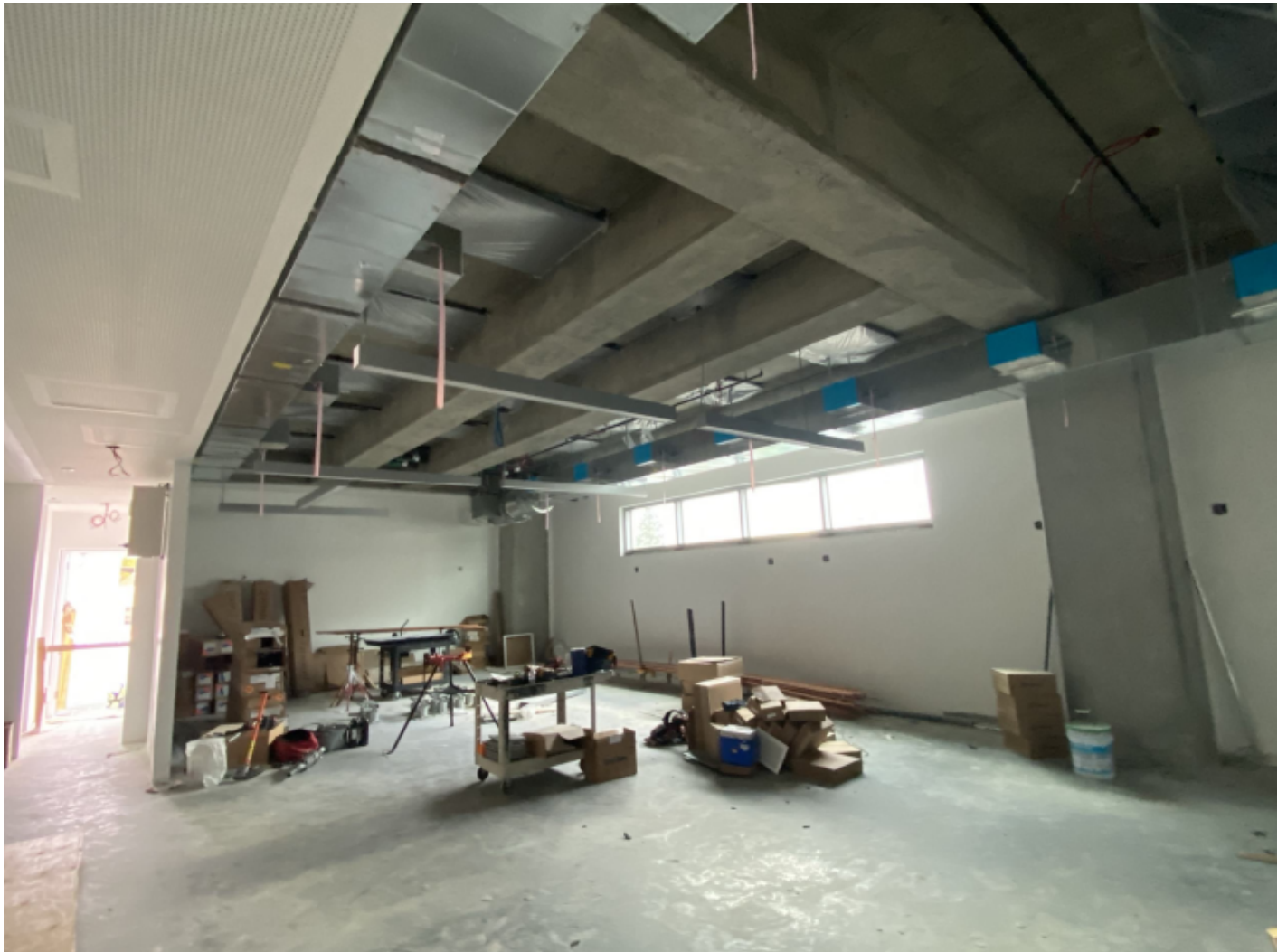
L2 Men's Locker Room.
