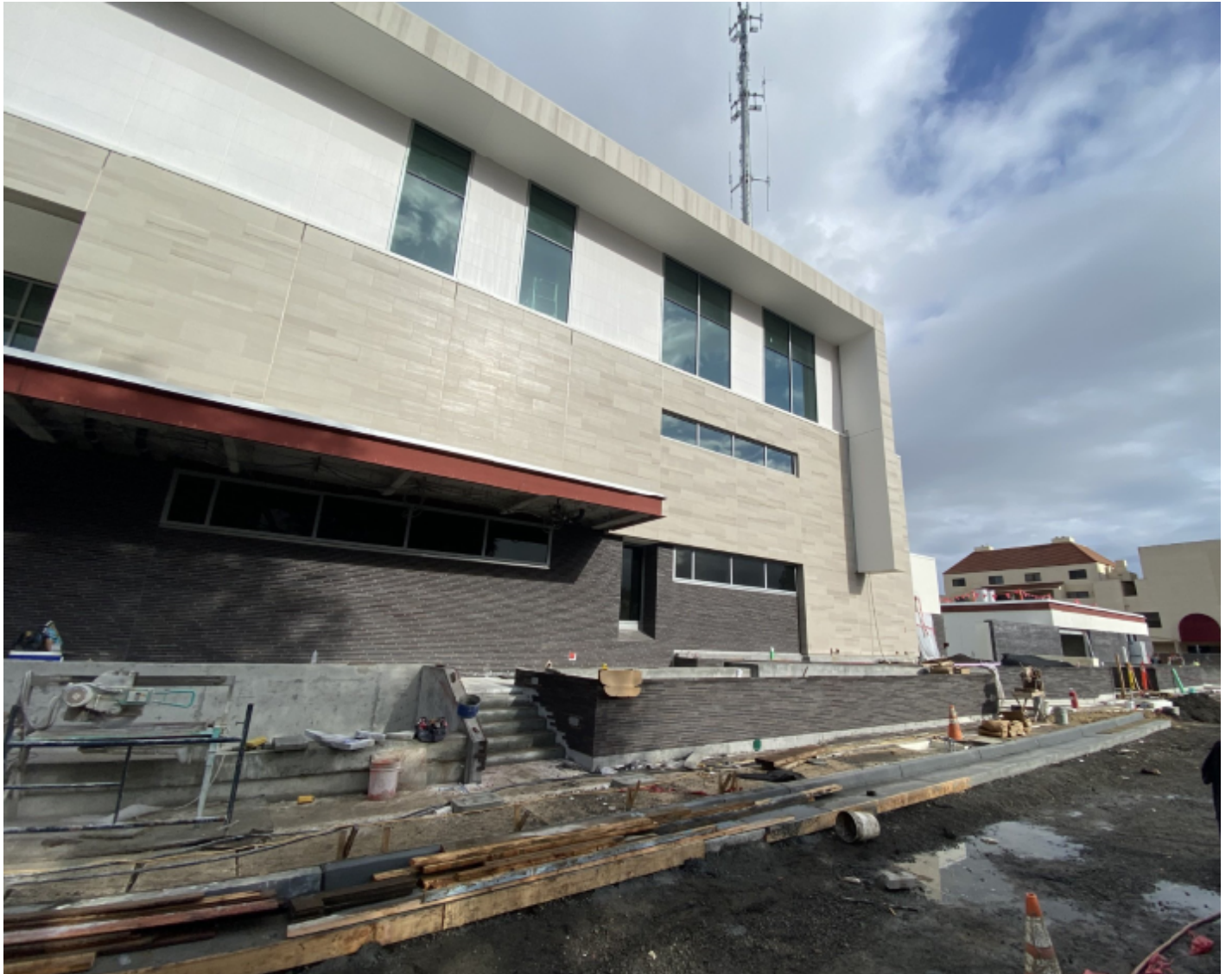
View of Sherman Ave. site concrete.
