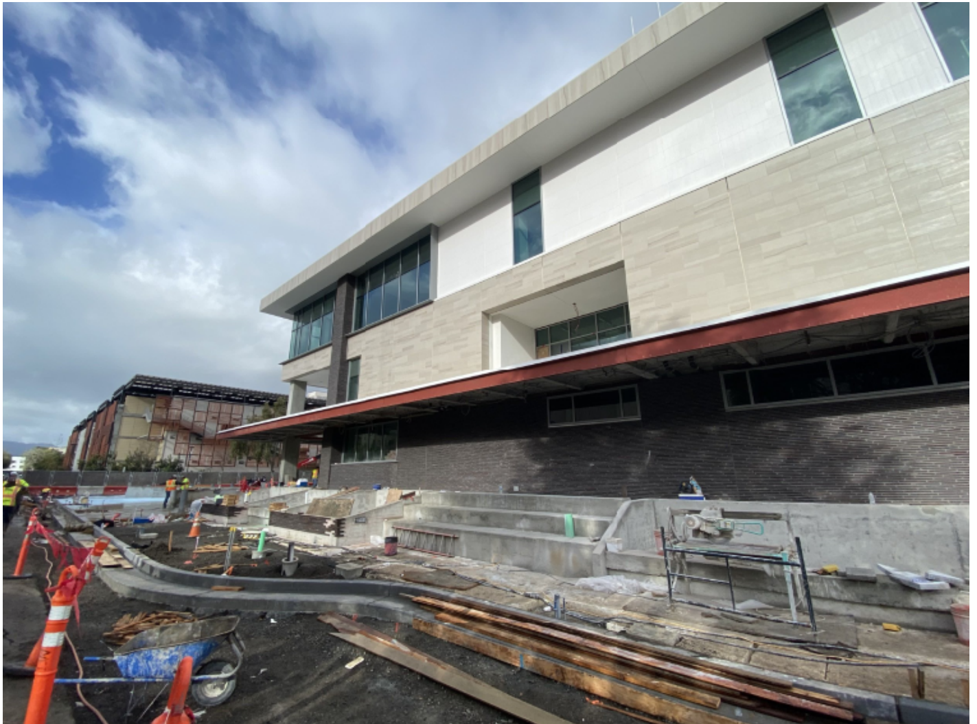
View of Sherman Ave. site concrete.
