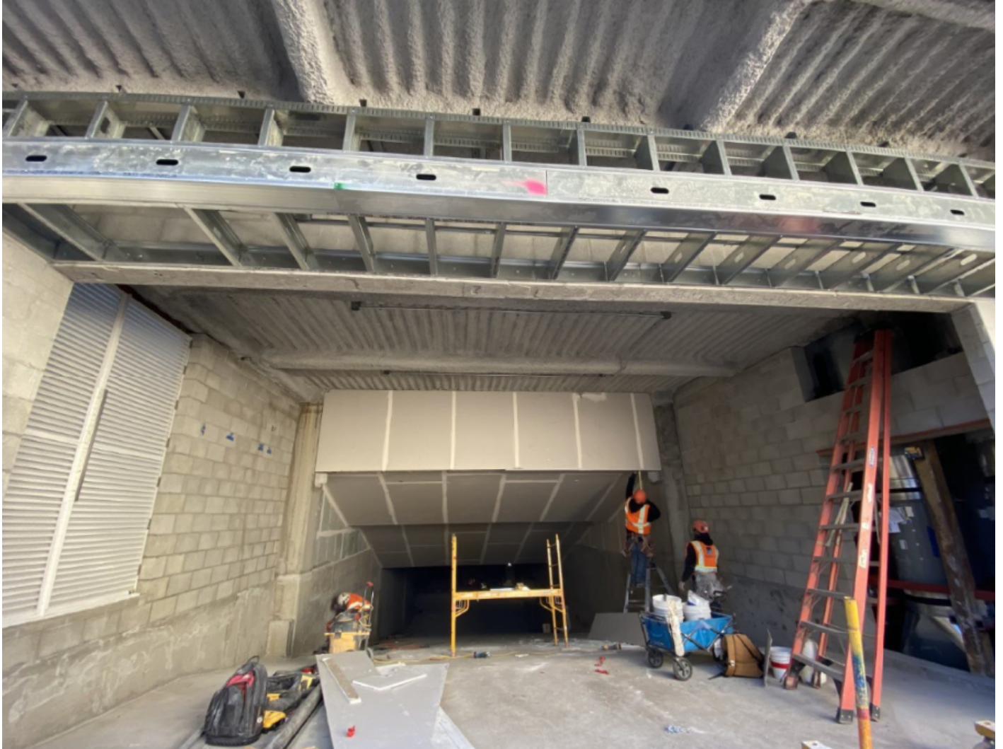
Garage access from Jacaranda.
