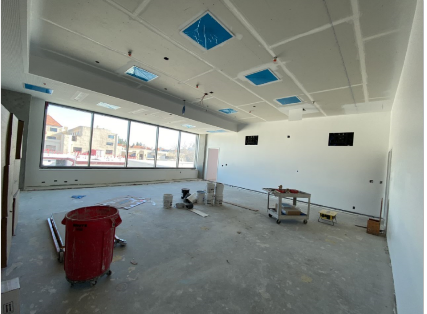
L3 Fitness Facility with windows installed.
