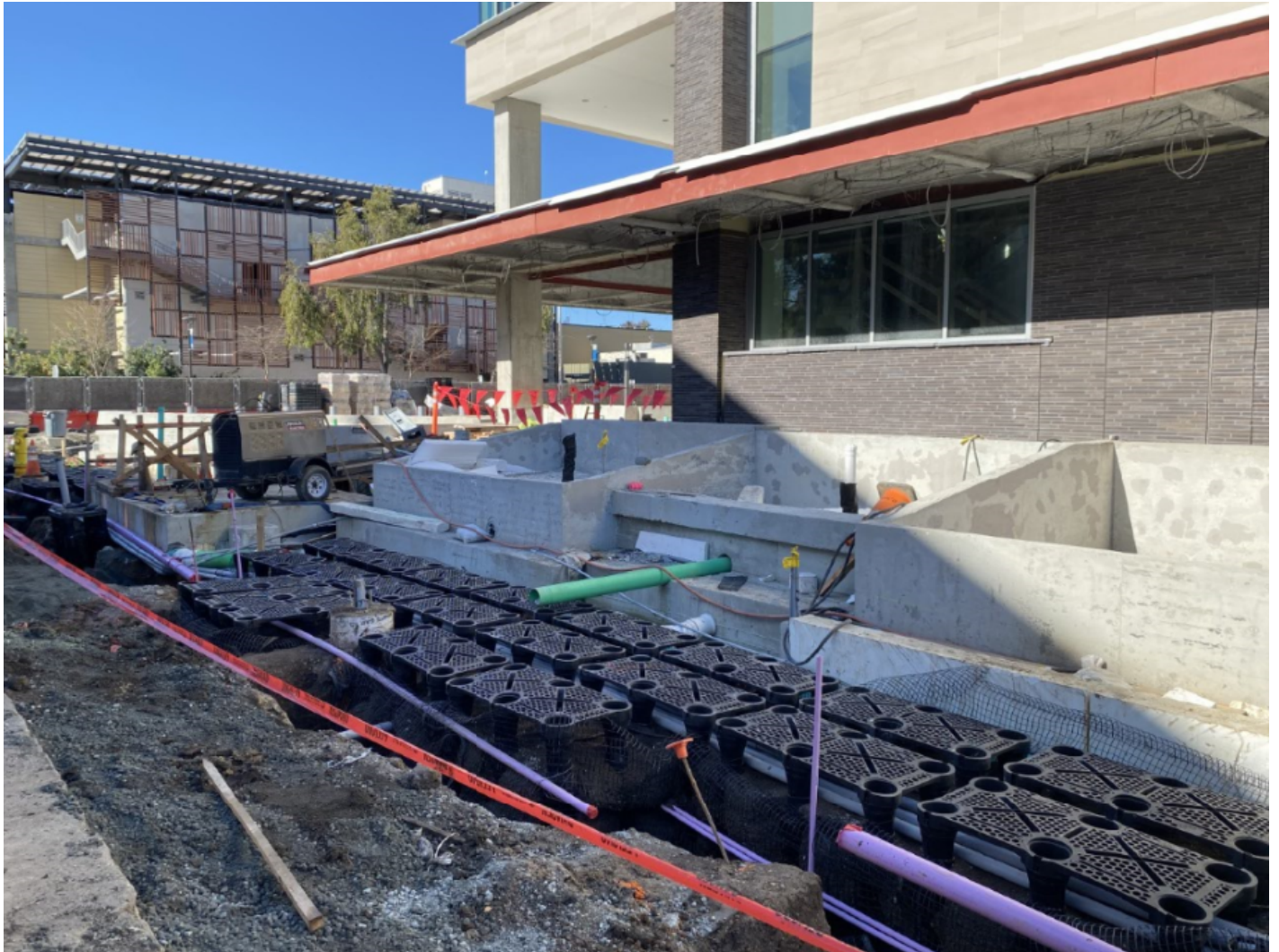
View of Sherman Ave. Soil Cell.
