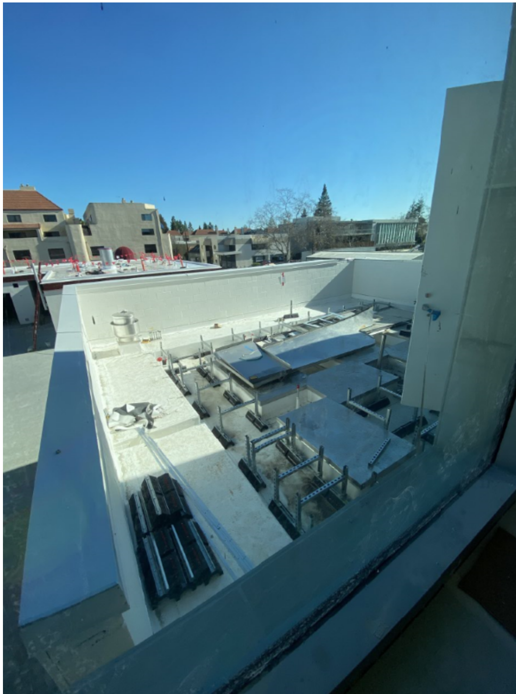
Electrical room roof pipe support installation.
