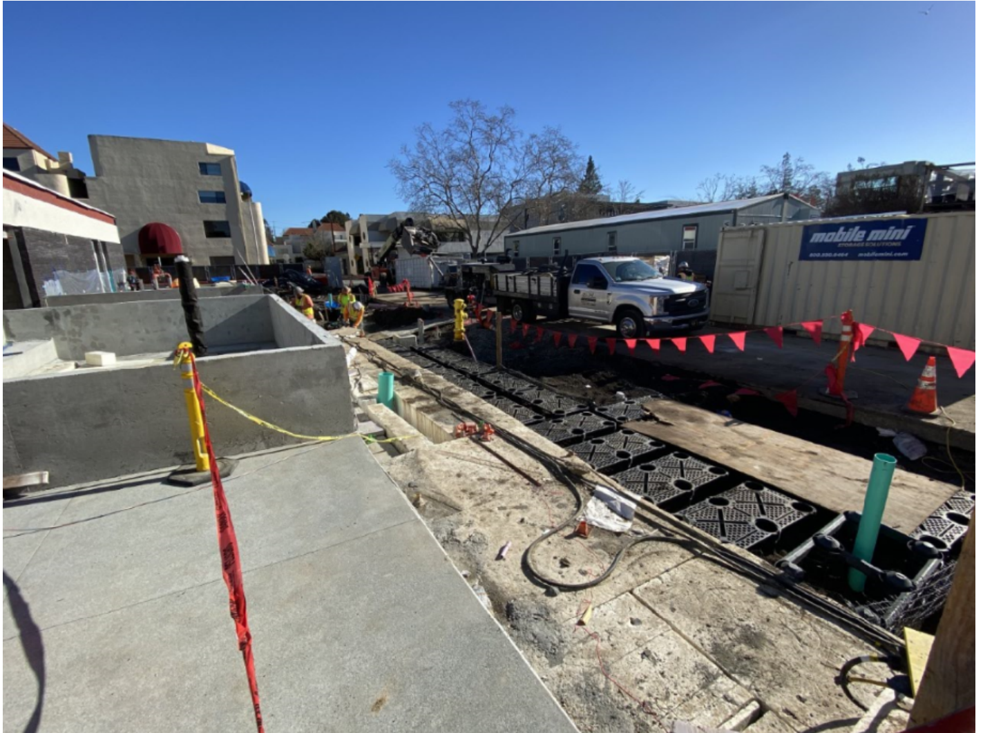
Soil Cell on Sherman Ave. East.
