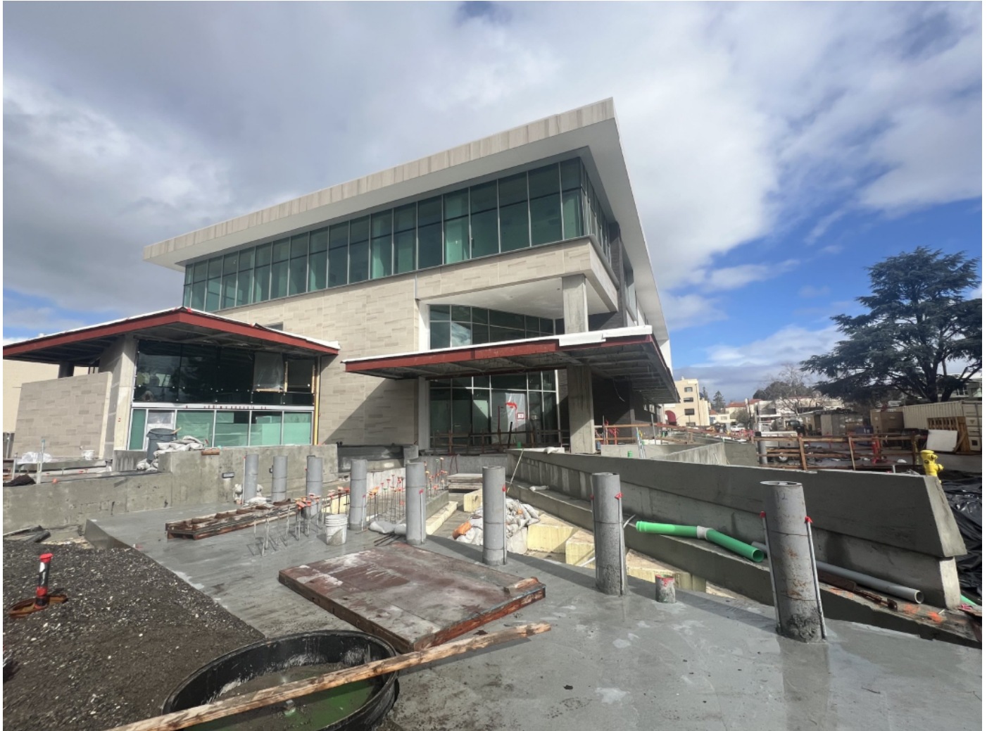
View of building entrance from Birch St.
