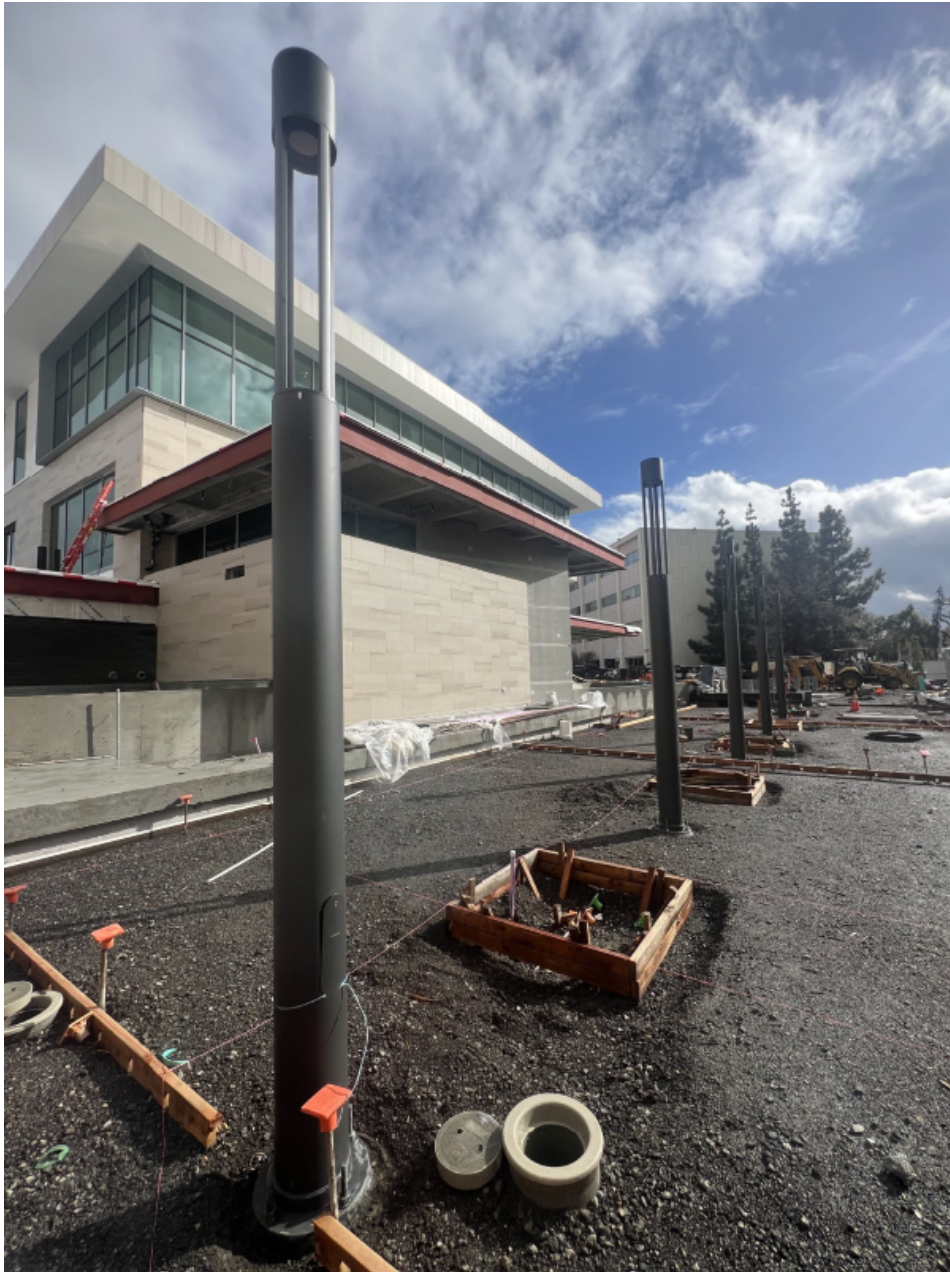
Birch St. flatwork and site lighting.
