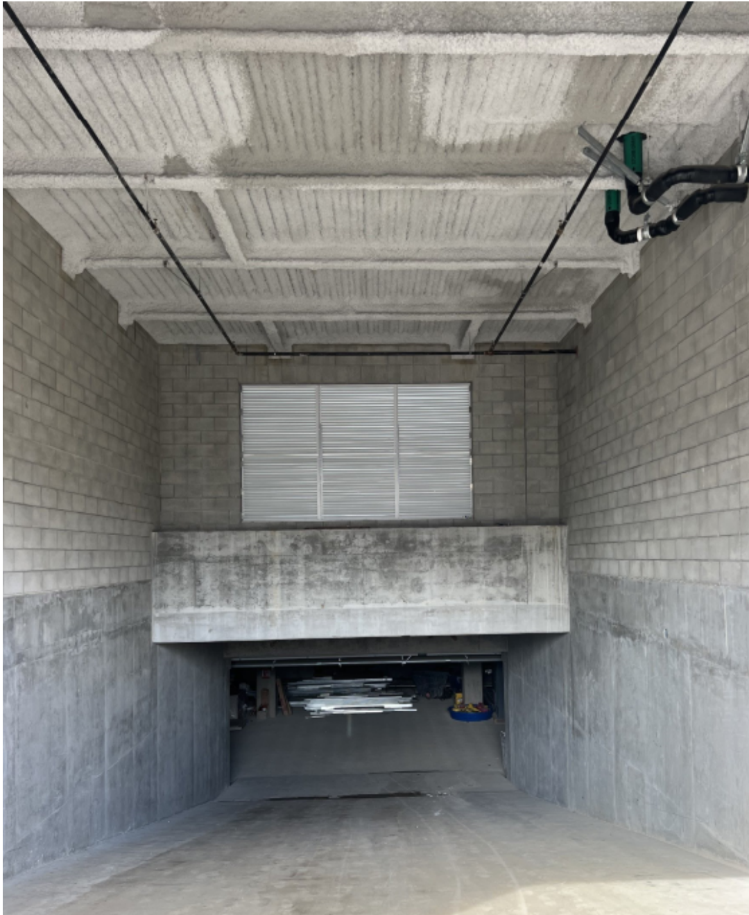
Garage ramp showing louver installation.
