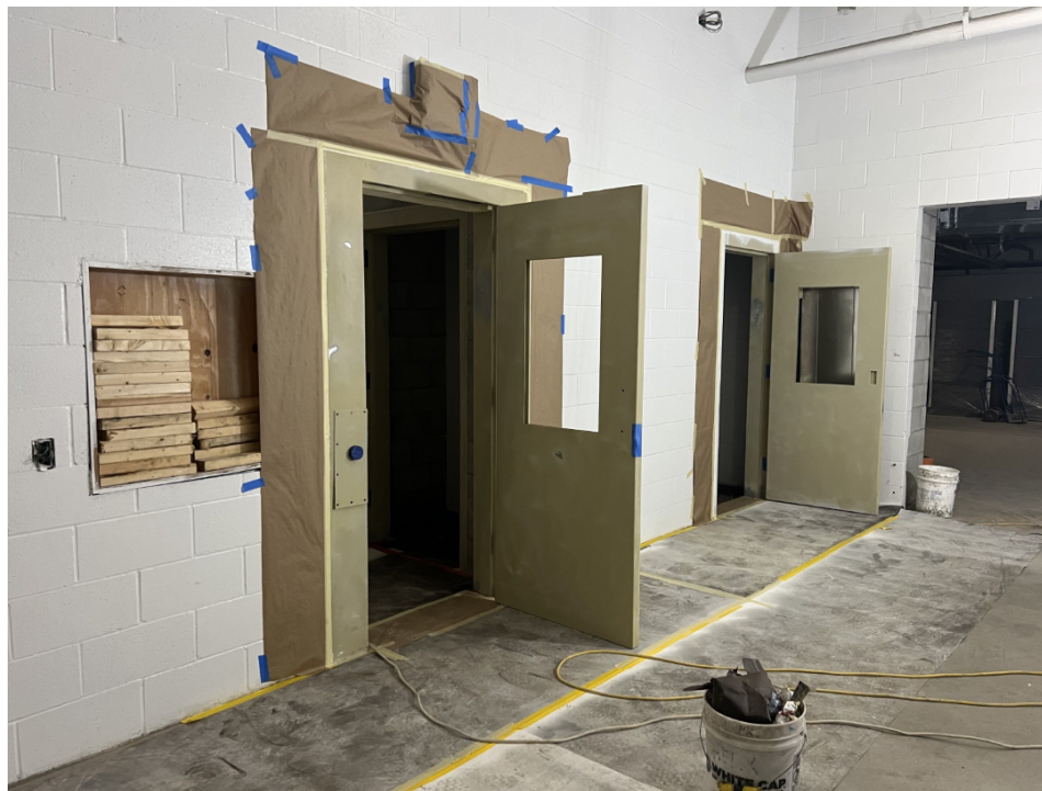
B1 detention entrance doors.
