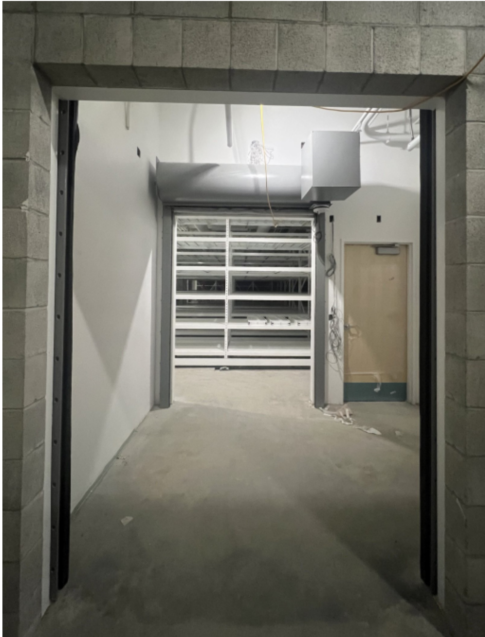
B1 coiling door installation.
