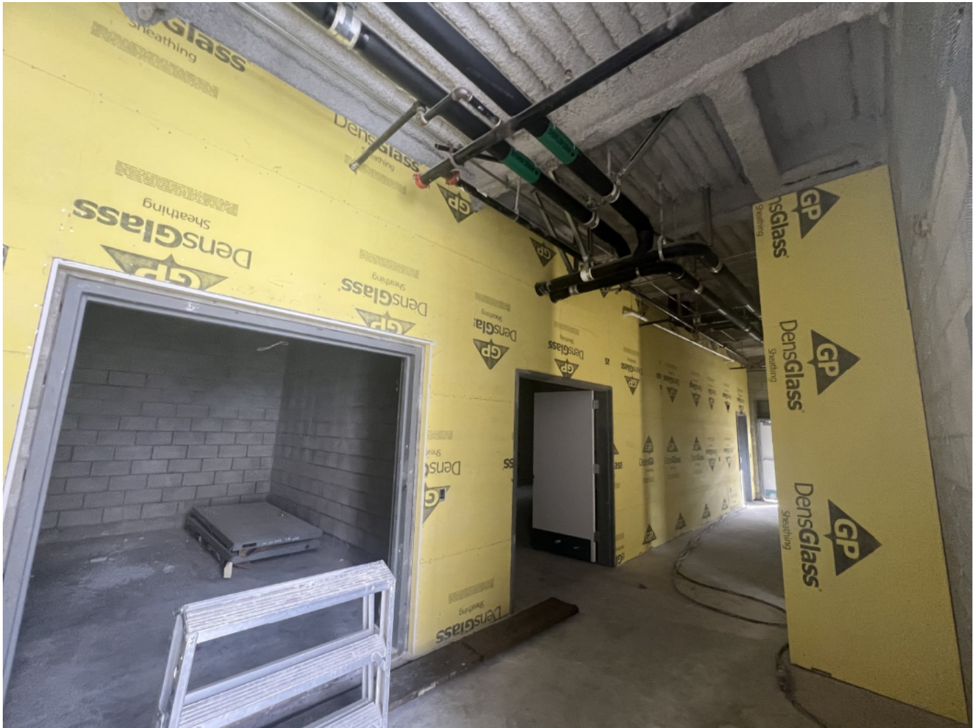
View of utility yard spaces.
