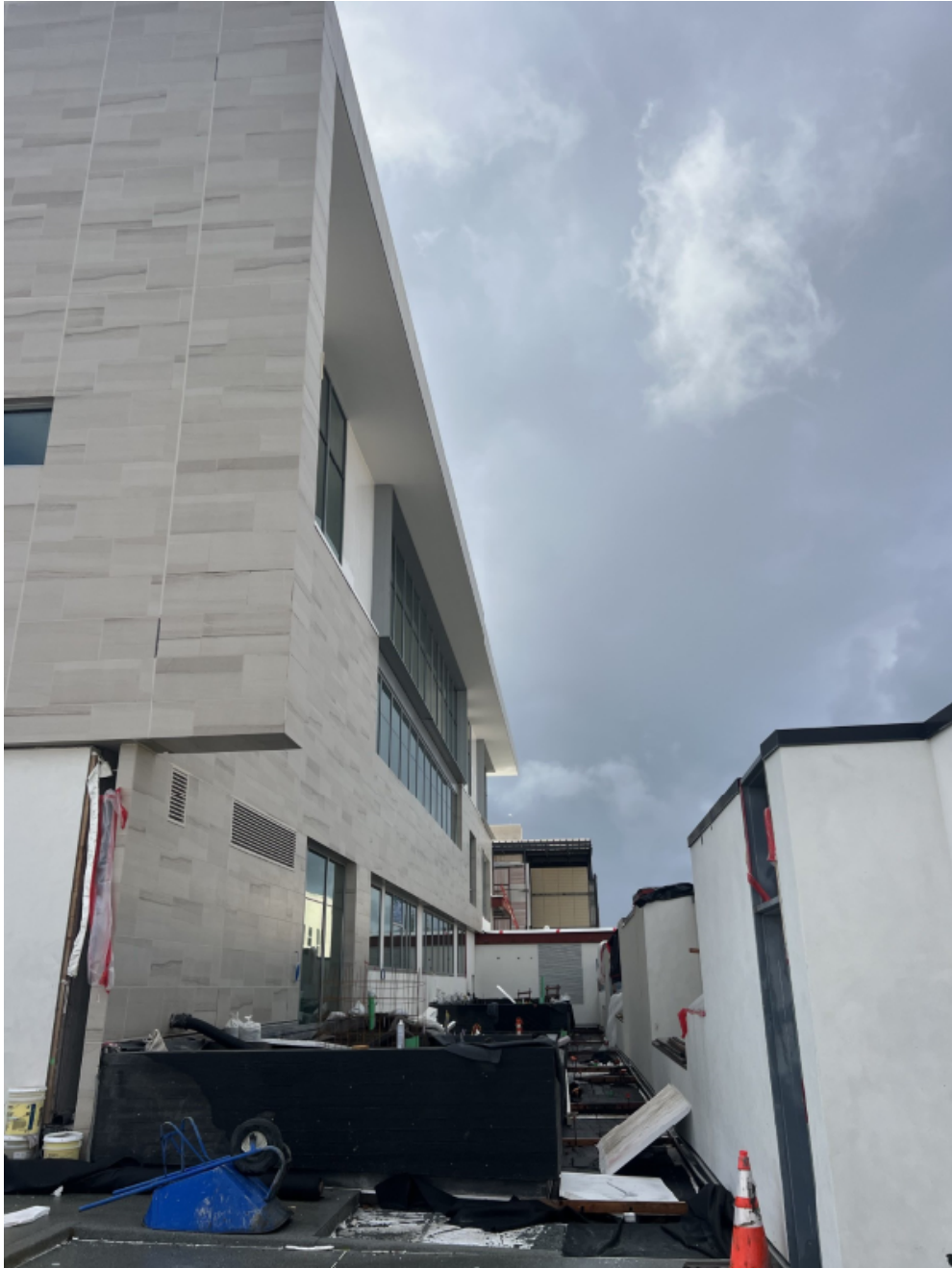
View of yard along Jacaranda Ln.
