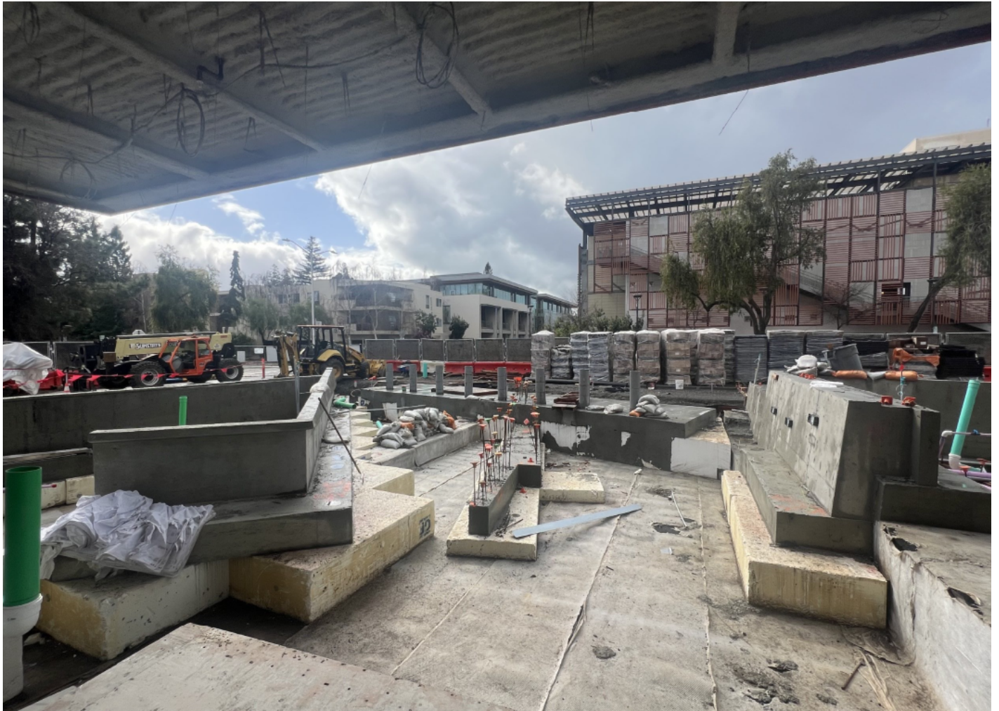
View of Plaza Entry from building storefront.
