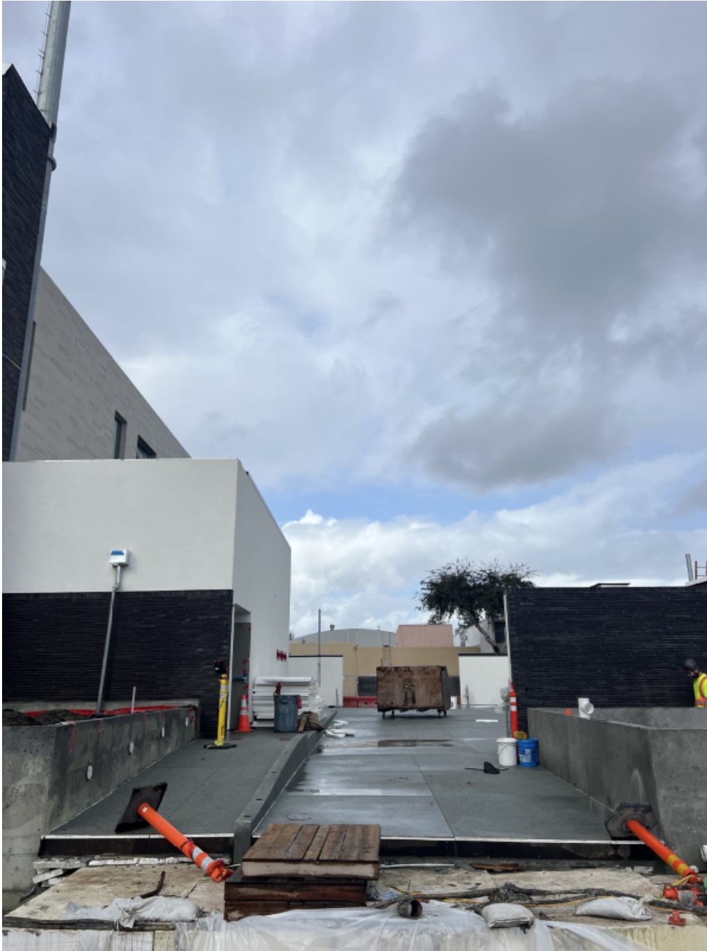
Utility yard entrance flatwork.
