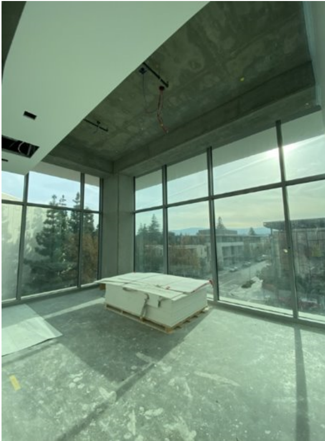
Police Chief and View of Atrium on L3.
