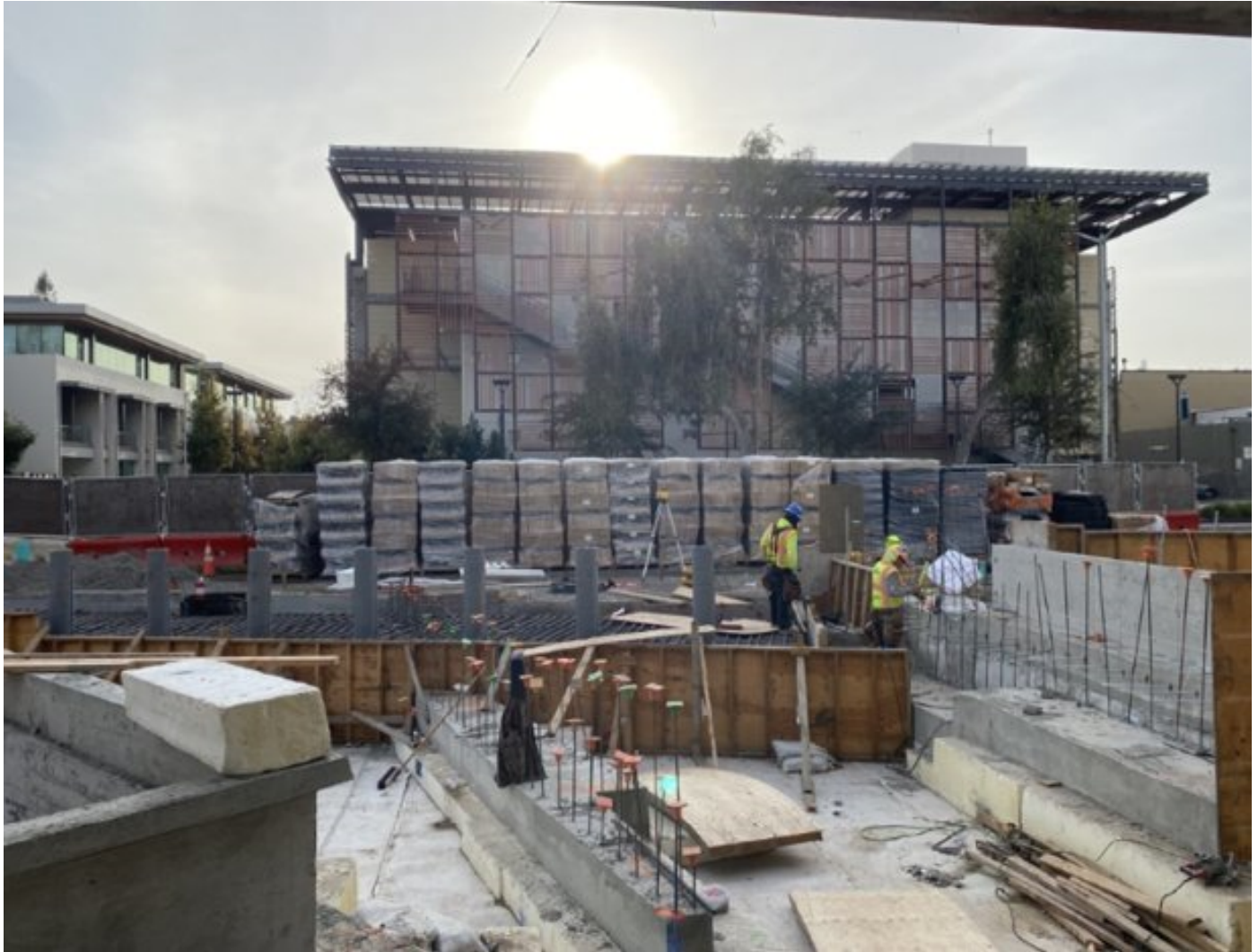
View of Plaza Formwork from Building Entrance.
