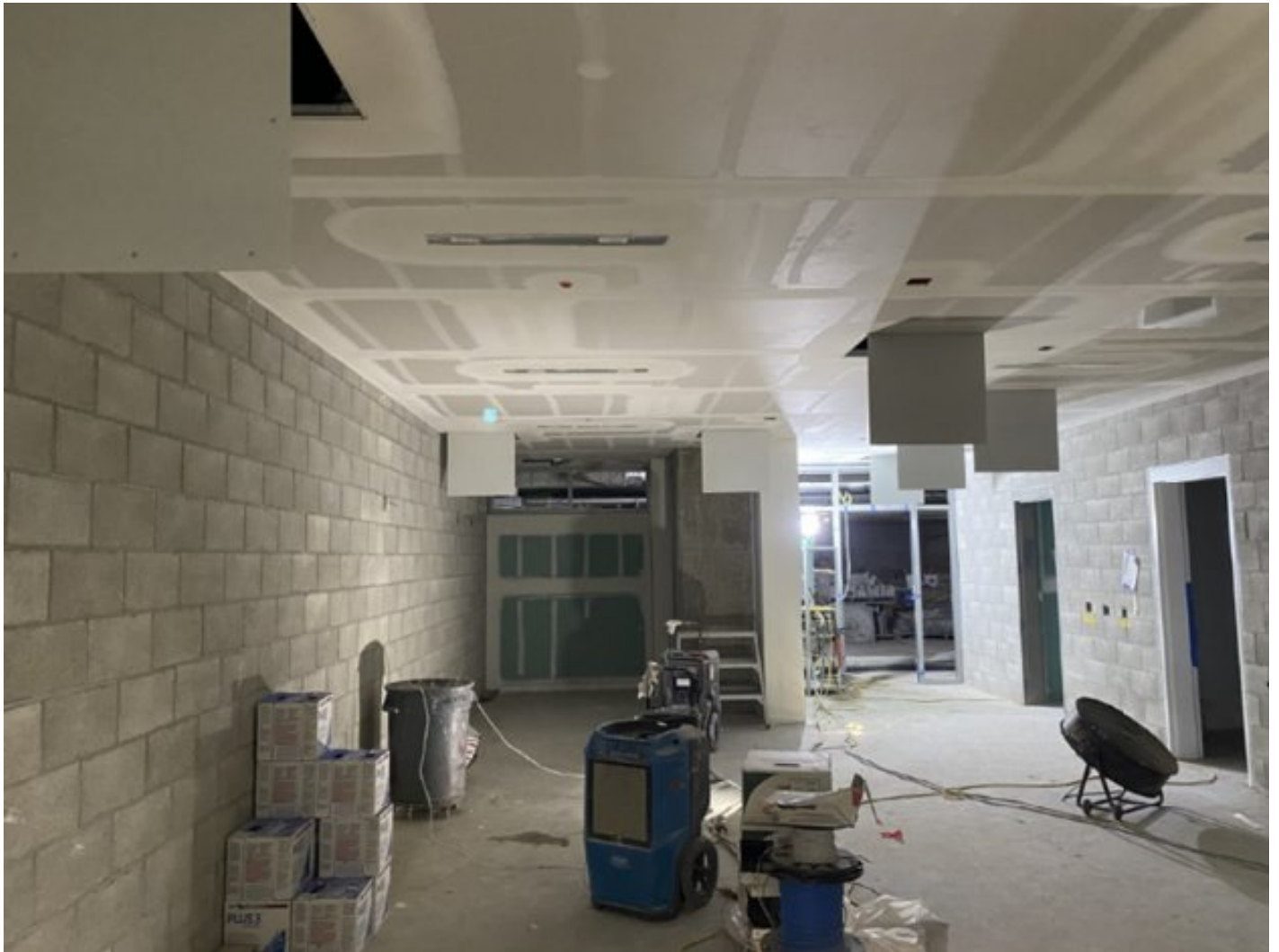
Entry Lobby on B1.
