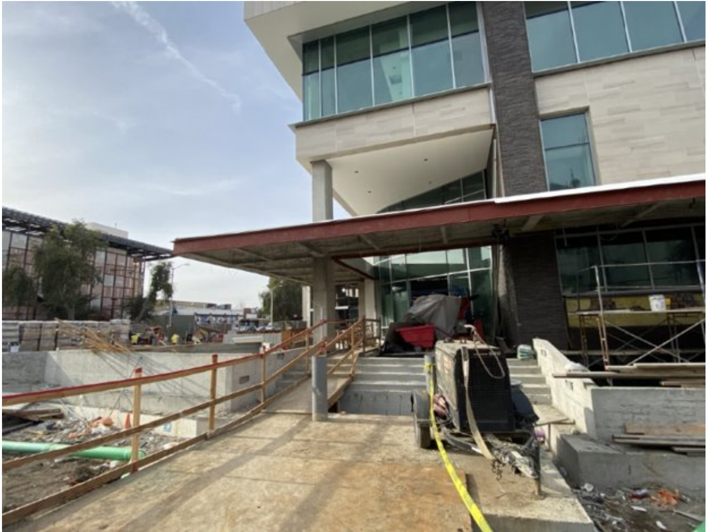
View of Plaza Entry from Sherman Ave.
