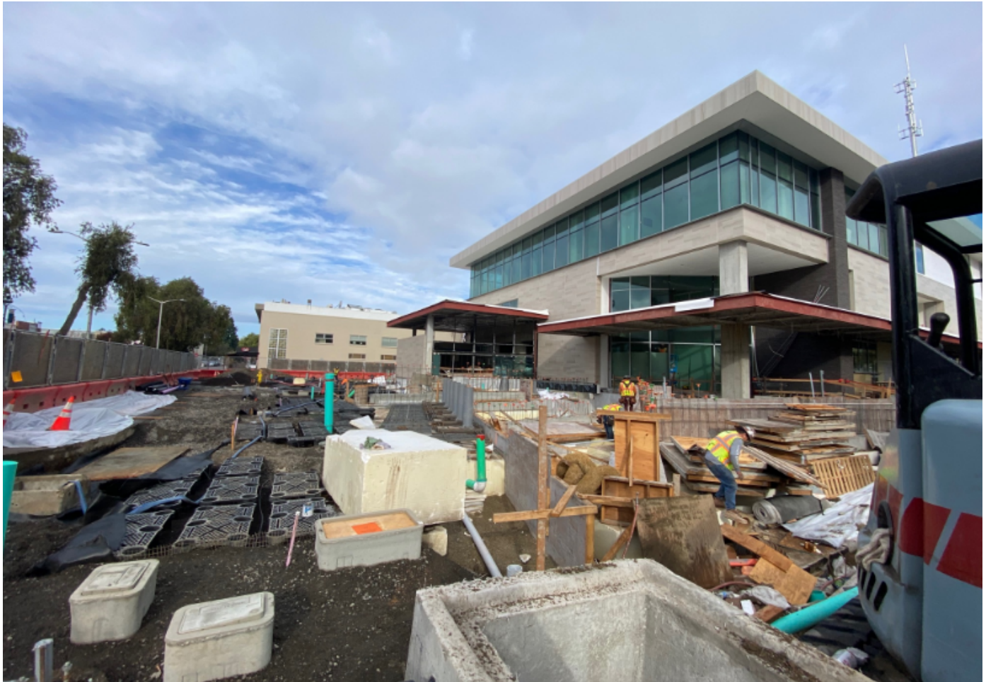
Birch St. Site Work and Silva Cell Install.
