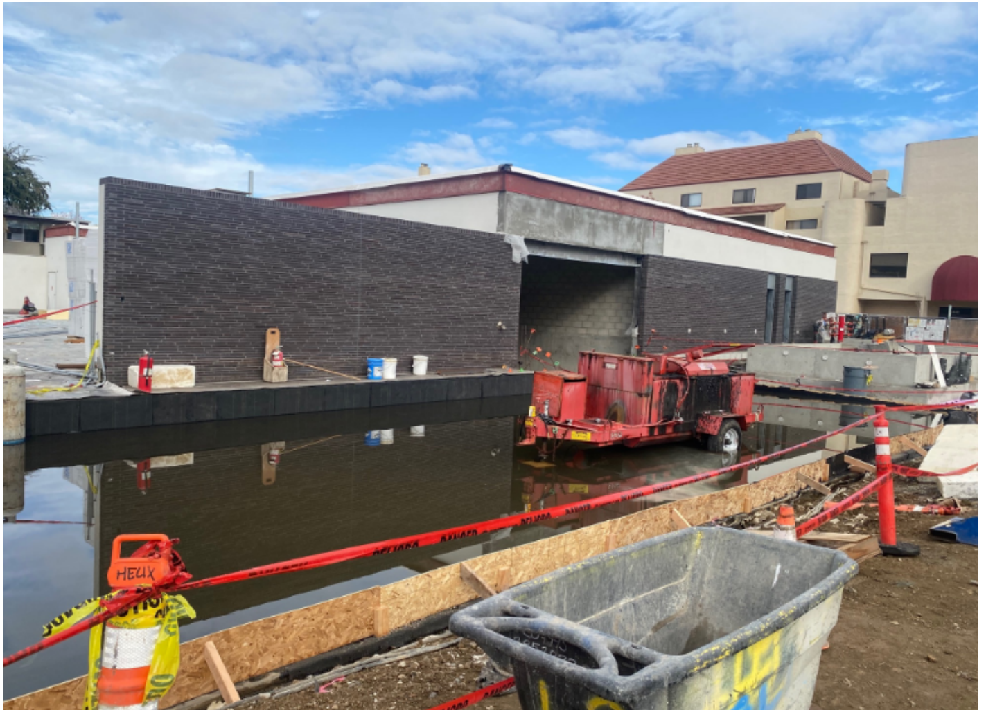
Flood testing and site work on Sherman Ave.
