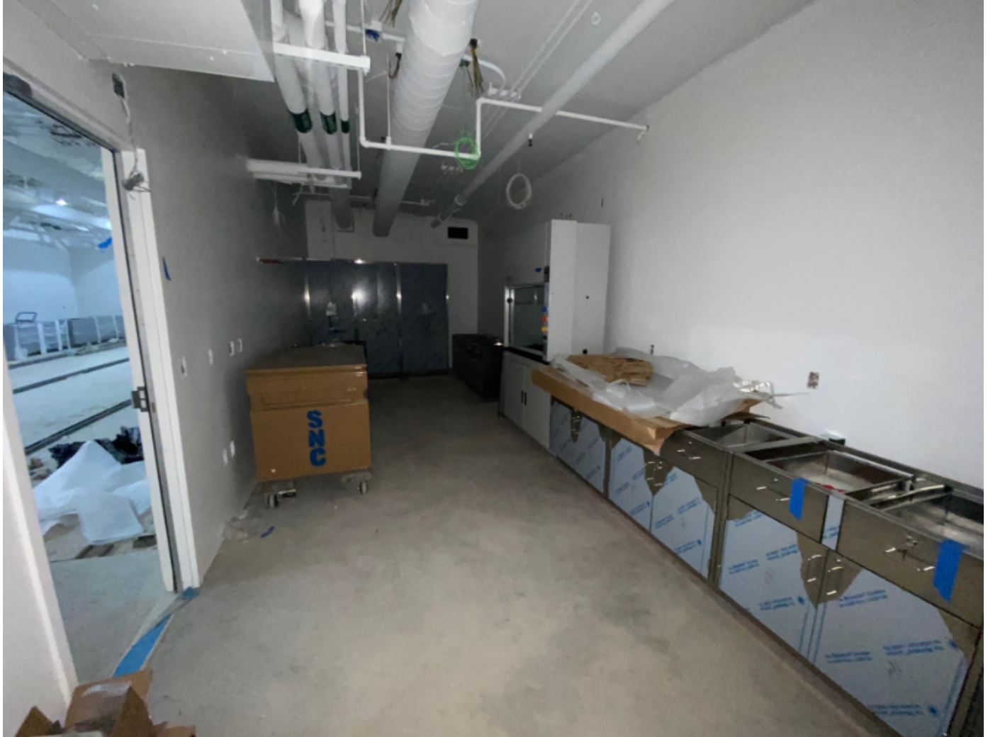
Casework installation on B1.
