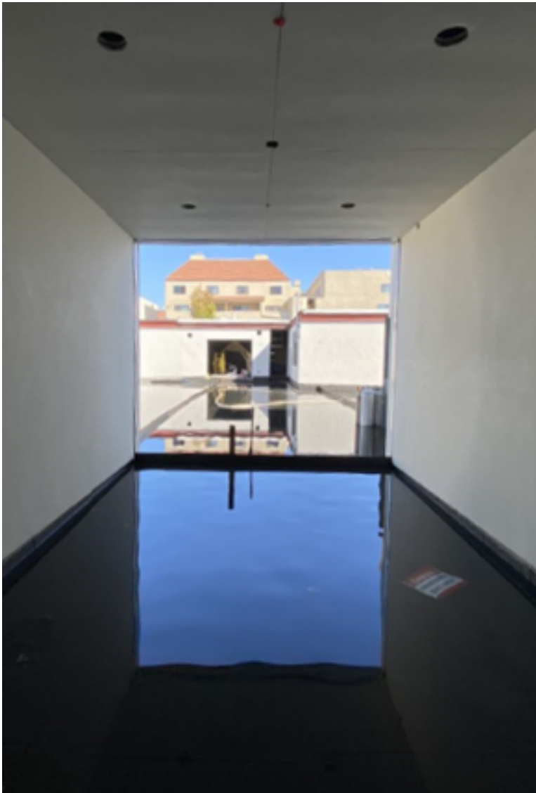
Utility Yard flood testing.
