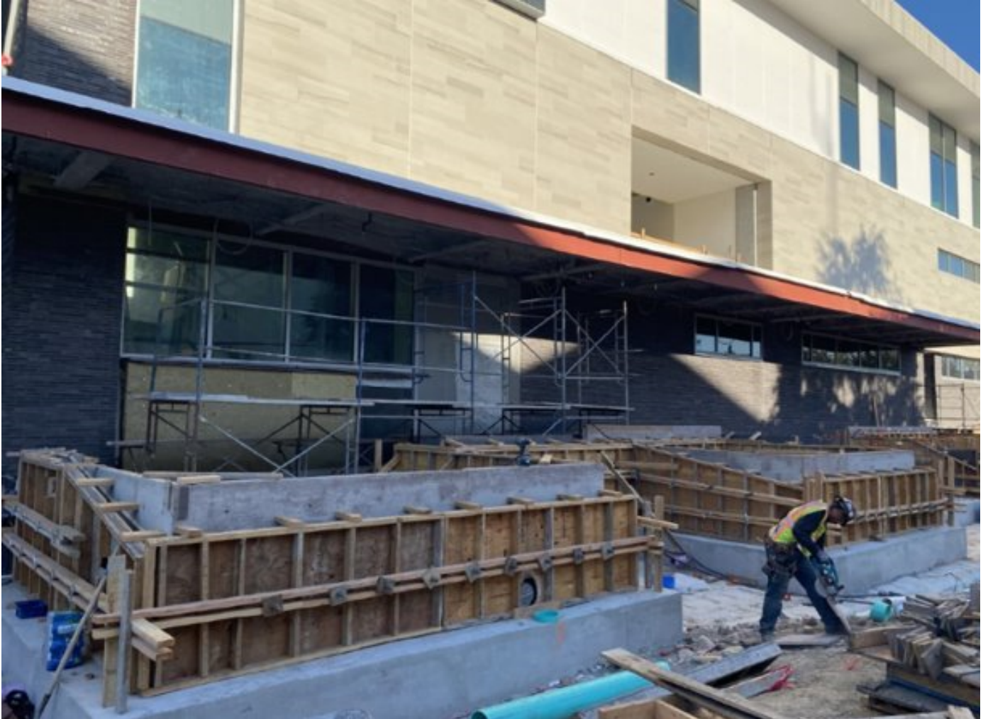
View of site concrete formwork on Sherman Ave.
