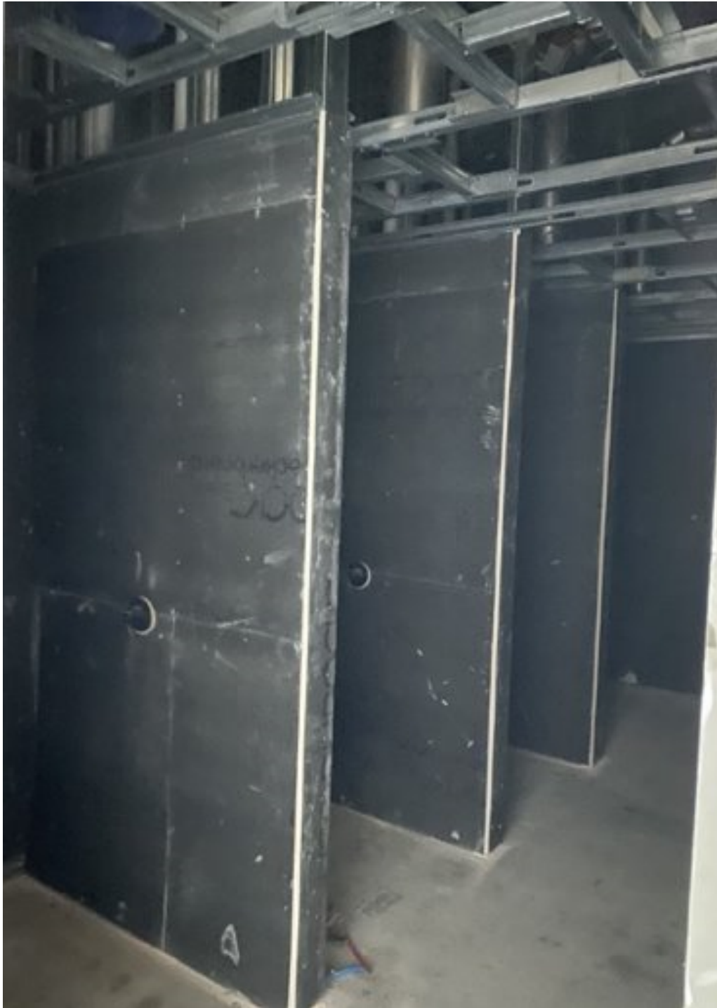
Bathroom stall installation.
