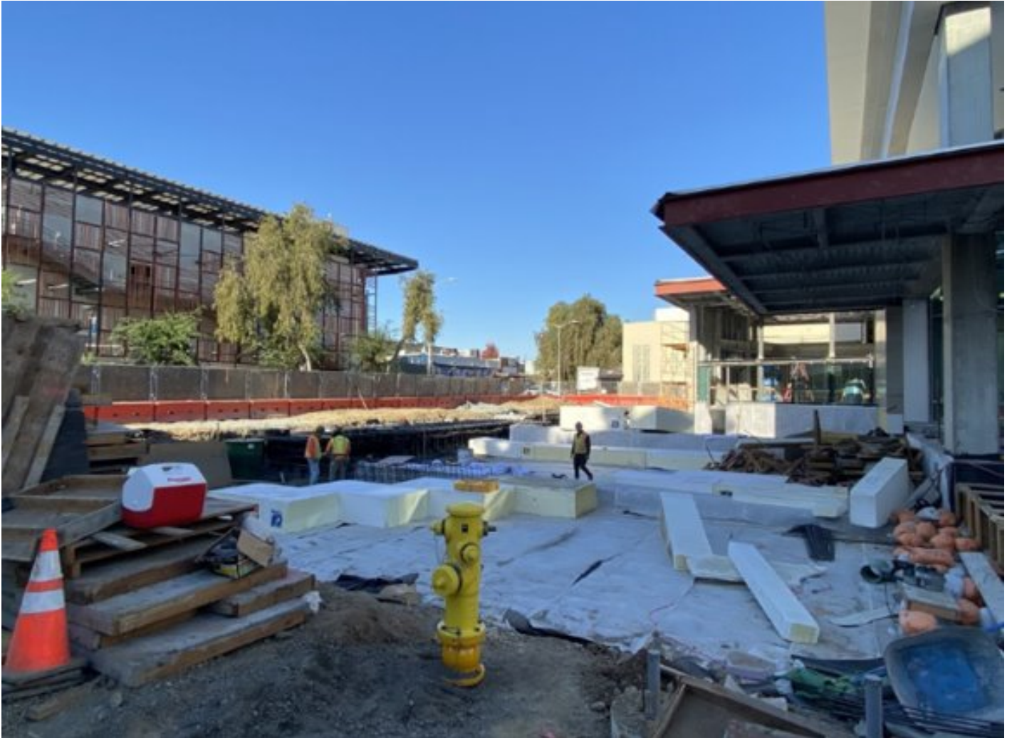
View of public entry waterproofing and soil cell.
