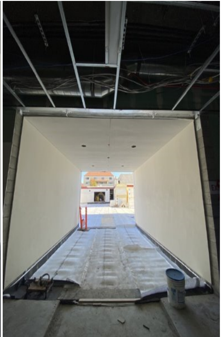
Utility Yard waterproofing.
