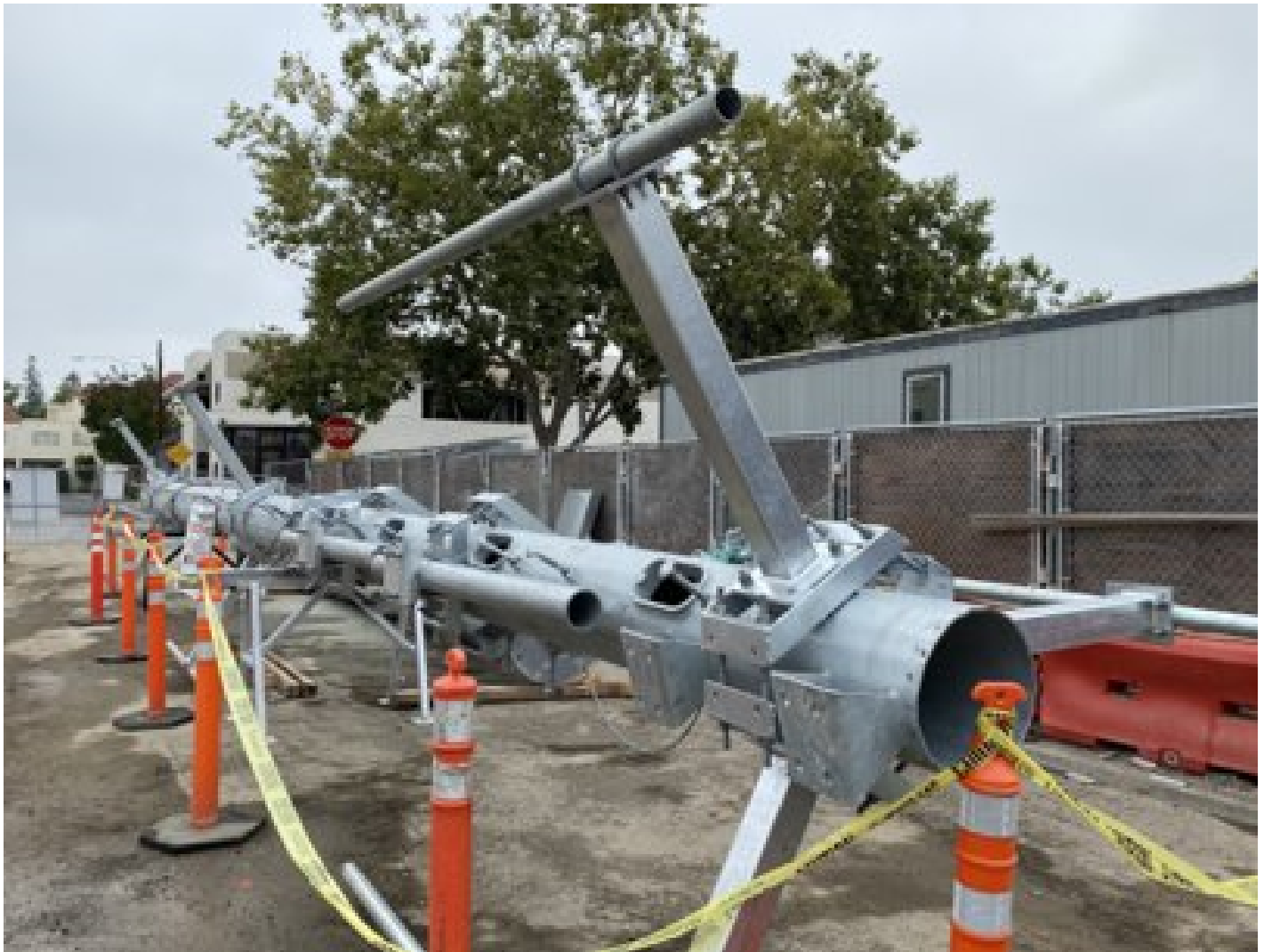
Monopole Tower delivered.
