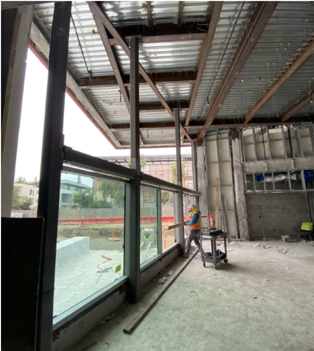
Glazing installation in Multi-Purpose Room.
