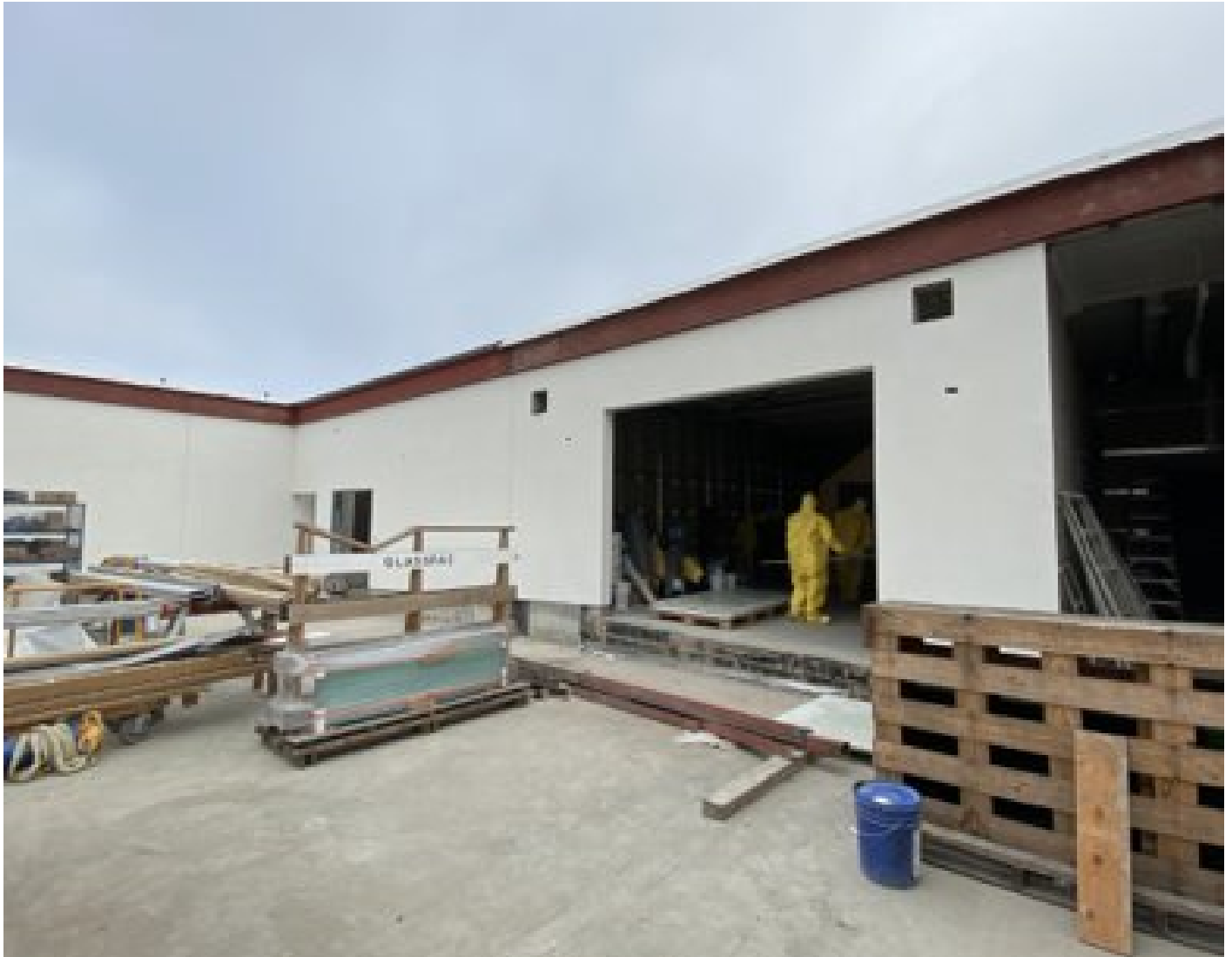
View of plaster in Utility Yard.
