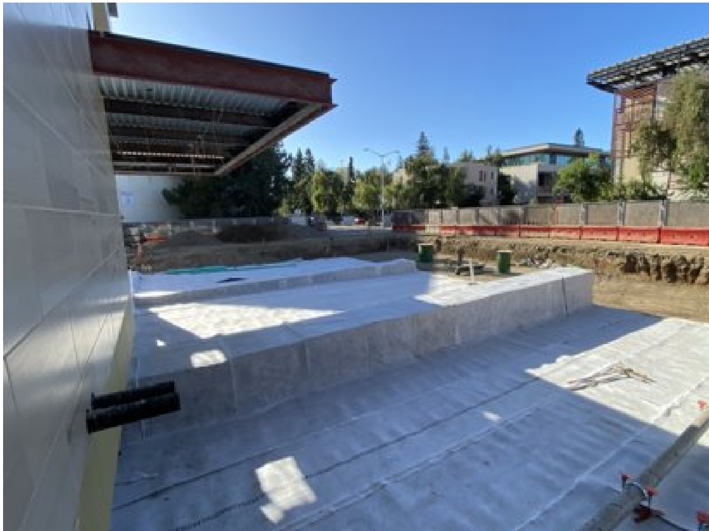
View of waterproofing from Multi-Purpose Room.
