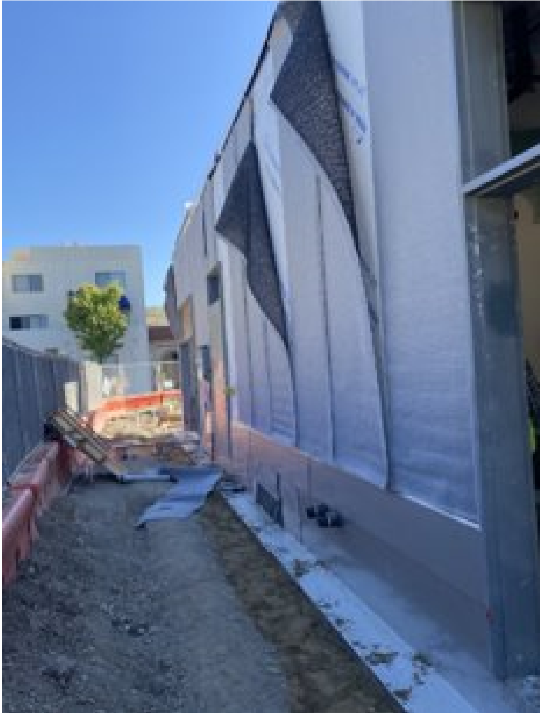
View of utility yard waterproofing from Jacaranda Rd.
