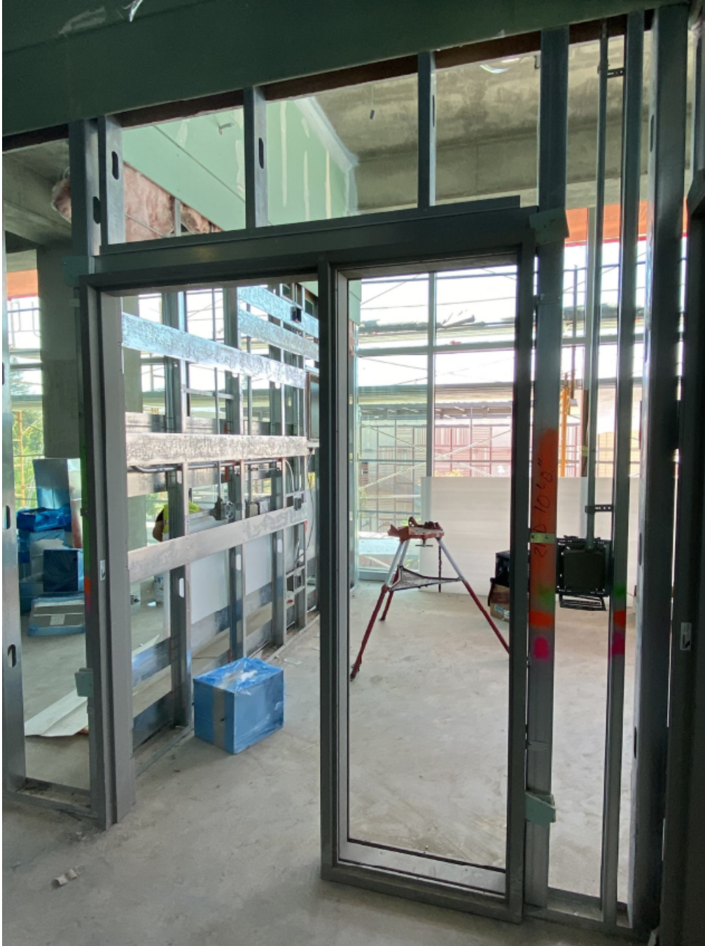
Door frame installation 3 rd Floor.
