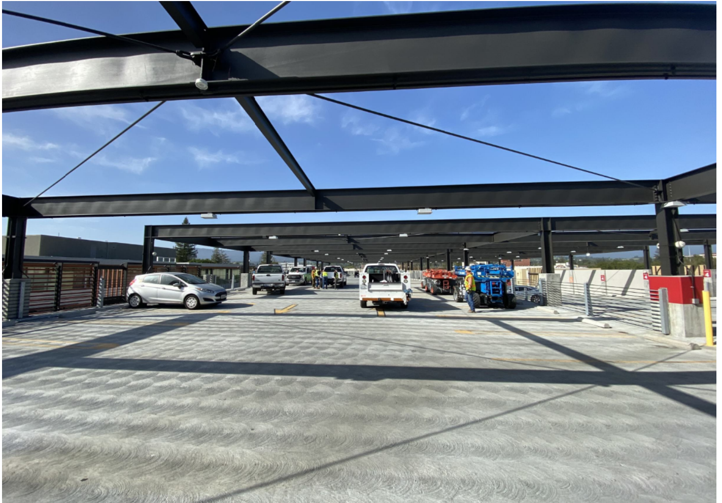
View of PV Mobilization Fourth Floor.
