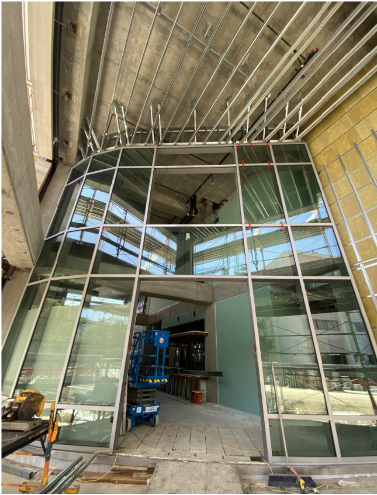
View of lobby from outside.
