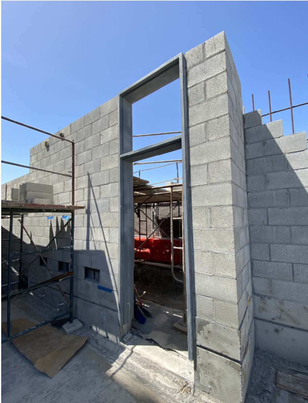
View of CMU on Jacaranda.
