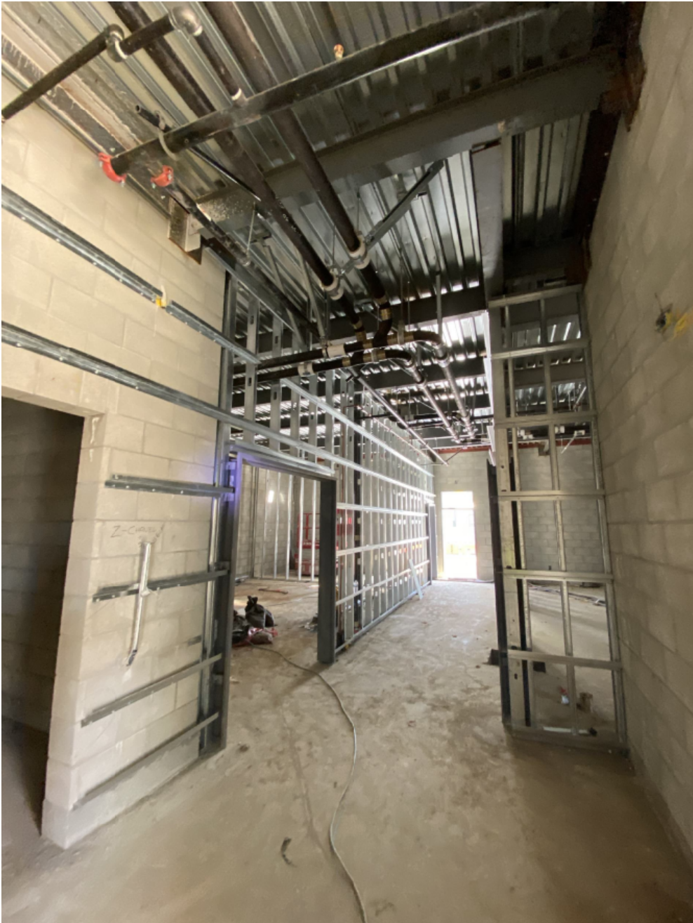
Utility Yard Framing.
