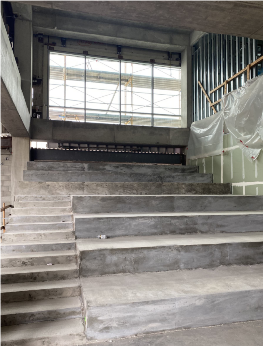
Lobby bleachers poured and cured.
