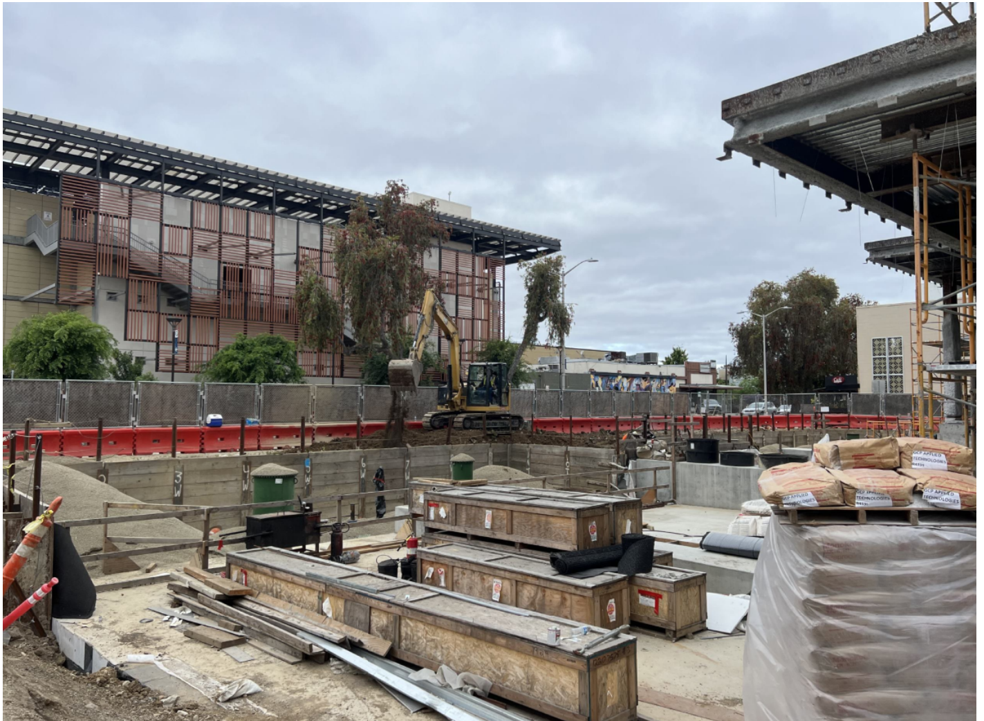
View of Fire and Water Tank Backfill on Birch.
