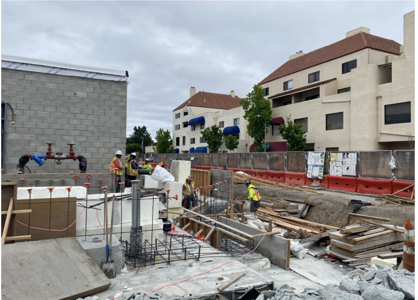
Site Retaining wall installation.
