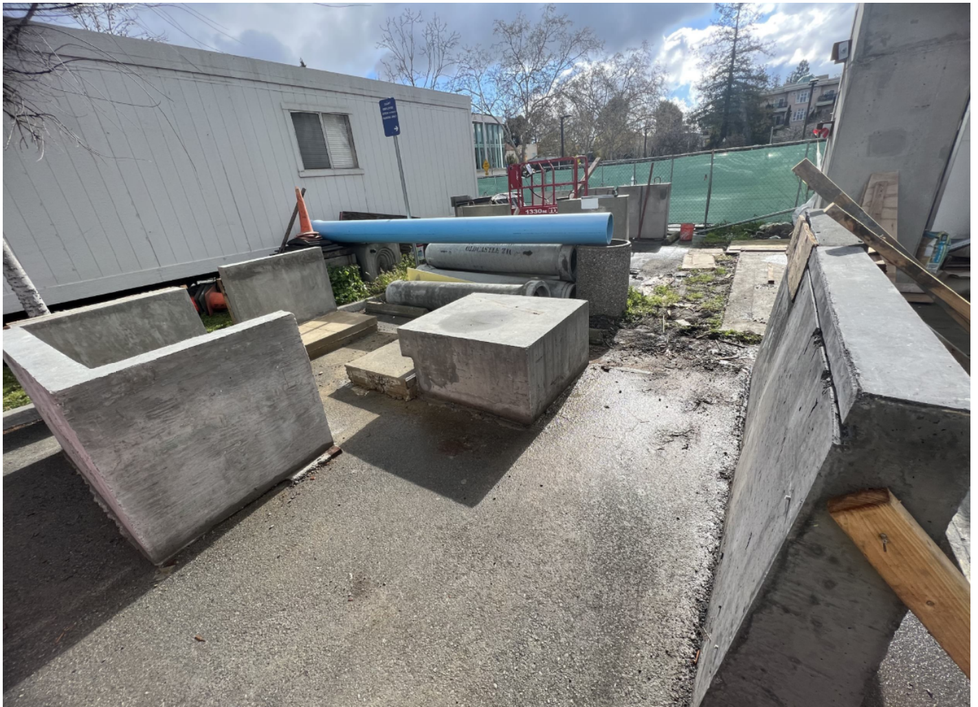
View of site work mock-up.
