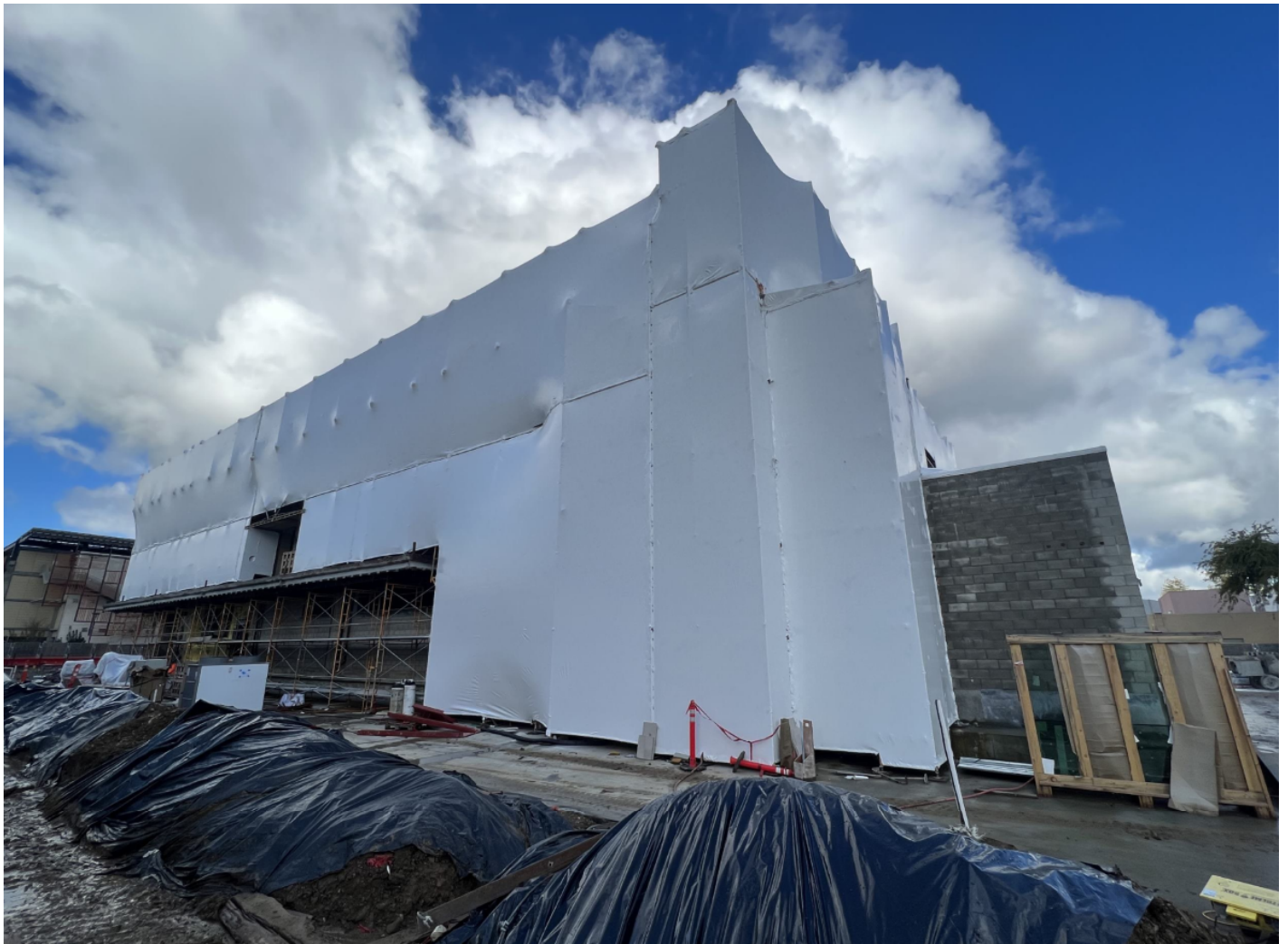
View from South elevation.
