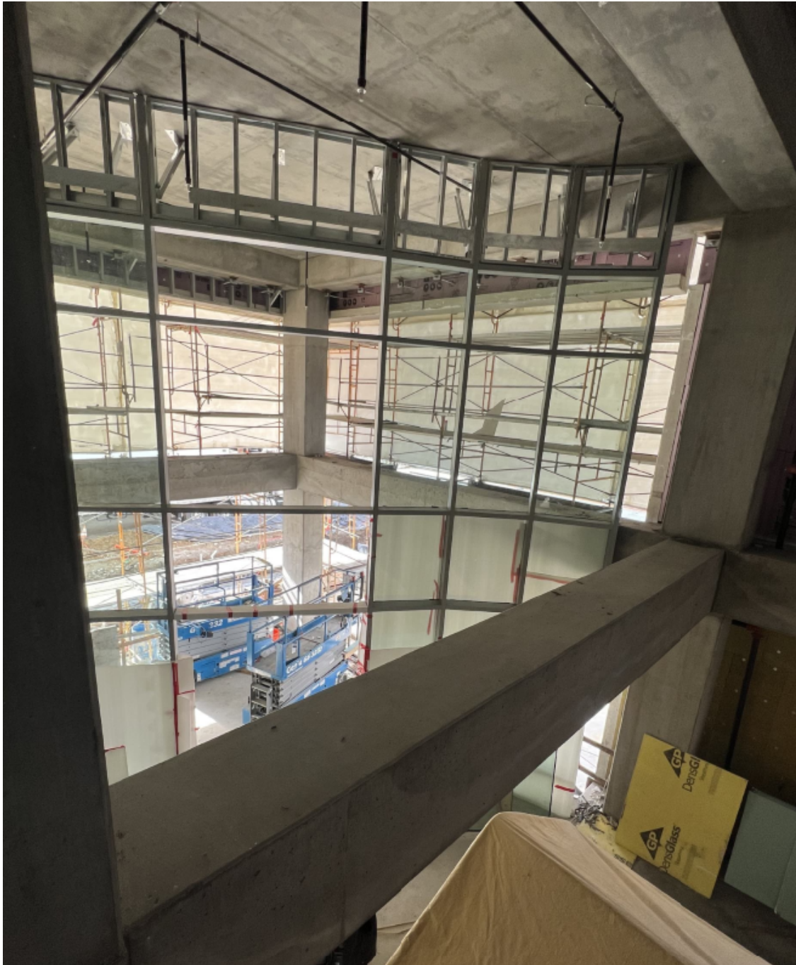
View of lobby from level 2.
