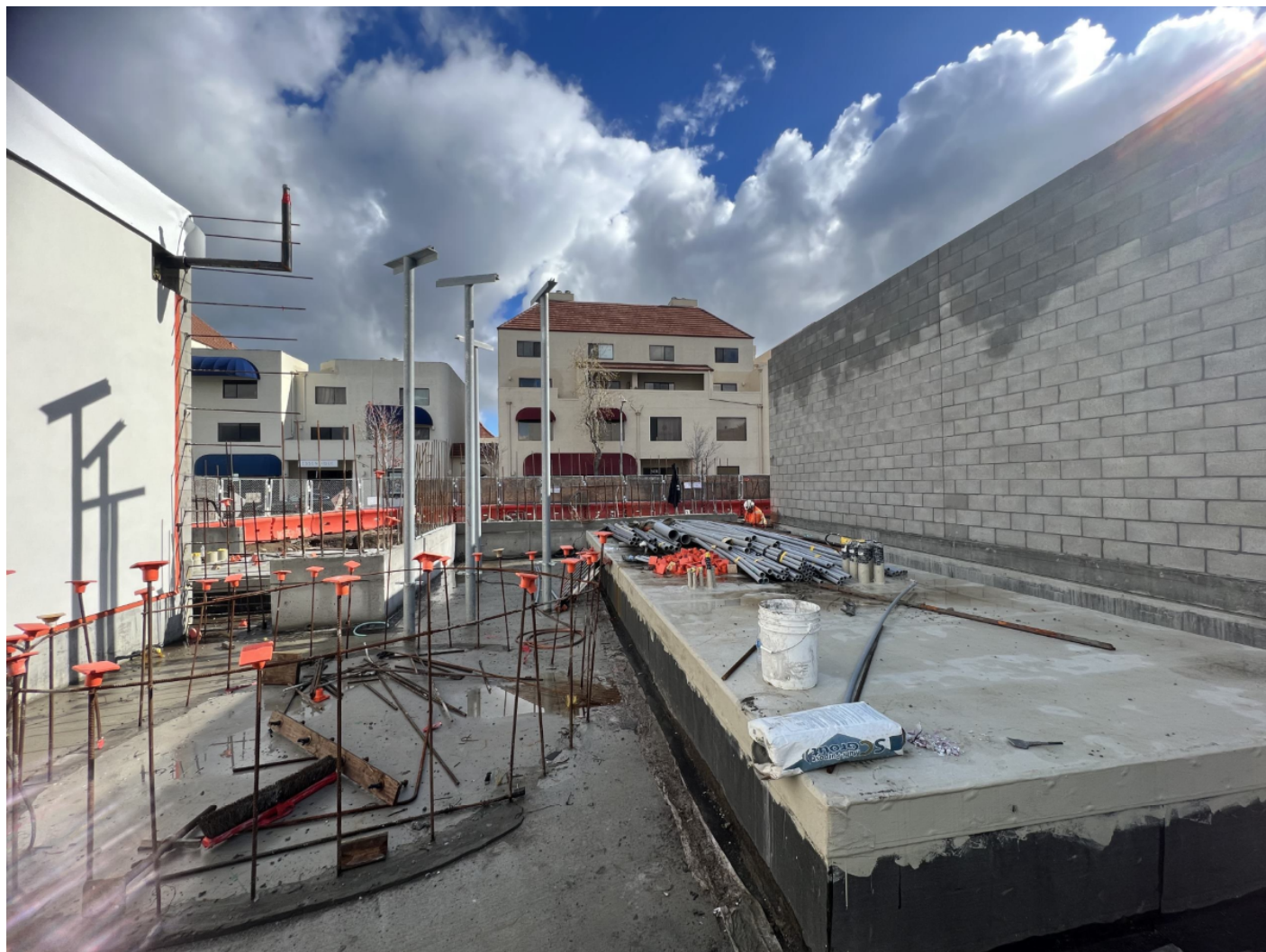
View from Utility Yard of Generator Pad and Plaster Mock-Up.
