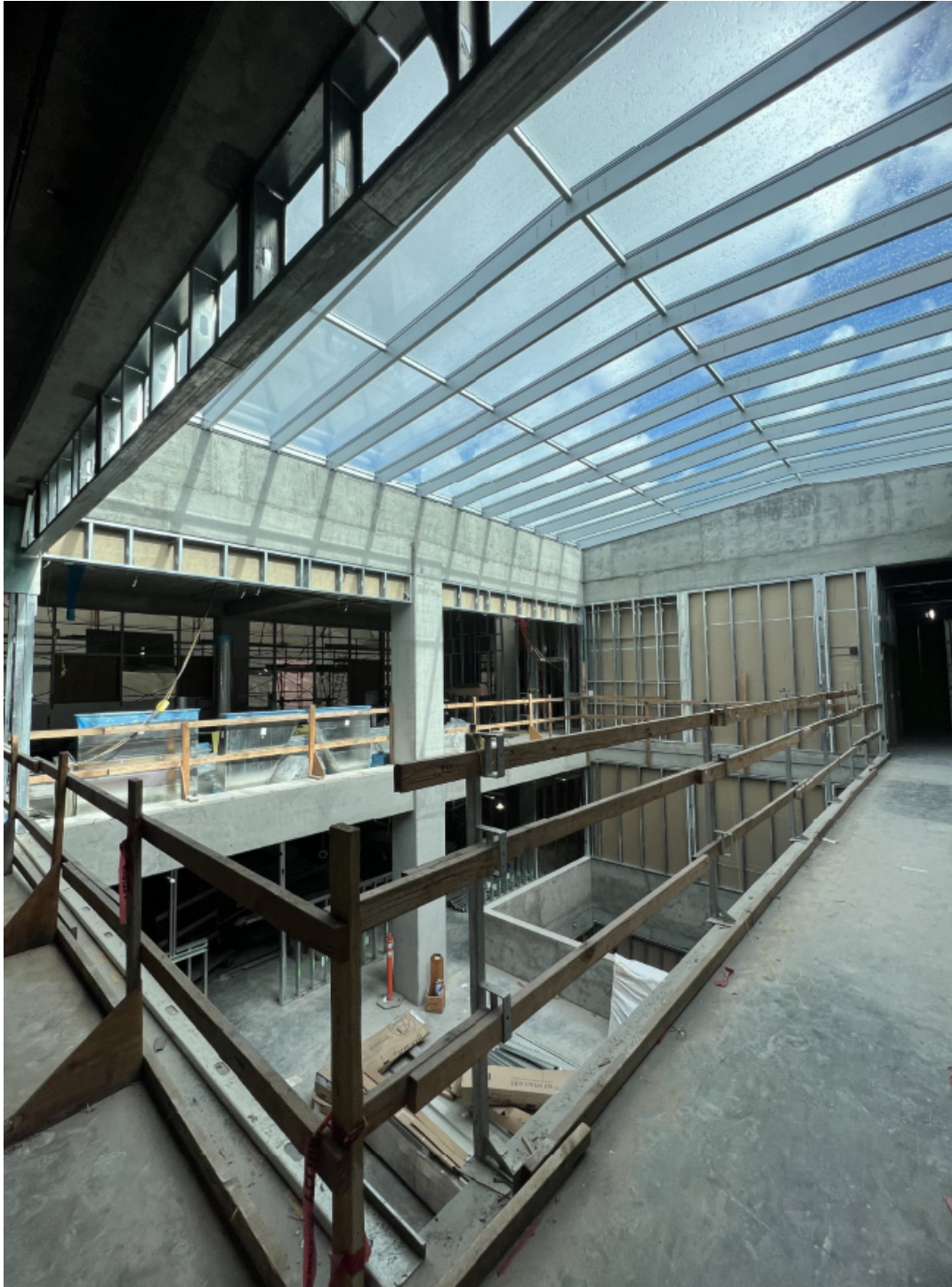
View of skylight from level 3.
