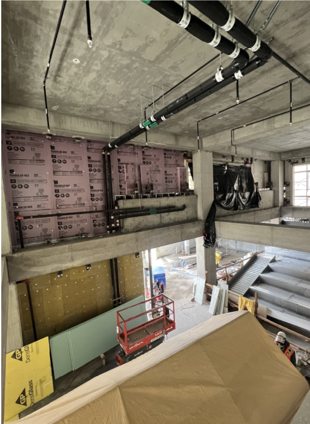
View of lobby from level 2.
