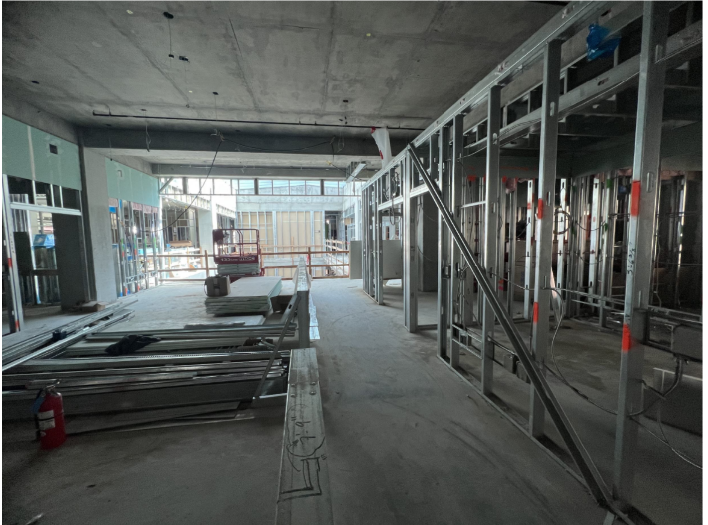
View of open office level 3.
