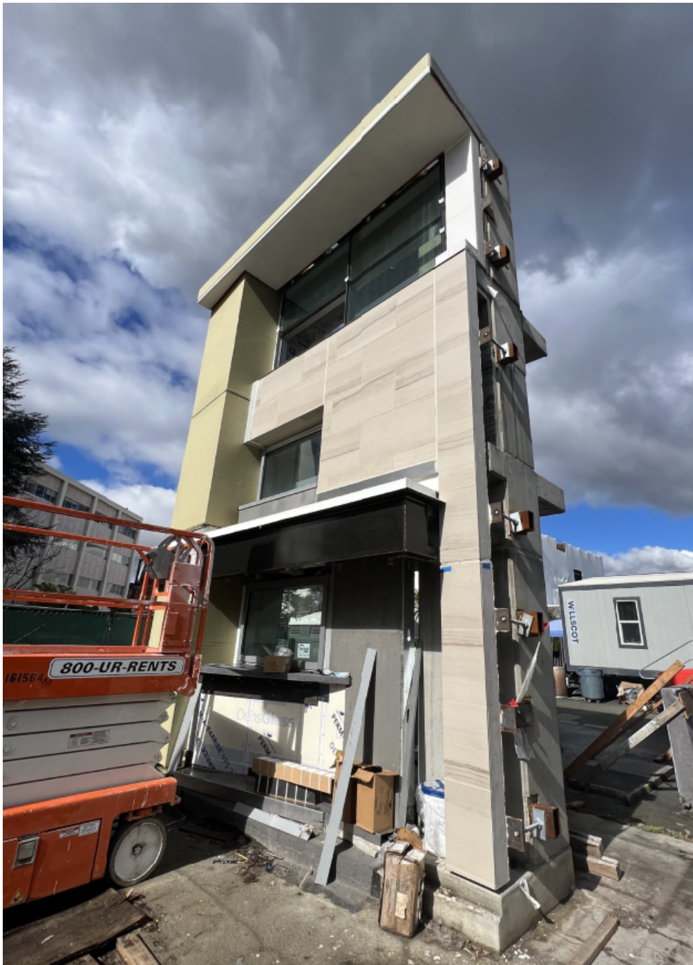
View of building mock-Up.
